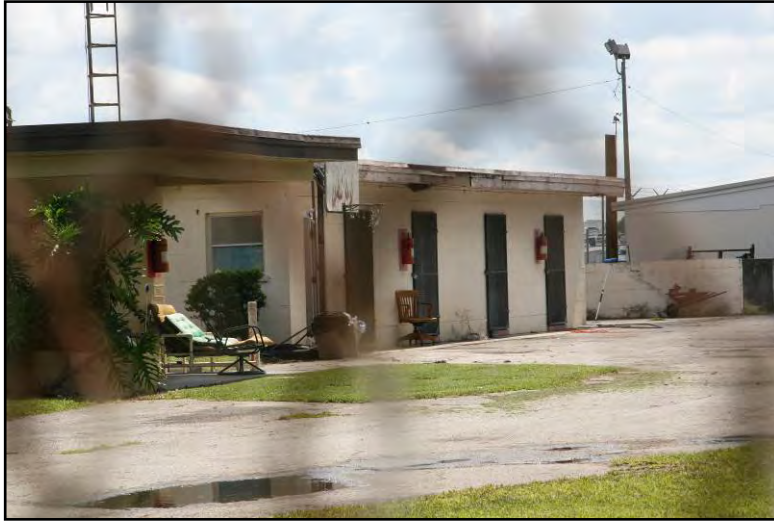
Figure 29. View of Resource Group 8PO07699, facing east.
