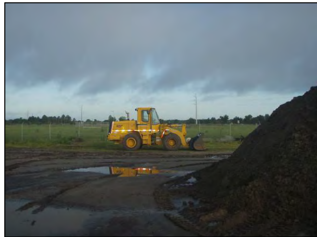
Figure 17. View of proposed Pond 4 showing ongoing construction activities, facing west.
