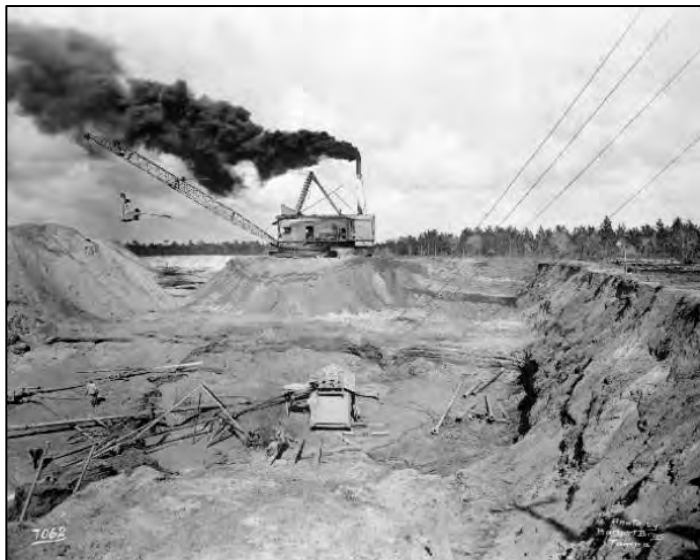
Figure 6. Dragline in use at Southern Phosphate Company Mine. Florida Memory #GE2409.
