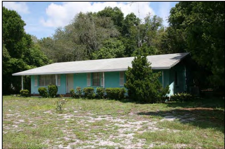
Figure 21. Resource 8PO07694, facing northwest.
