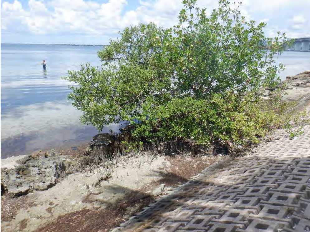
Photo 13: WL-2 facing northeast
