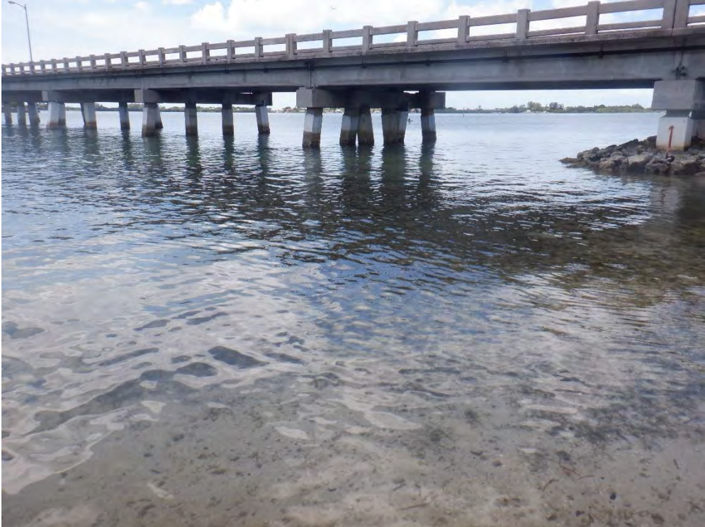
Photo 9: Existing SB bridge from water facing north
