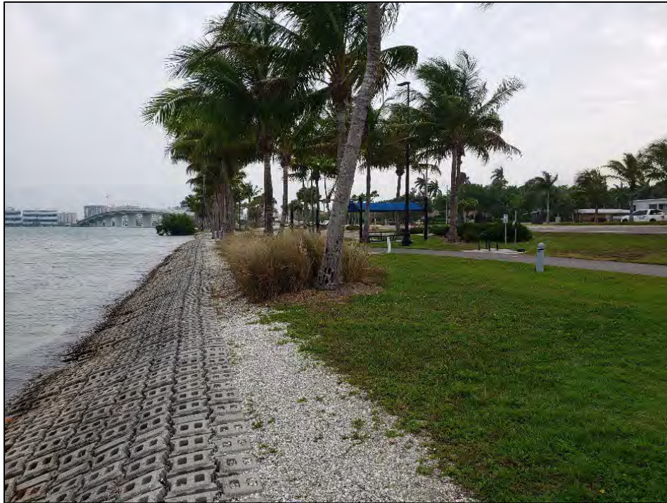
Photo 2-1. Looking northeast towards the Ringling Bridge Causeway Park.
