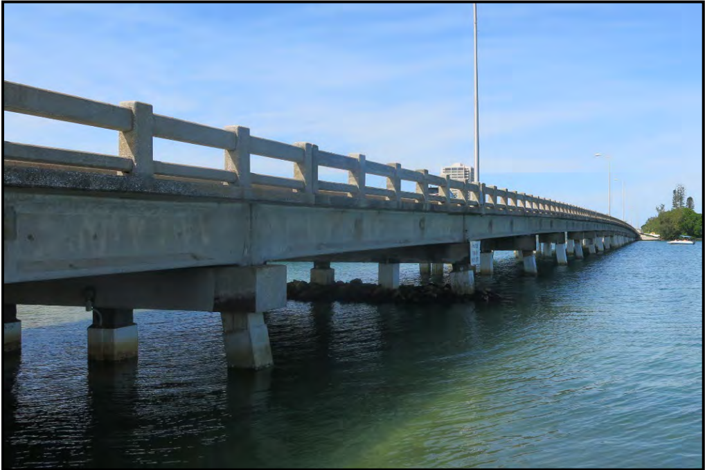
Photo 5-3 SR 789 Southbound over Coon Key Waterway (Bridge No. 170951/8SO06907), looking southwest.
