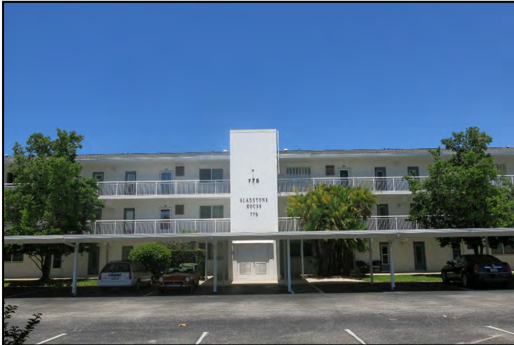
Photo 5-4. 775 John Ringling Boulevard/Gladstone House (8SO12048), looking northwest.
