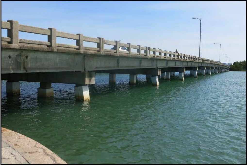
Photo 5-2. SR 789 Northbound over Coon Key Waterway (Bridge No. 170022/8SO06906), looking northeast.
