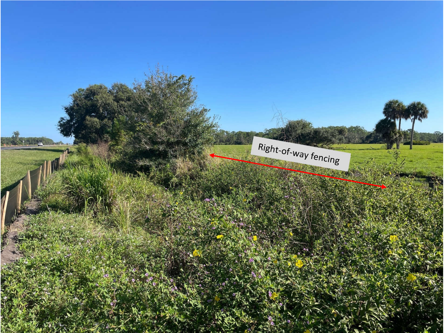
View from top of headwall on the east side of US 27 facing northeast.
