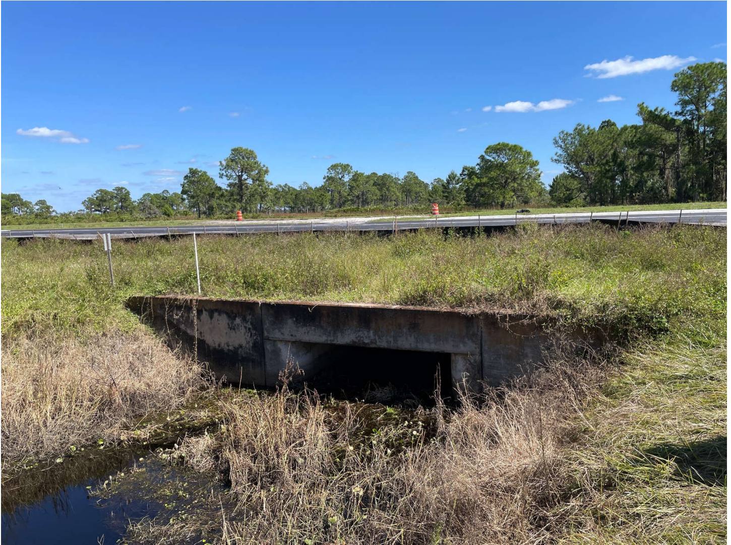
Existing box culvert on the west side of US 27 facing east.
