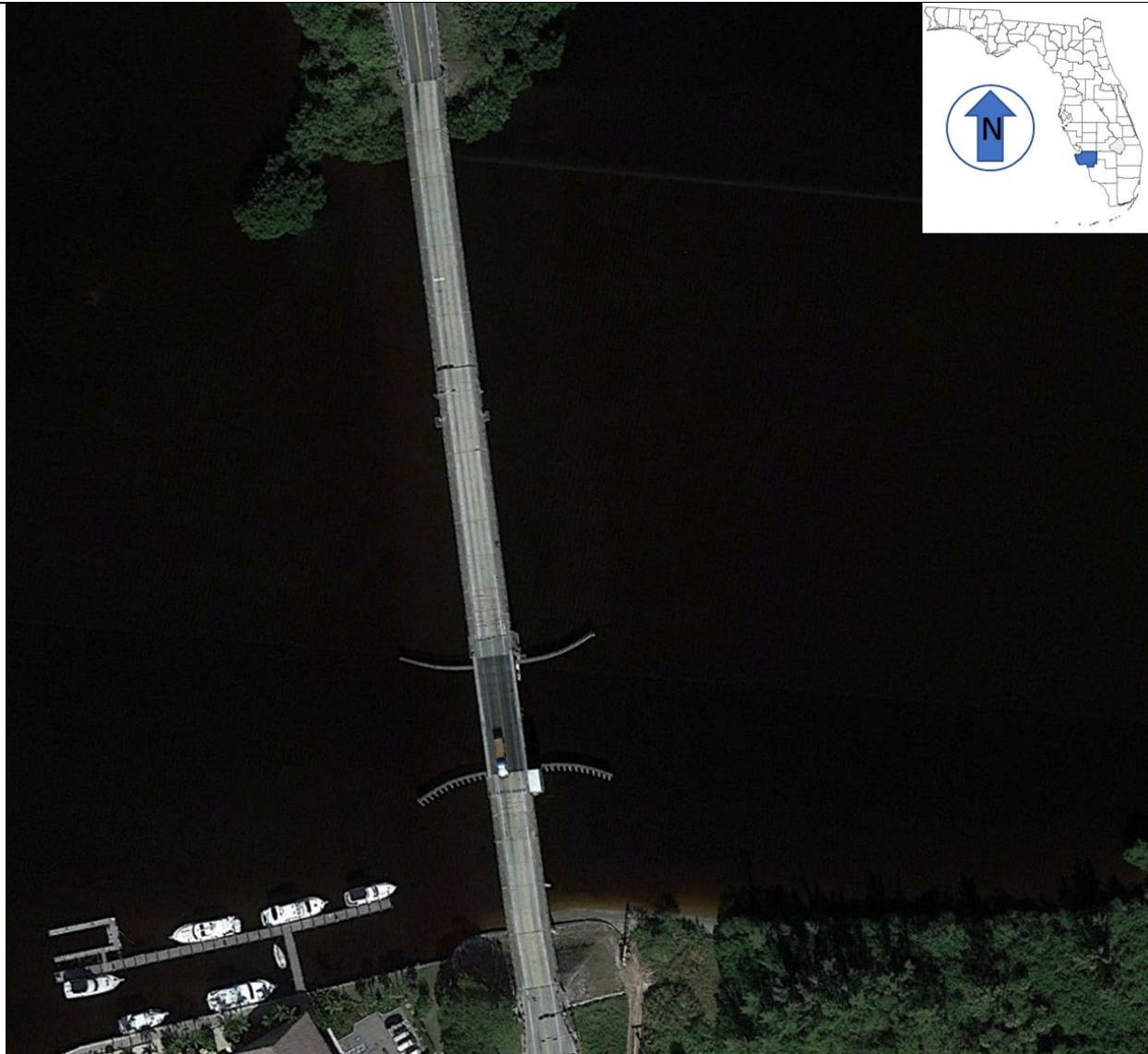
Figure 2.2 Zoomed View of Existing Bridge
