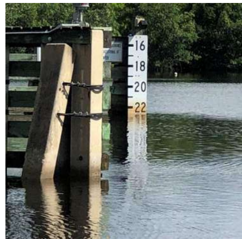
Figure 2.2.2 Vertical Clearance Post
