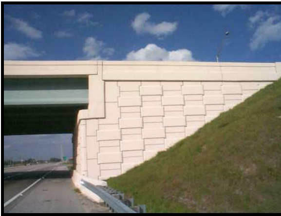
Figure 7.0.1 Wrap-Around MSE Wall
