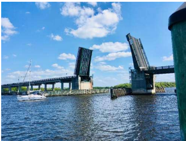
Figure 2.2.1 Bridge Elevation – Bascule Span Open
