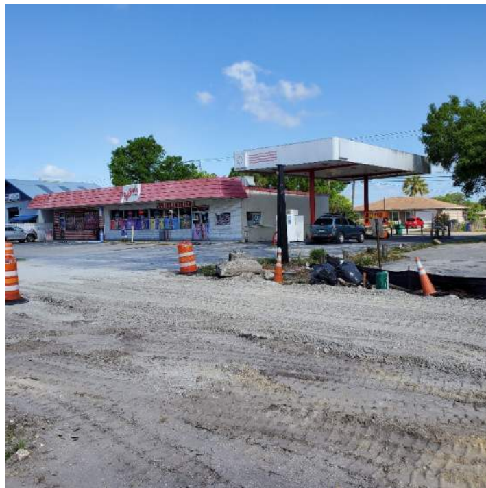
Site 11 – Redbone Spirits/Former Circle K gas station SR 80 looking northwest
