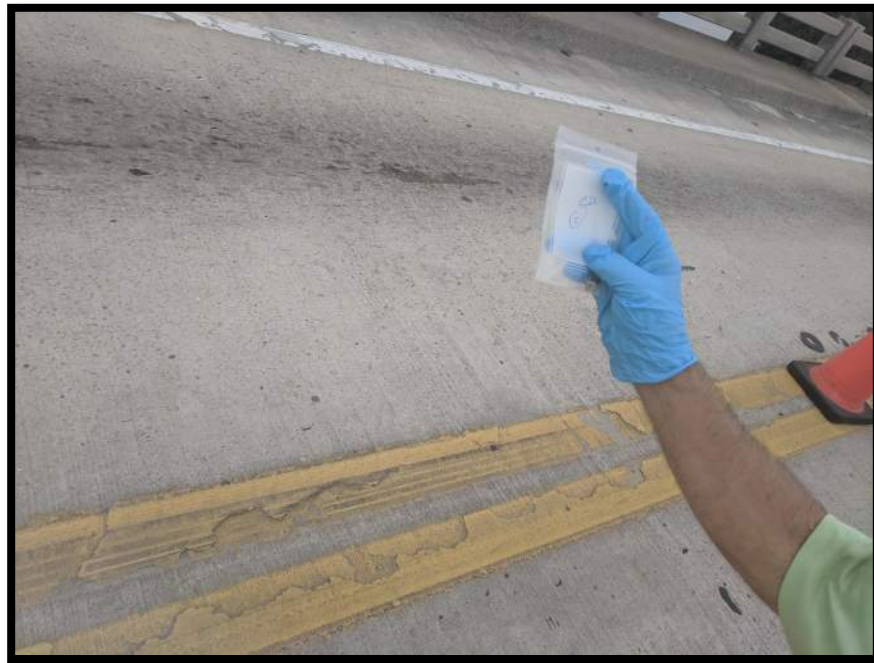
Photograph 4 View of Asbestos Homogeneous Area 1 – Concrete – Roadway Deck (Sample Location 2).
