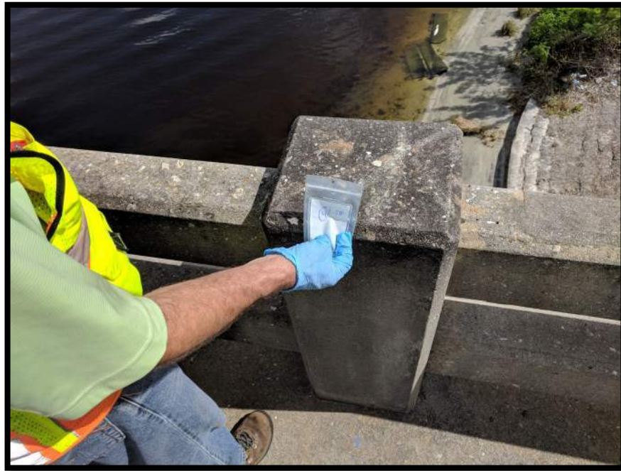
Photograph 5 View of Asbestos Homogeneous Area 2 – Concrete – Barriers and Sidewalks (Sample Location 4).
