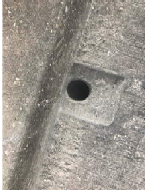
Photo No. 10 - View of Steel Scuppers- NOT Suspected to Contain Asbestos
