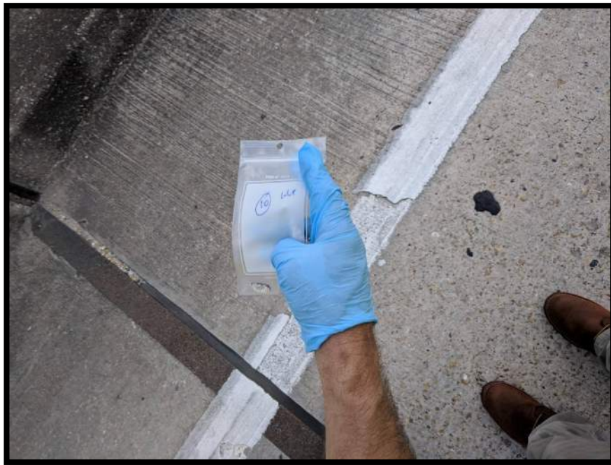
Photograph 11 View of Asbestos Homogeneous Area 4 – White Lane Paint – Roadway Deck (Sample Location 10).
