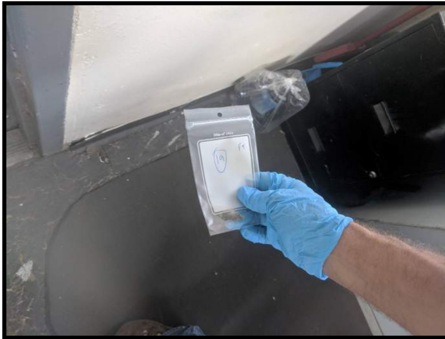
Photograph 20 View of Asbestos Homogeneous Area 7 – 12”x12” Floor Tile and Adhesive Mastic (Bottom Layer) – Tender House (Sample Location 19).
