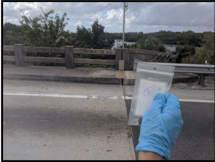
Photograph 37 View of Asbestos Homogeneous Area 12 – Asphalt Roadway – Bridge Approaches (Sample Location 36).
