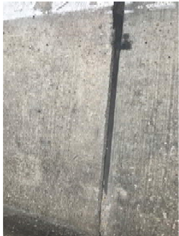
Photo No. 8 - Non-Asbestos-Containing Expansion Joint
