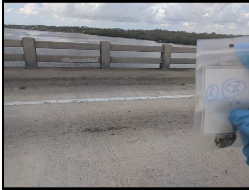
Photograph 7 View of Asbestos Homogeneous Area 2 – Concrete – Barriers and Sidewalks (Sample Location 6).
