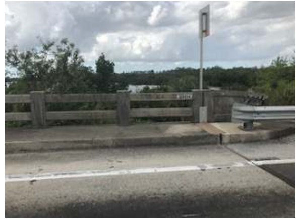
Photo No. 6 - Non-Asbestos-Containing Concrete Barriers
