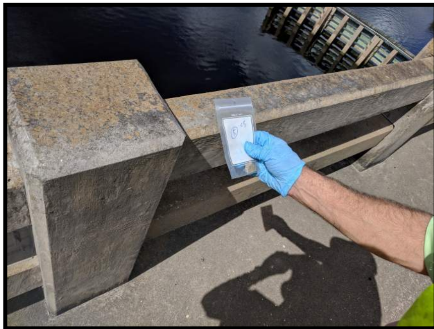
Photograph 6 View of Asbestos Homogeneous Area 2 – Concrete – Barriers and Sidewalks (Sample Location 5).
