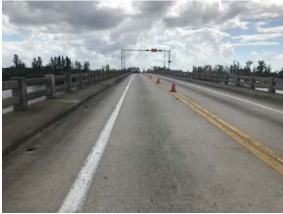
Photo No. 9 - Non-Asbestos-Containing Yellow and White Lane Paint
