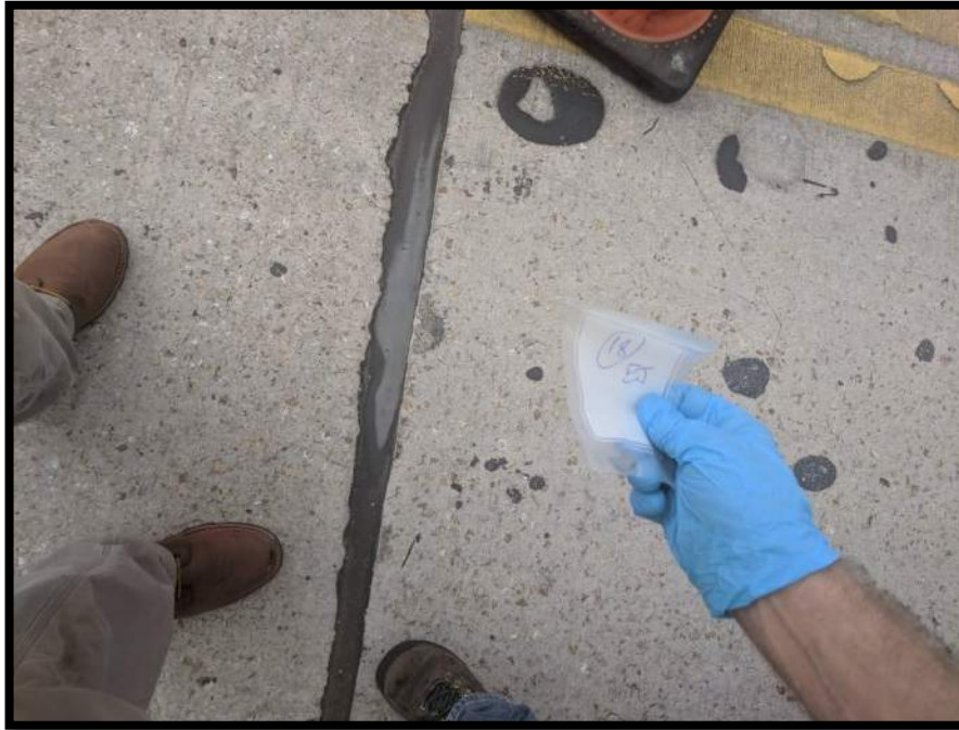
Photograph 19 View of Asbestos Homogeneous Area 6 – Expansion Joints – Roadway (Sample Location 18).
