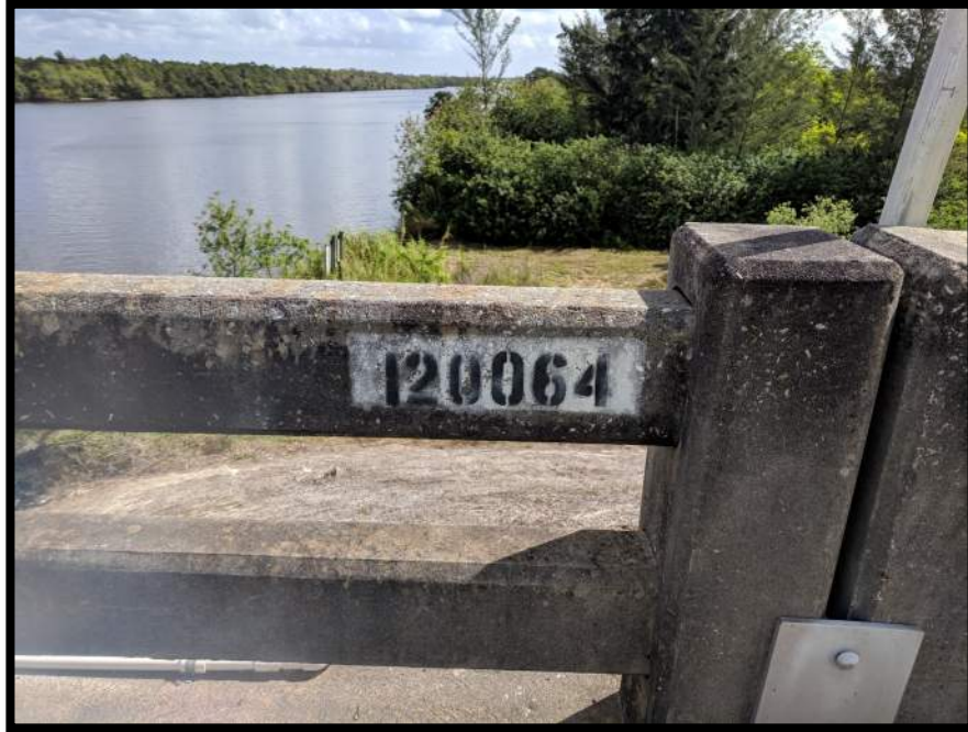
Photograph 1 View of Bridge No. 120064.
