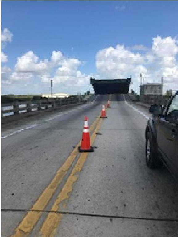
Photo No. 1- Non-Asbestos-Containing Concrete Barriers, Concrete Roadway and Yellow Lane Paint
