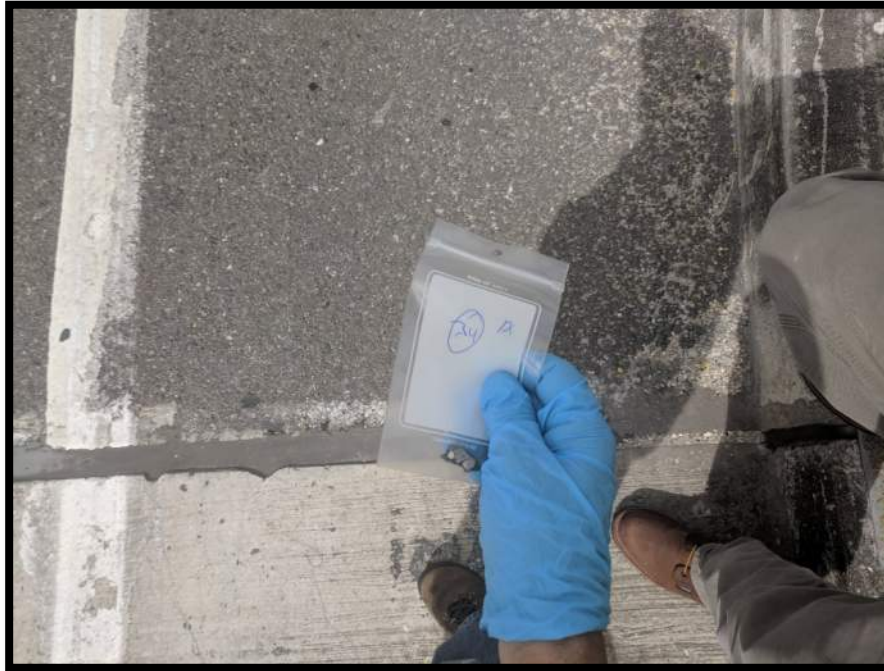
Photograph 35 View of Asbestos Homogeneous Area 12 – Asphalt Roadway – Bridge Approaches (Sample Location 34).
