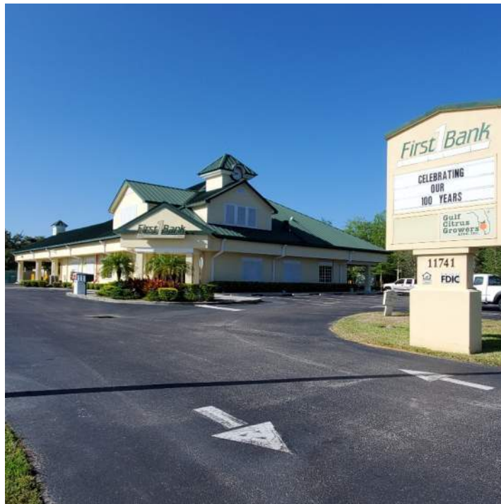
Site 3 – First Bank South side of SR 80 looking south
