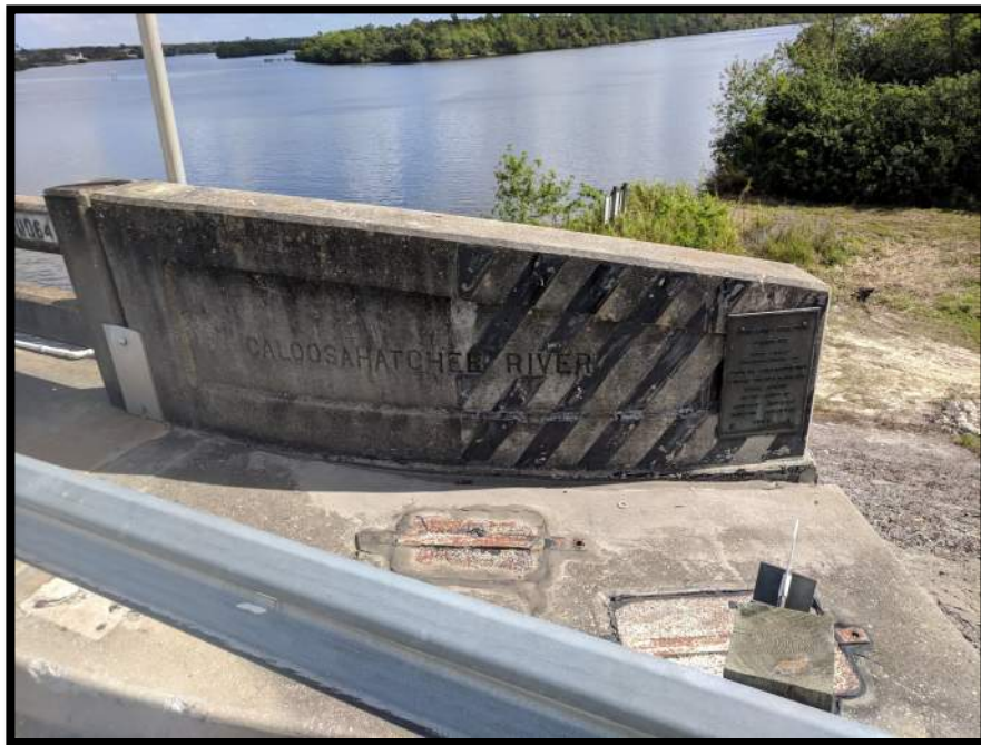
Photograph 2 View of Bridge No. 120064.
