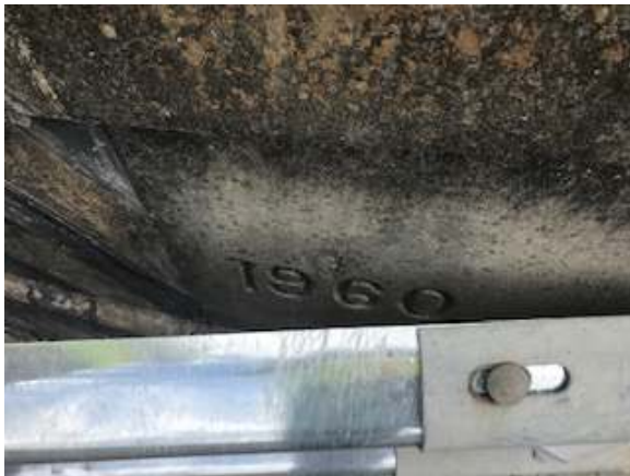
Photo No. 11- Non-Asbestos-Containing Concrete Barrier Showing Year of Construction (1960)
