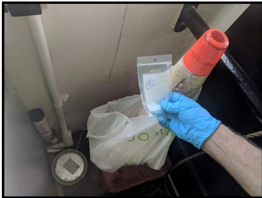
Photograph 34 View of Asbestos Homogeneous Area 11 – Textured Wall Paint – Tender House (Sample Location 33).
