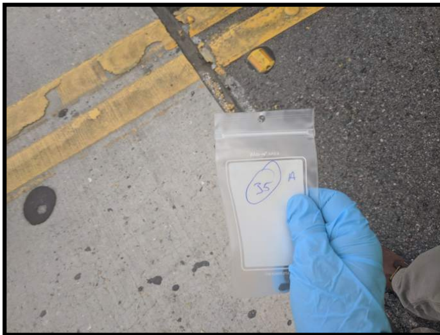
Photograph 36 View of Asbestos Homogeneous Area 12 – Asphalt Roadway – Bridge Approaches (Sample Location 35).
