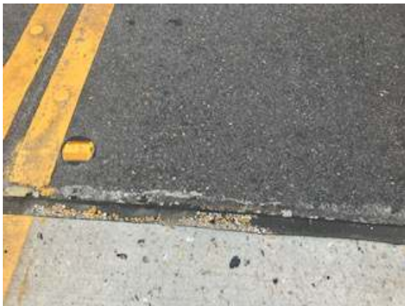
Photo No. 7 - Non-Asbestos-Containing Reflector Mastic
