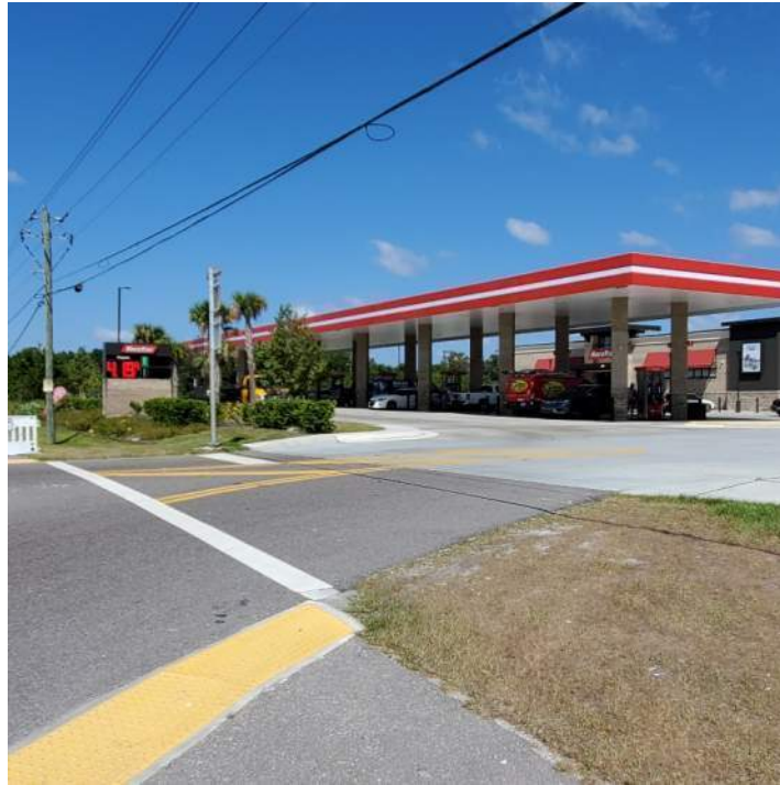
Site 8 – RaceTrac North of SR 80 looking northwest
