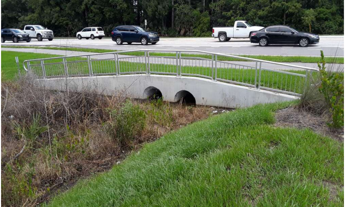
Existing Cross Drain CD-04 - North side of SR 80, Looking South
