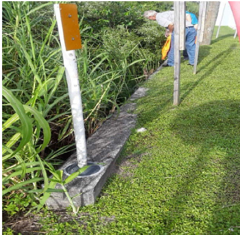
Existing Cross Drain CD-02 – West side of SR 31, Looking West, Downstream Side
