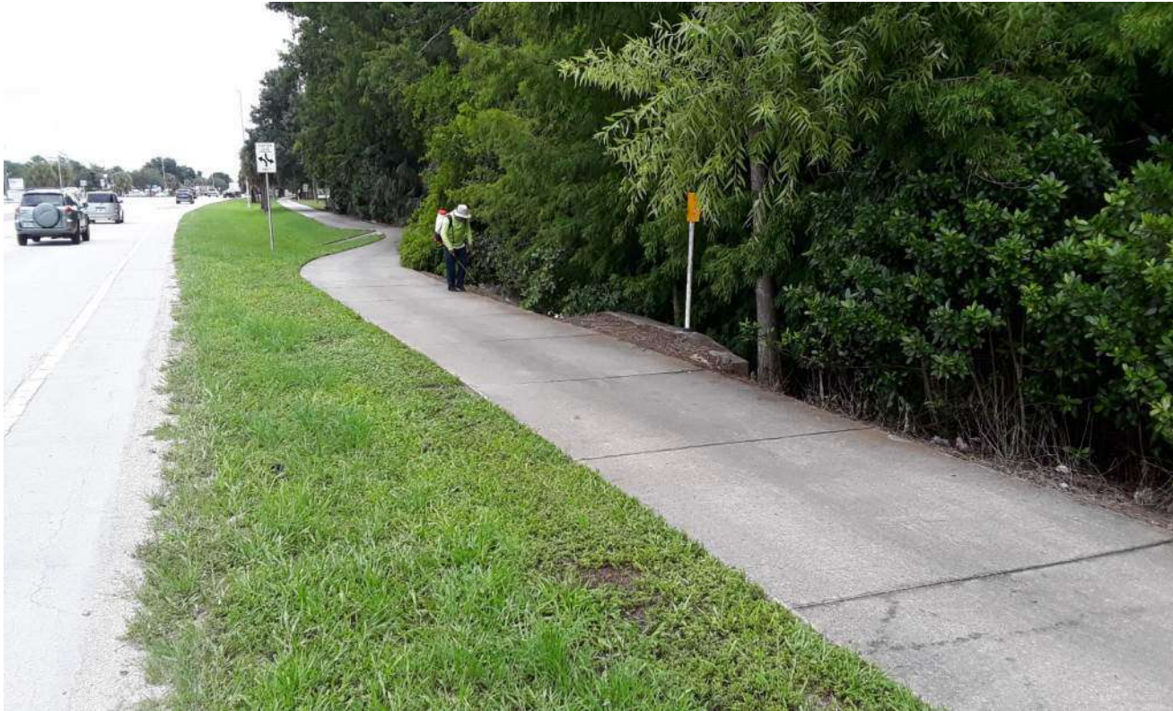
Existing Cross Drain CD-04 – South side of SR 80, Looking East at CD-04 Headwall
