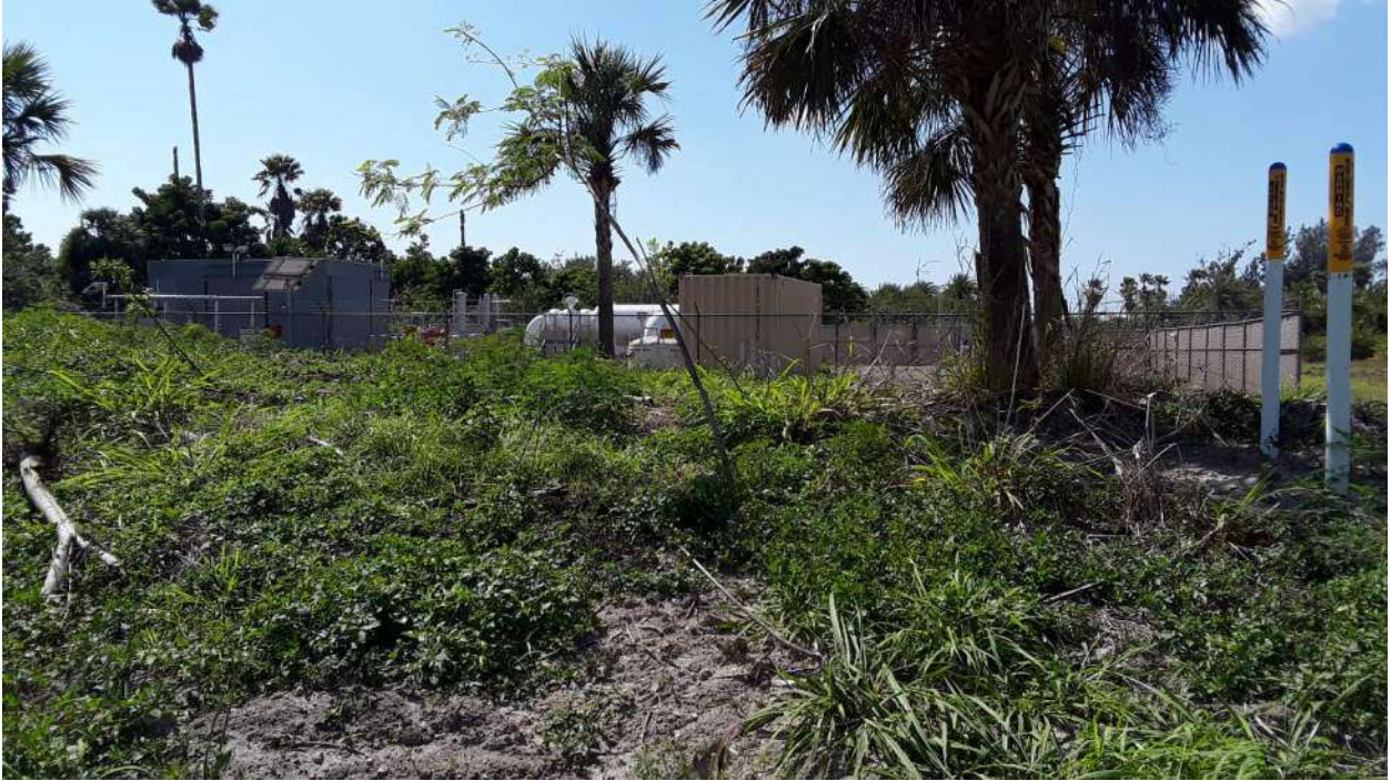
Looking West at Gas Line Sub-Station
