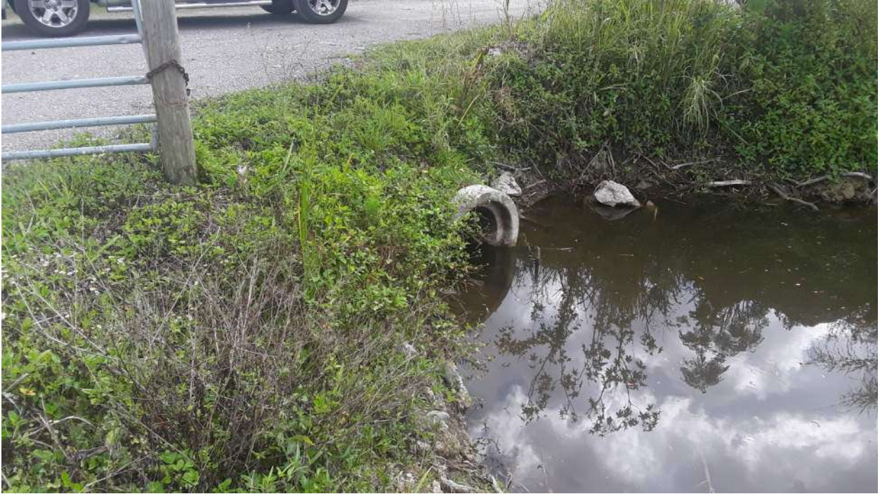
Looking West at Upstream end of Existing 24" cross drain
