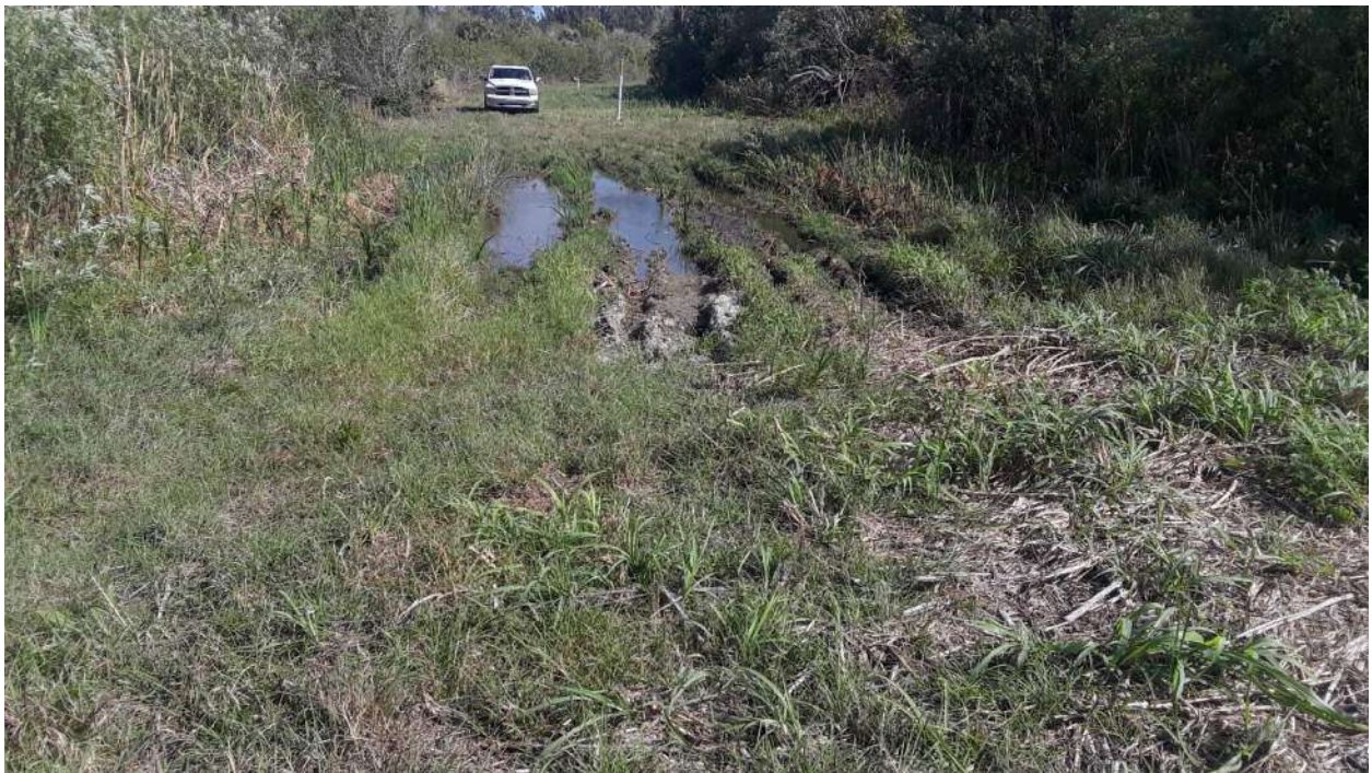
Looking North at natural Drainage swale outfall in Gas line trail
