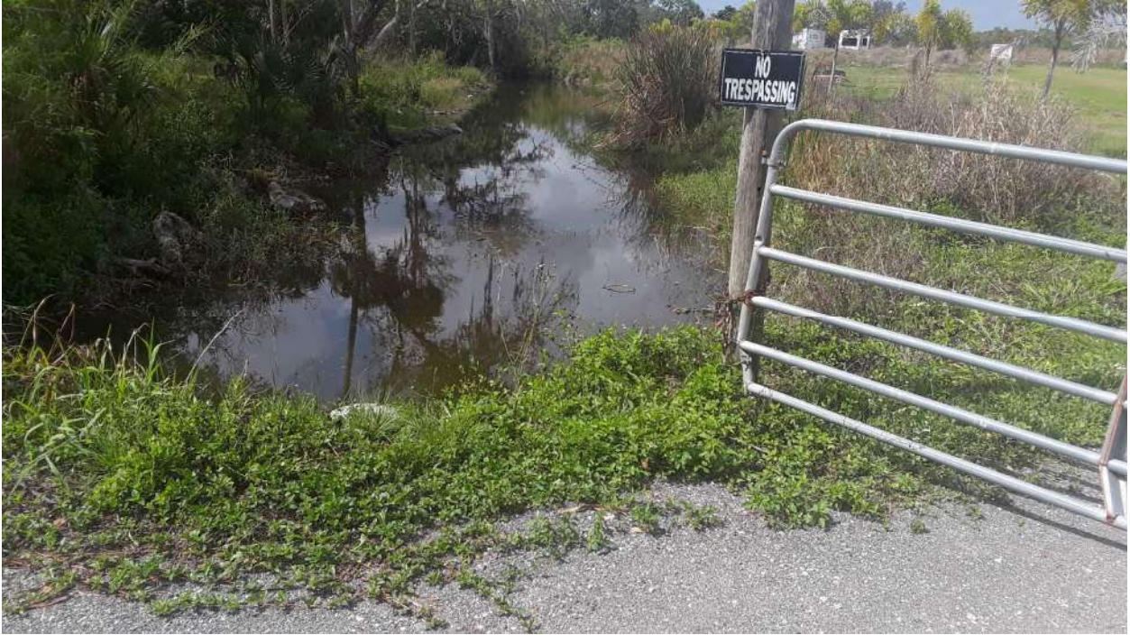
Looking West at Downstream side of 24" cross drain
