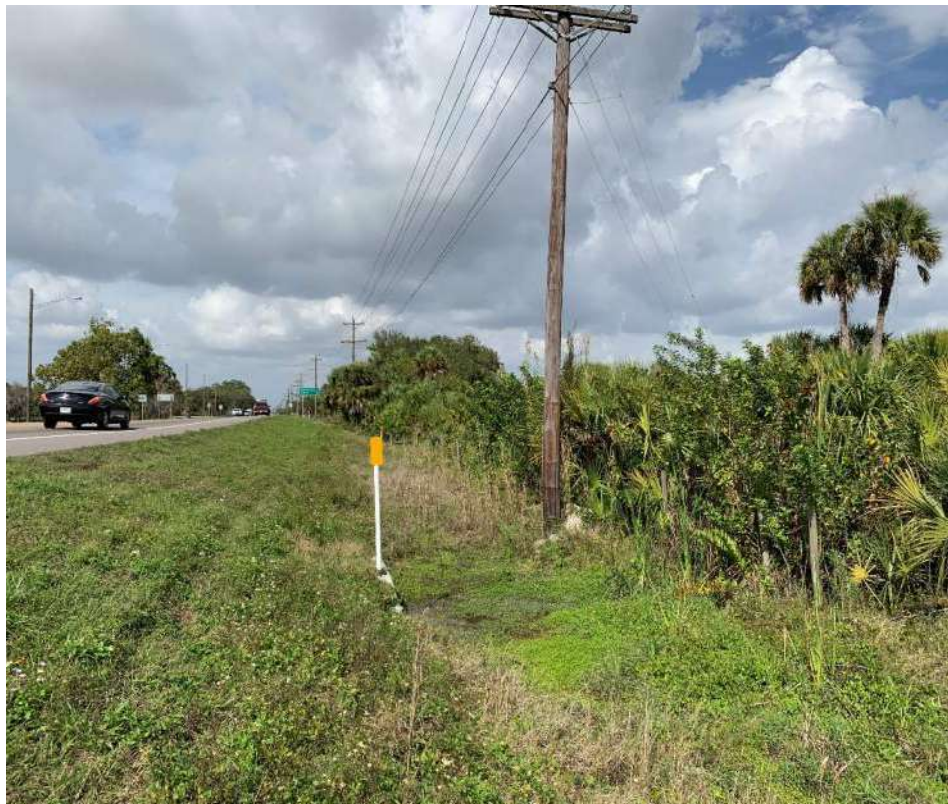
Existing Cross Drain CD-03 – east side of SR 31, Looking North, Downstream Side
