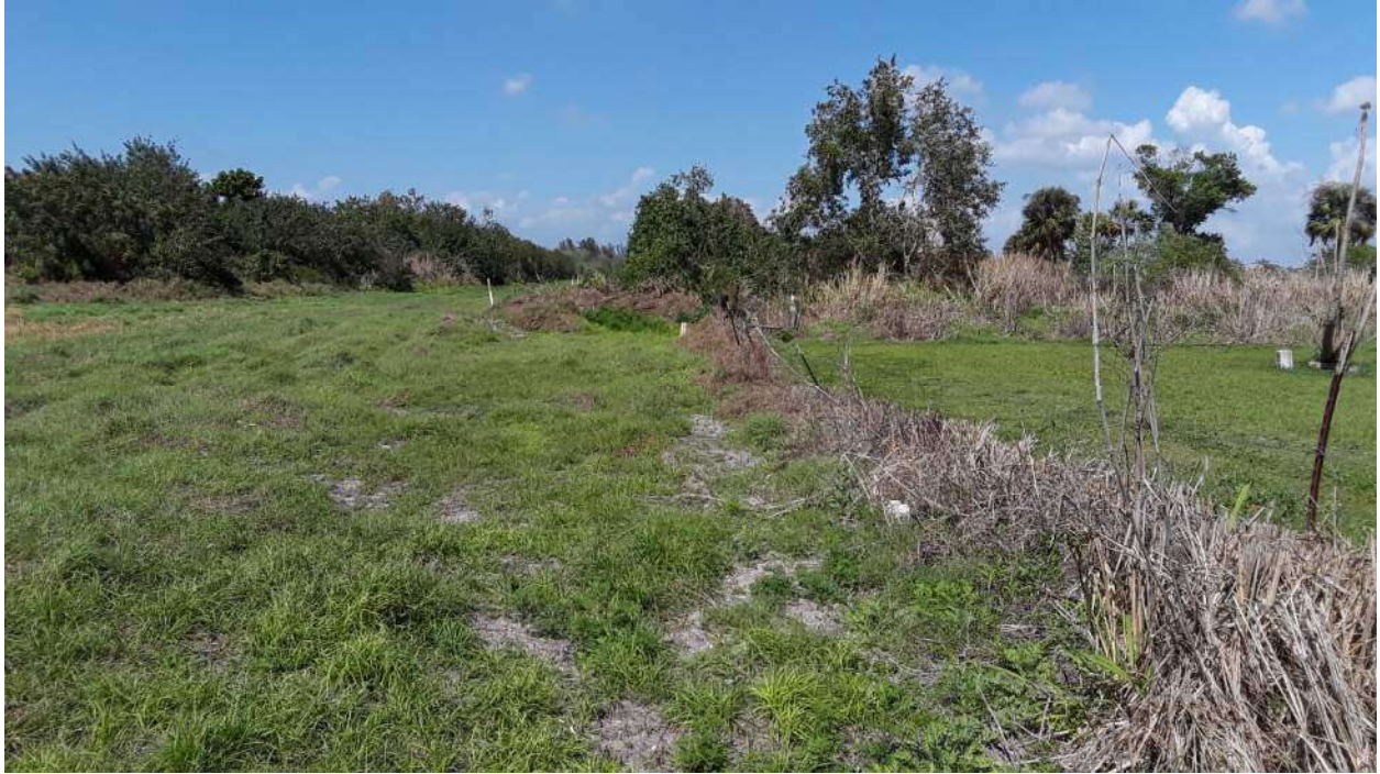
Looking North along natural drainage swale at the east side of Gas Line Sub-Station
