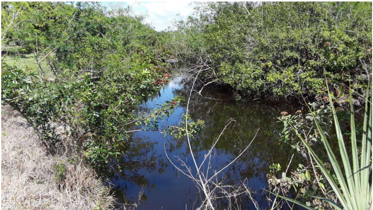
Looking West at Drainage Outfall creek
