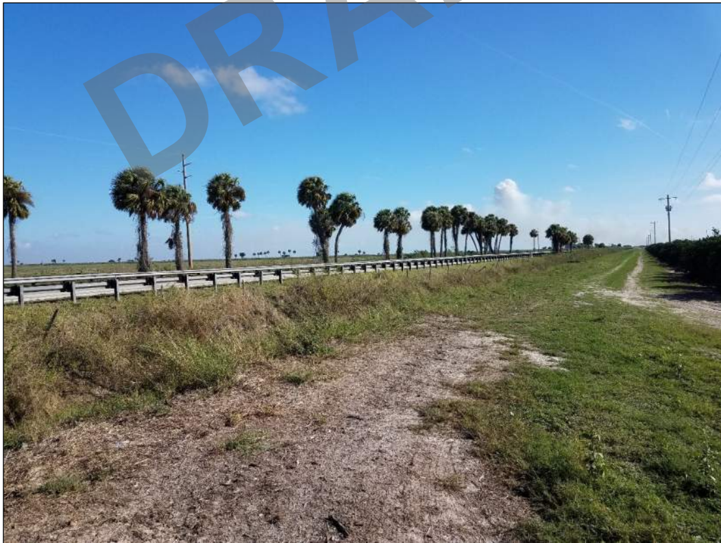
Survey Station 7, facing east
