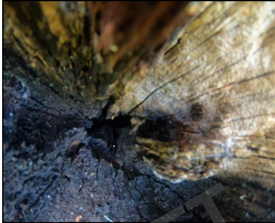
Photo 7. Photograph of a live oak cavity that was visually inspected using the extension pole – Tree 4 (see Attachment C ).
