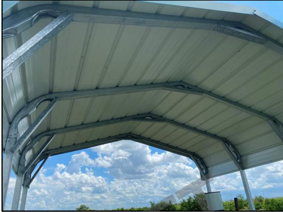
Photo 31. Photograph of a pavilion structure within the project study area.
