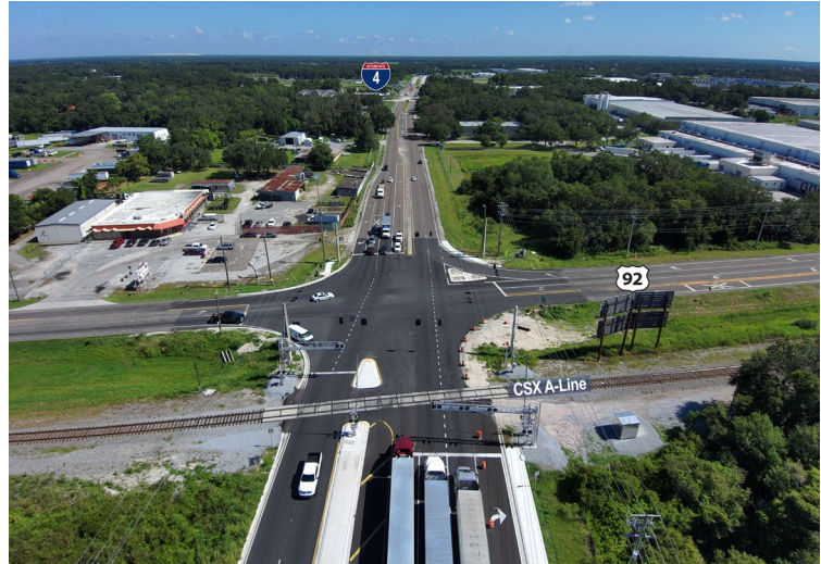
County Line Road at-grade crossing with CSX A-Line (Looking North)
