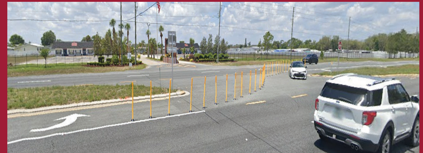
An example of temporary delineators that may be installed in 2024.
