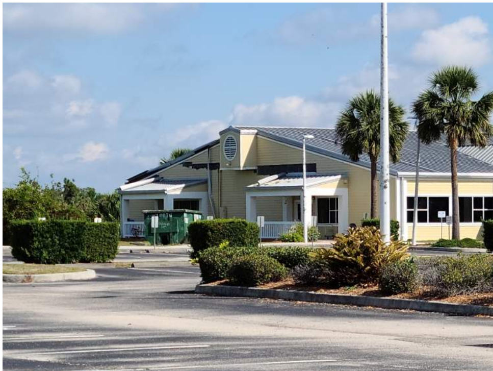
Site 5 – Charlotte County Pest-Management Harborview road near eastern project boundary, looking northeast
