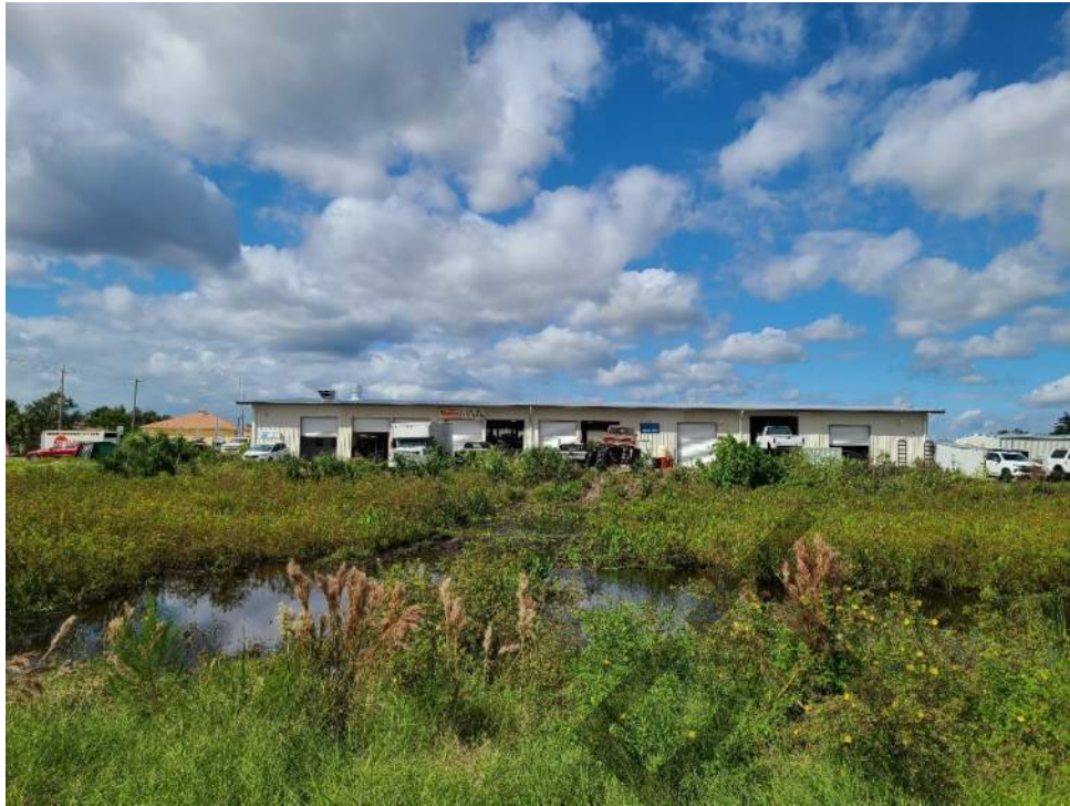
Site 8 – Clune’s Autobody Inc/Dr. D’s Auto & Marine Repair North end of Harborview Road and Melbourne Street intersection
