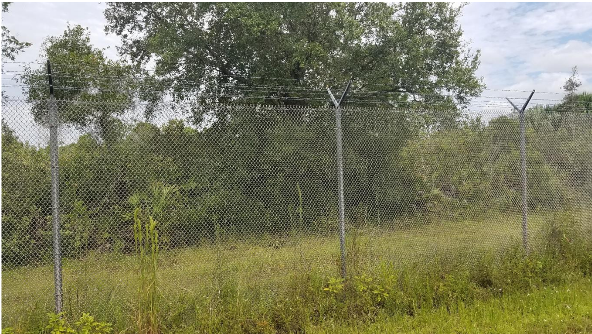
Pond 5C: southern boundary looking north
