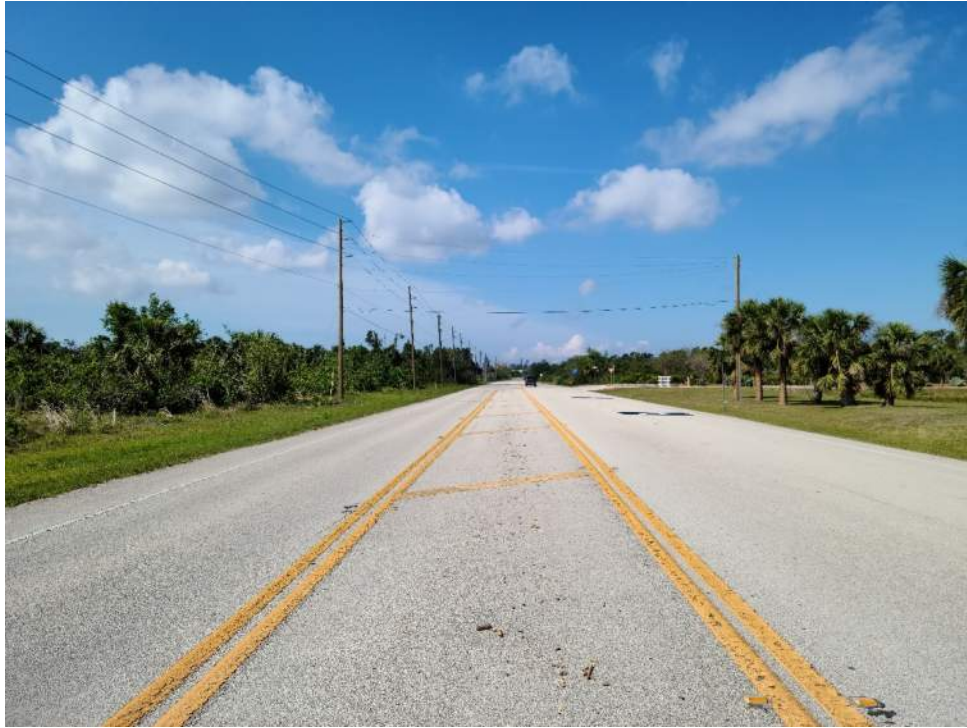
Eastern project boundary Harborview Road facing west
