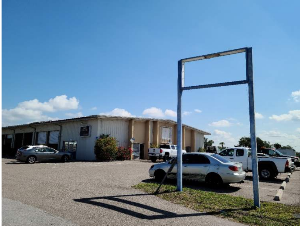
Site 8 – Clune’s Auto Body Inc/Former Dr. D’s Auto & Marine Repair Harborview Road looking northeast
