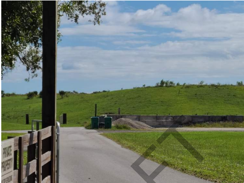
Site 6 – Former Raulerson Yard Trash Compost Site Rowland Drive looking east
