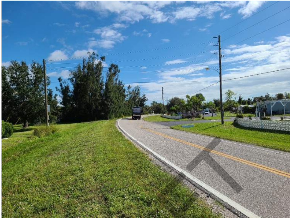
Near the center of the project Harborview Road looking northeast
