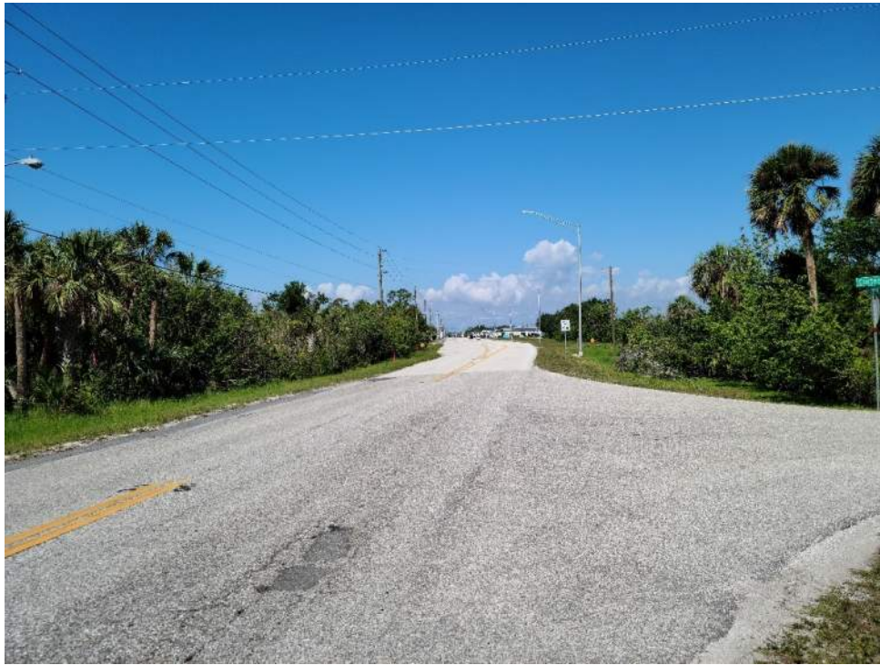
Harborview Road and Cortez Drive Near western project boundary looking west
