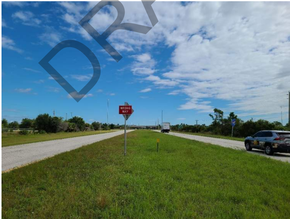
Eastern project boundary Harborview Road looking northeast
