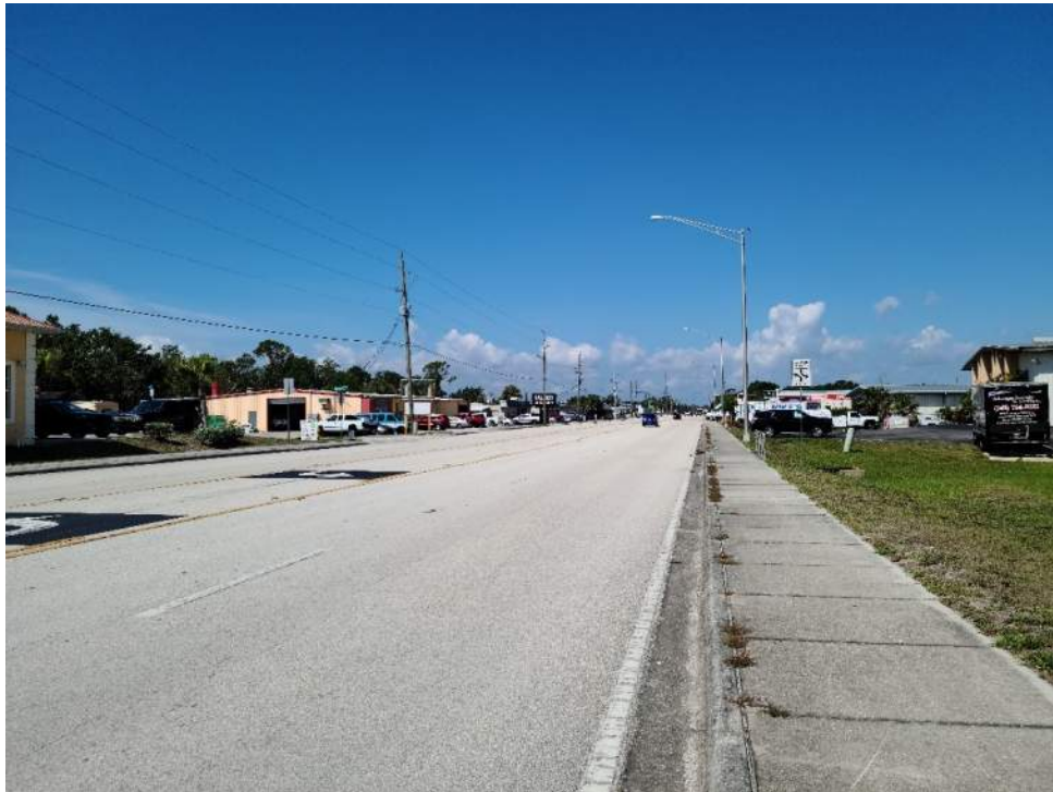
Western project boundary Harborview Road looking east
