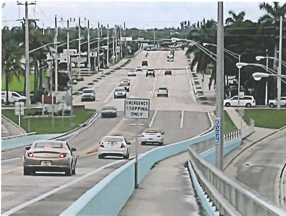
Photo 6. Looking north along sidewalk (Estero-Bonita “trail”) on the Matanzas Pass Bridge toward San Carlos Island.
