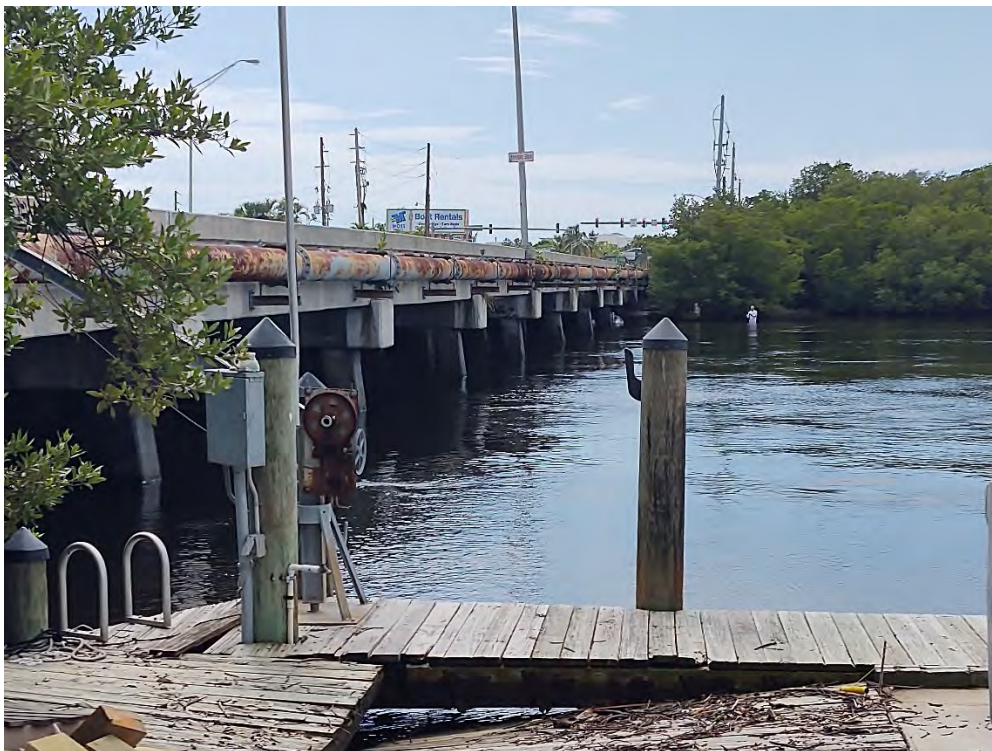
Photo 2. Looking south along the west side of the Hurricane Bay Bridge at Great Calusa Blueway Paddling Trail crossing location under bridge.
