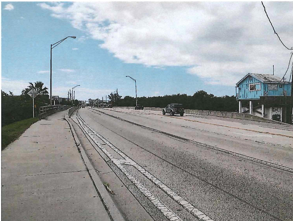
Photo 8. Looking south along sidewalk (Estero-Bonita “trail”) approaching the north side of the Hurricane Bay Bridge
