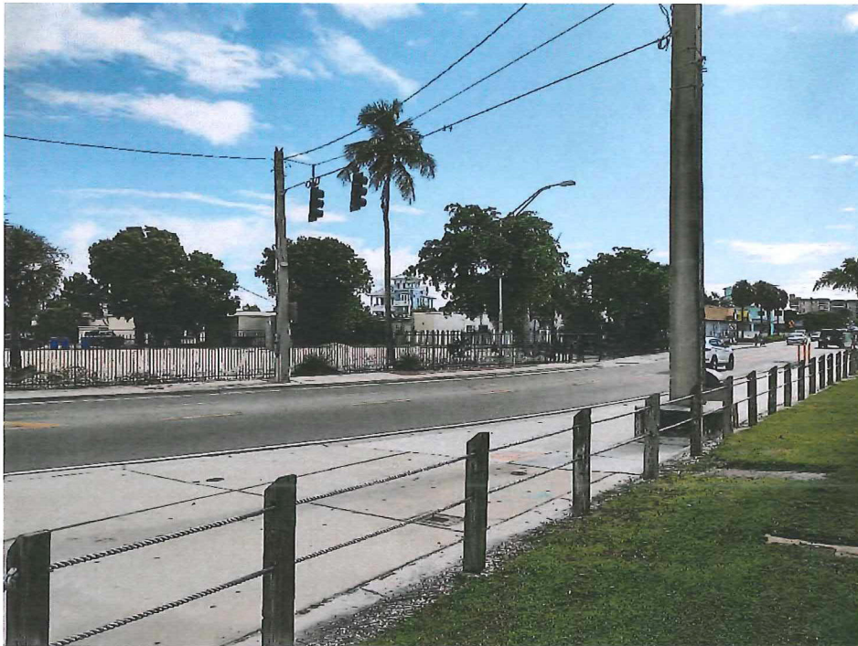
Photo 1. Looking north at sidewalk (Estero-Bonita “trail”) along black vertical fence along north side of SR 865 opposite Crescent Beach Family Park.
