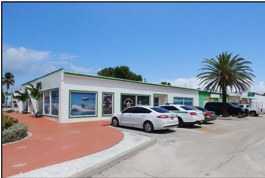
Photo 4. 1133 Estero Boulevard (Bldg 1) (8LL02836), looking north.
