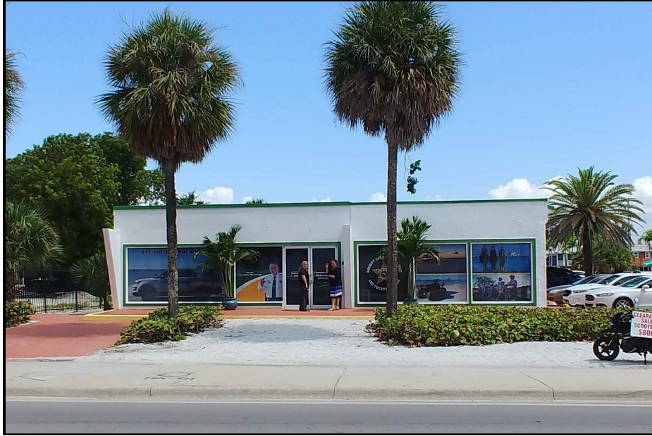
Photo 3. 1133 Estero Boulevard (Bldg 1) (8LL02836), looking northeast.
