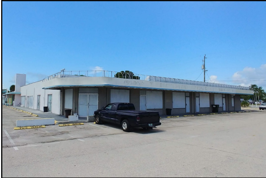
Photo 5. 1133 Estero Boulevard (Bldg 2) (8LL02837), looking southwest.
