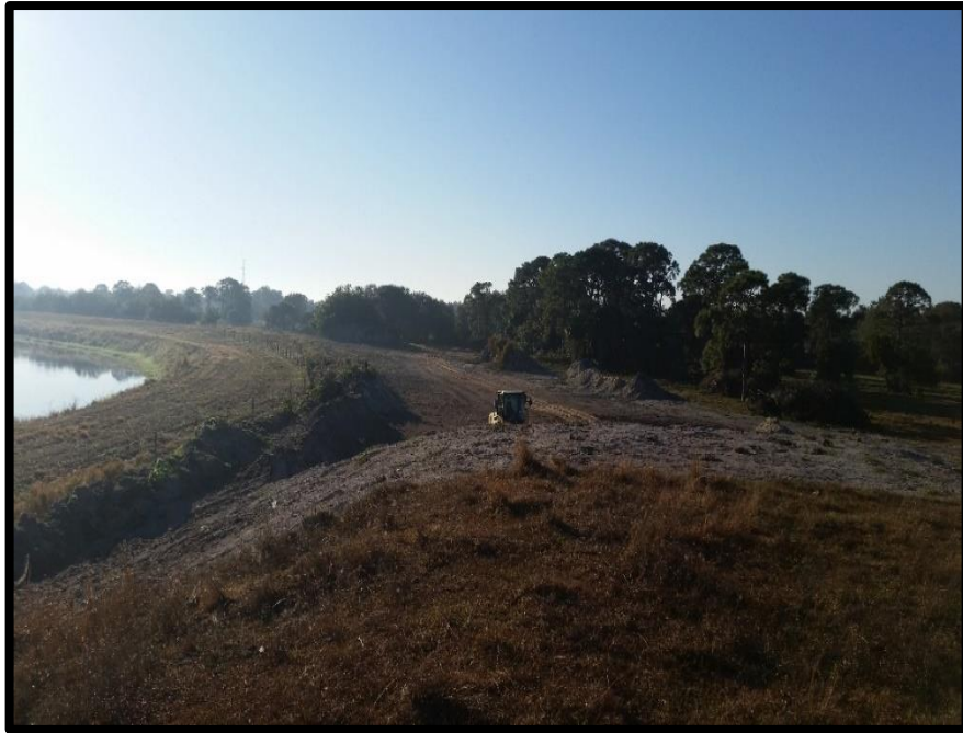
Station 4 – View South
