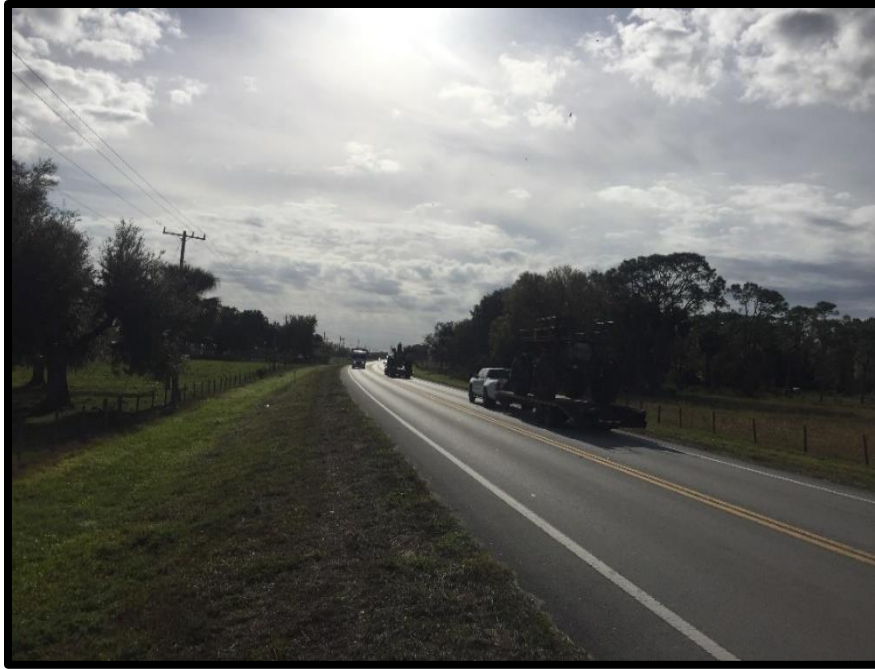
Station 6 – View East
