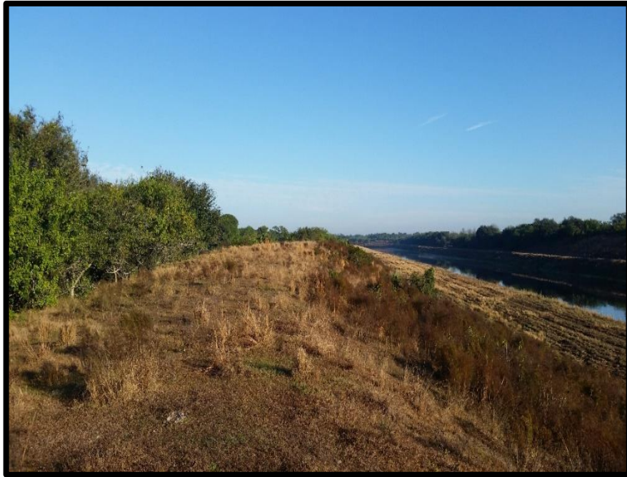
Station 4 – View North
