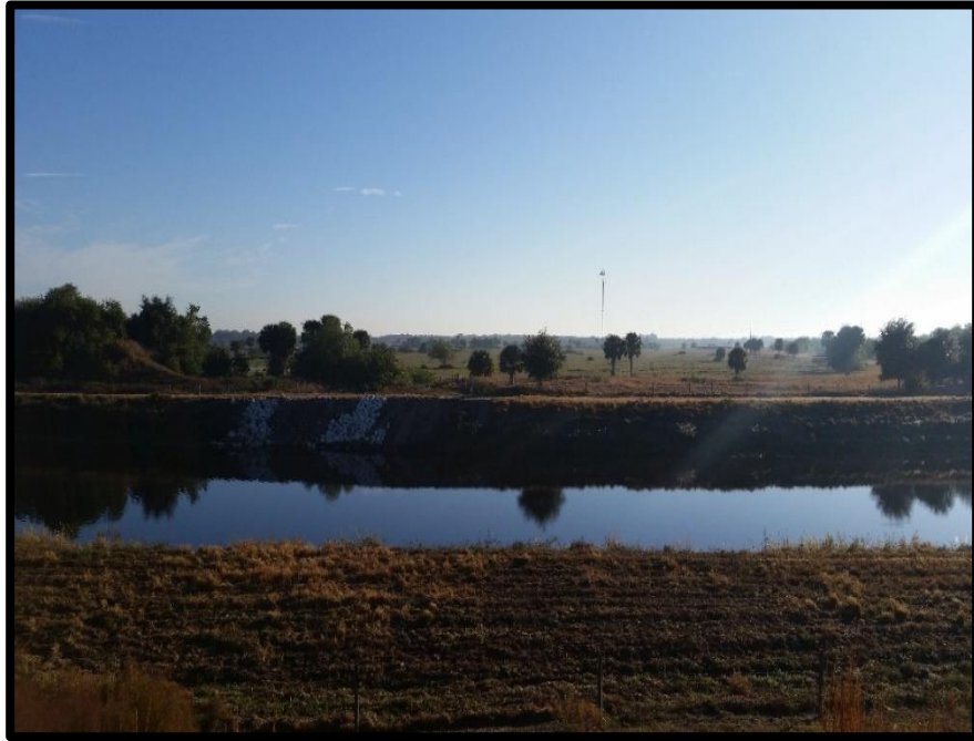
Station 4 – View East
