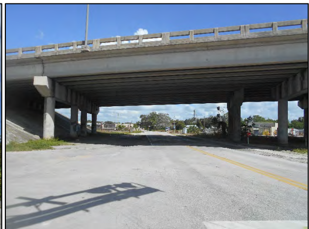
End of Segment 1 at Magnolia Avenue overpass
