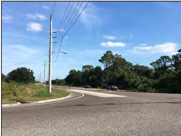
Right-of-way along SR 544/Lucerne Park Road
