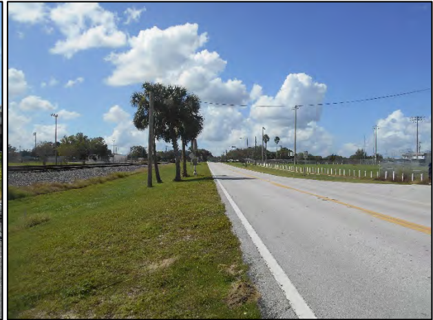
Right-of-way along Stadium Road
