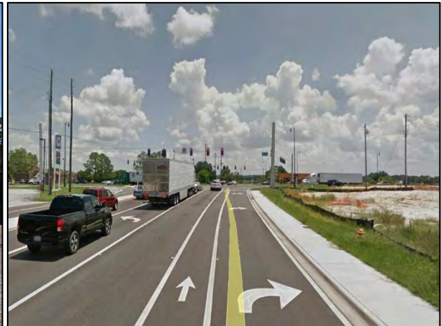
End of Segment 10 at US 27
