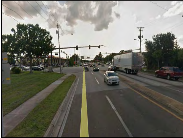
Beginning of Segment 10 at Avenue T NW
