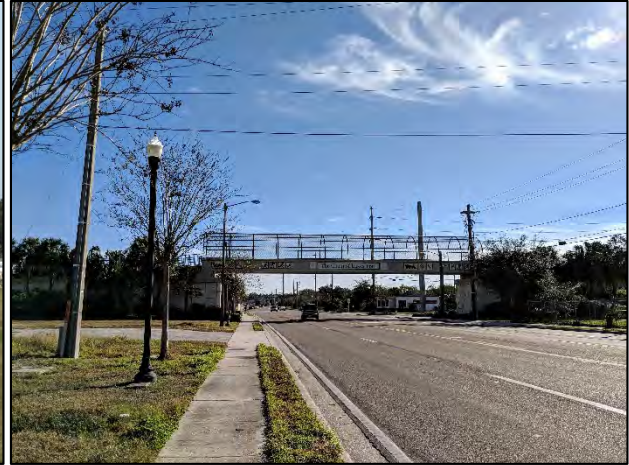
End of Segment 4 at the Chain of Lakes Trail bridge
