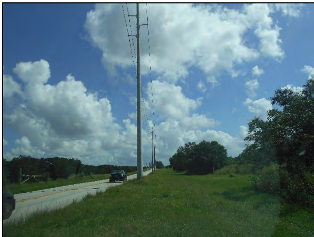
Right-of-way along Old Lake Alfred Road
