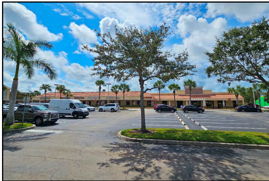
Photo 5.4. 8951 Bonita Beach Road SE (Bldg 1) (8LL02984), looking south.
