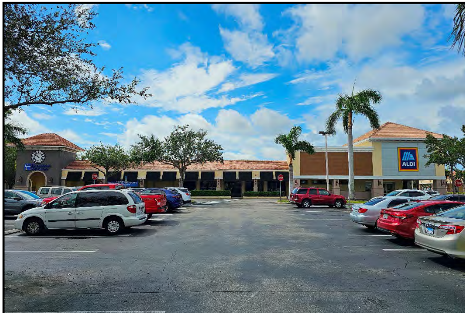
Photo 5.5. 8951 Bonita Beach Road SE (Bldg 2) (8LL02985), looking south.
