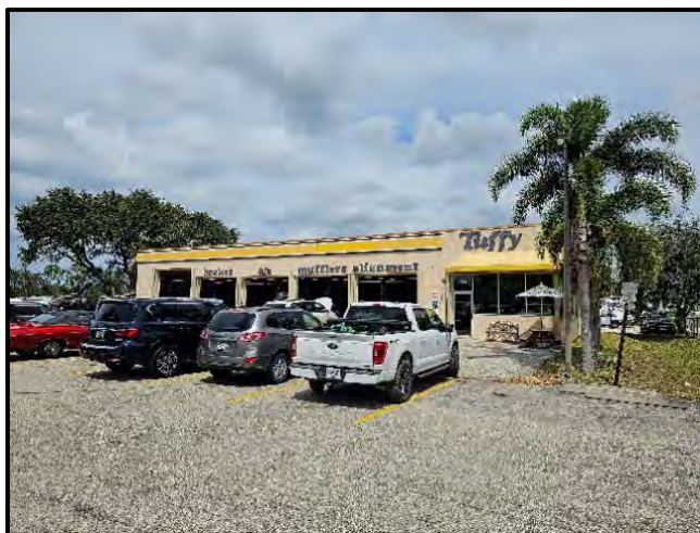
Photo 2.10. Building conditions within Pond West facing northwest.
