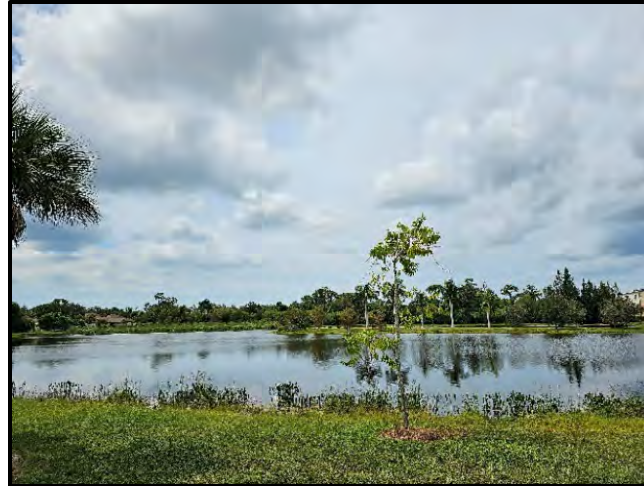
Photo 2.11. Conditions of existing Pond North from Arroyal Road facing southwest.
