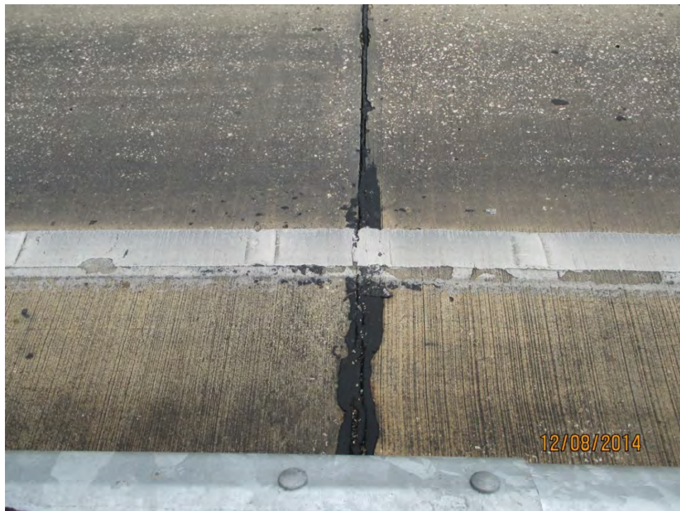
Photo 11: Homogeneous Area #3 (Samples 022T-024T) Black Expansion Fill, Deck (160133)
