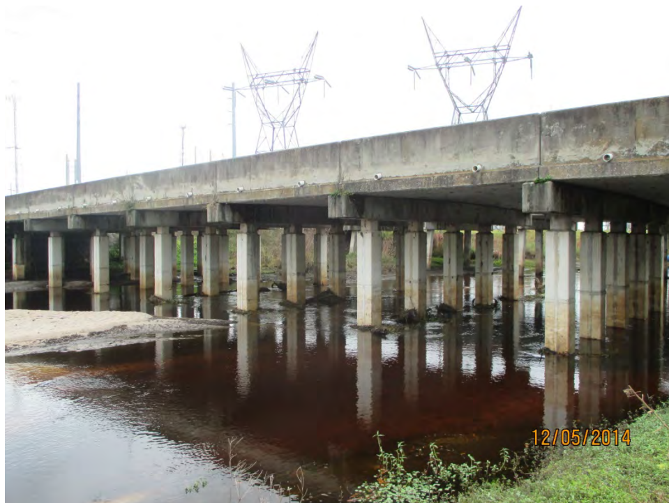
Photo 6: Homogeneous Area #5 (Samples 013B-015B) Smooth gray concrete w/ fiberglass coat, Pile (160045)
