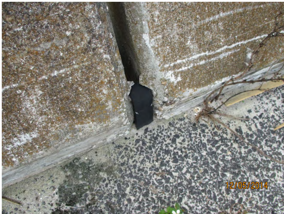
Photo 4: Homogeneous Area # 3 (Samples 007T-009T) Black expansion fill, Deck (160045)
