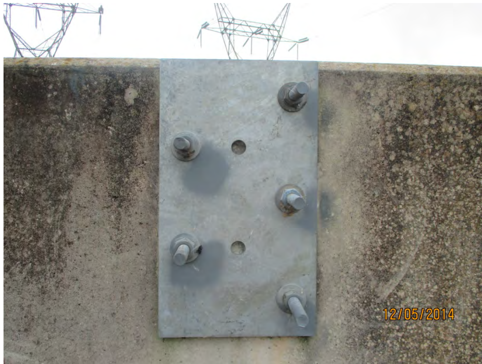
Photo 7: 2' x 1' steel mounting plate on Bridge Structure 160045 (Sample PC-1)
