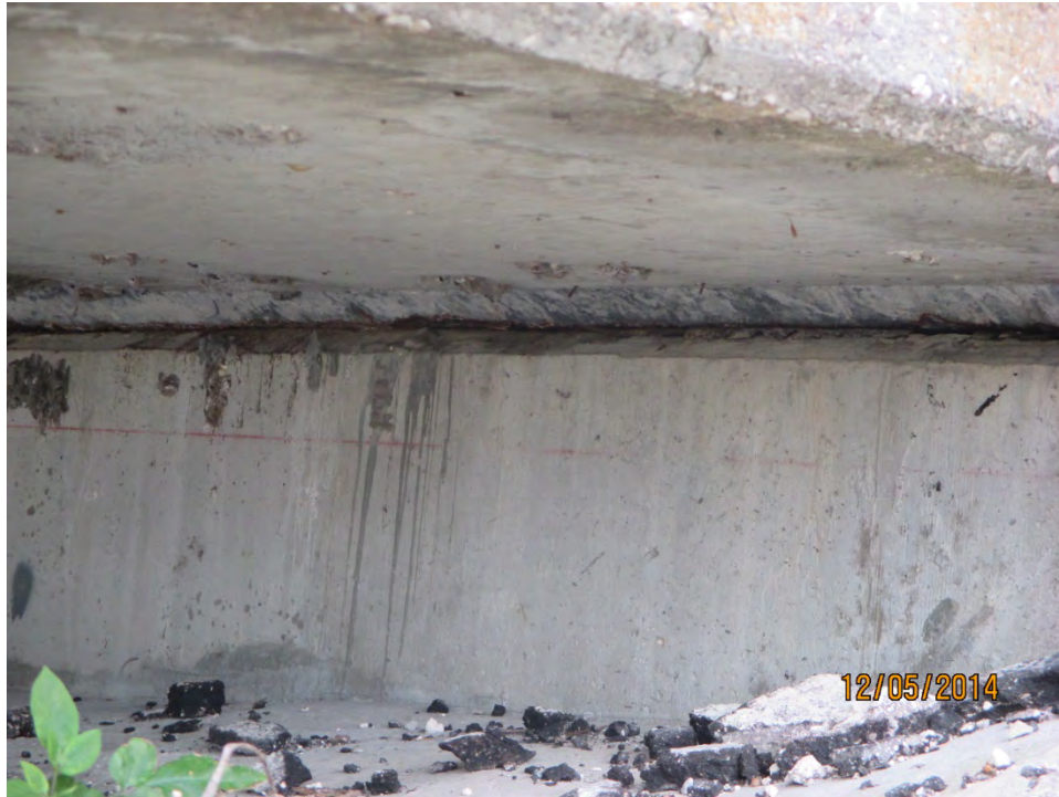
Photo 3: Homogeneous Area #2 (Samples 004B-006B) Black Tar Paper, Bent and Homogeneous Area # 6 (Samples 016B-018B) Light gray concrete, Deck (160045)
