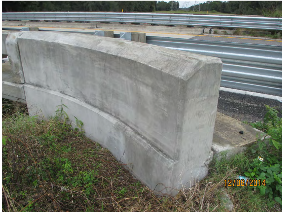
Photo 14: View of Homogeneous Area #6 (Samples 031S-033S) Light Gray Concrete, Wingwall (160133)
