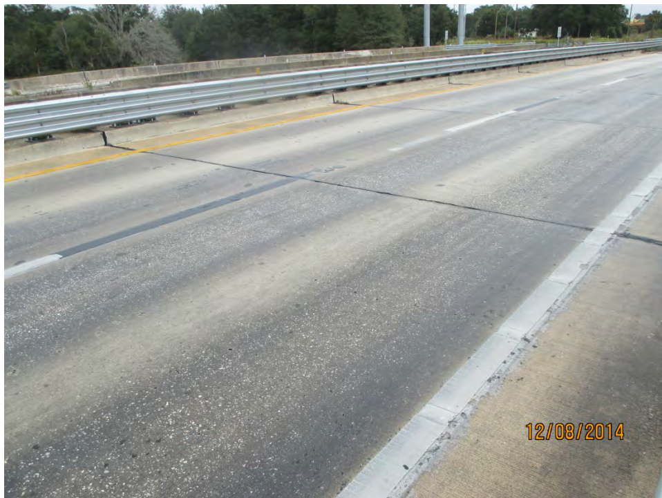
Photo 13: Homogeneous Area #5 (Samples 028T-030T) Gray Concrete w/ black coat, Deck (160133)
