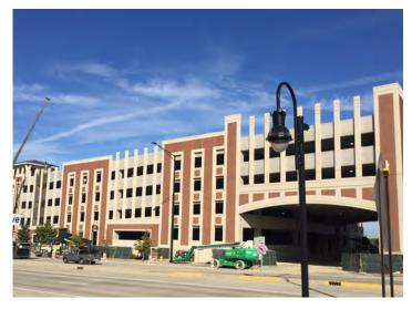
**City of Orland Park, IL Main Street Triangle** Five-level, precast concrete mixed-use parking structure with grade-level commercial and built over a street.
