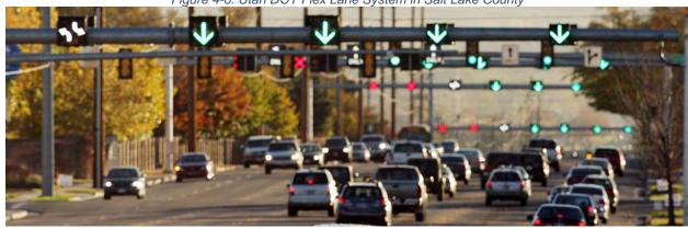
Figure 4-6: Utah DOT Flex Lane System in Salt Lake County
