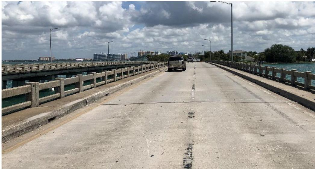
The existing bridges are relatively low to the water with approximately 10 feet of clearance at the center and approximately 4 to 5 feet at the bridge ends. Existing bridge plans from 1956 show an 800-foot vertical curve centered on the bridges with grades of 1.65% leading into each end of the vertical curve. The elevation of the Causeway throughout the project limits varies from approximately 4 feet to 8 feet.
