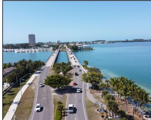
Within the project limits, the existing John Ringling Boulevard is classified as an Urban, Minor Arterial and consists of a four-lane, divided facility between Bird Key Drive and Sarasota Harbour West.
