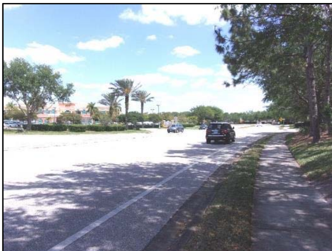
Photo 5. Conditions along Cattlemen Road.
