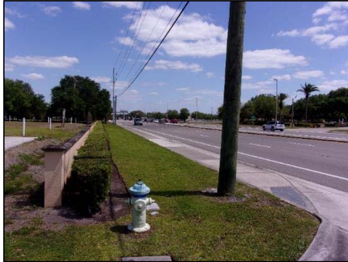
Photo 6. Conditions in vicinity of Honore Road.
