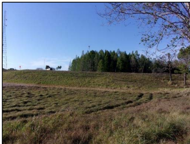
Photo 2. Conditions at the northbound interchange.
