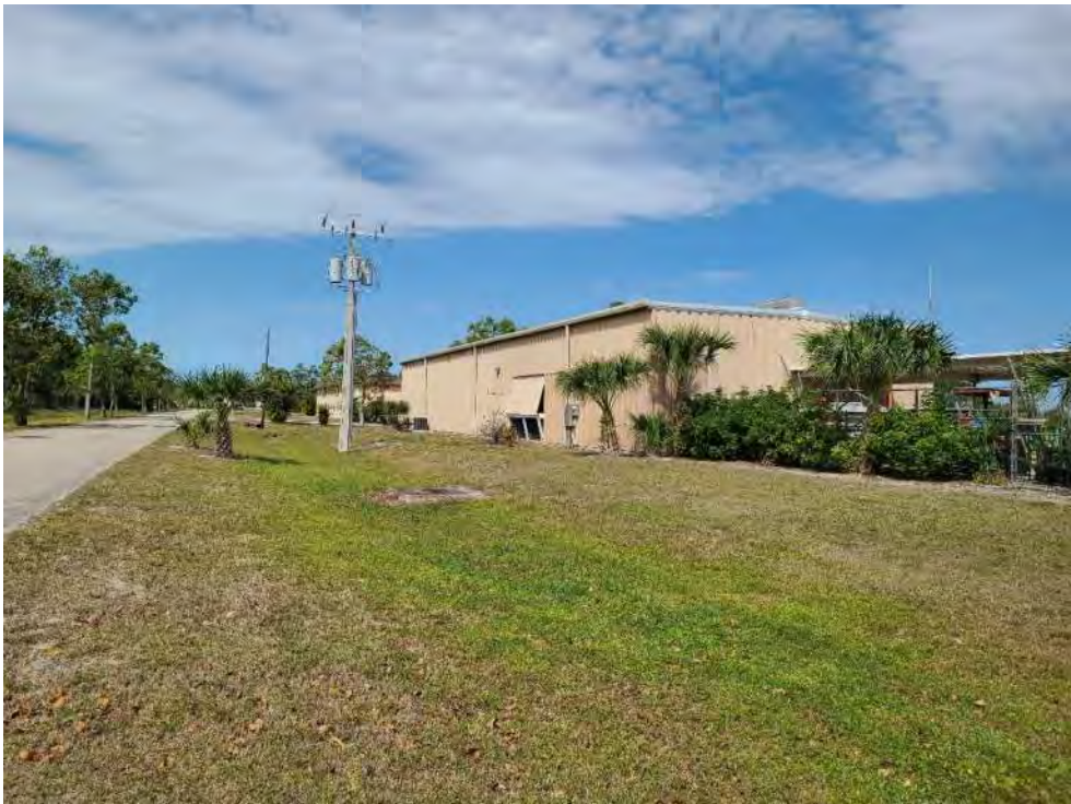
Site 24 – Maintenance Building Compound Road looking northwest
