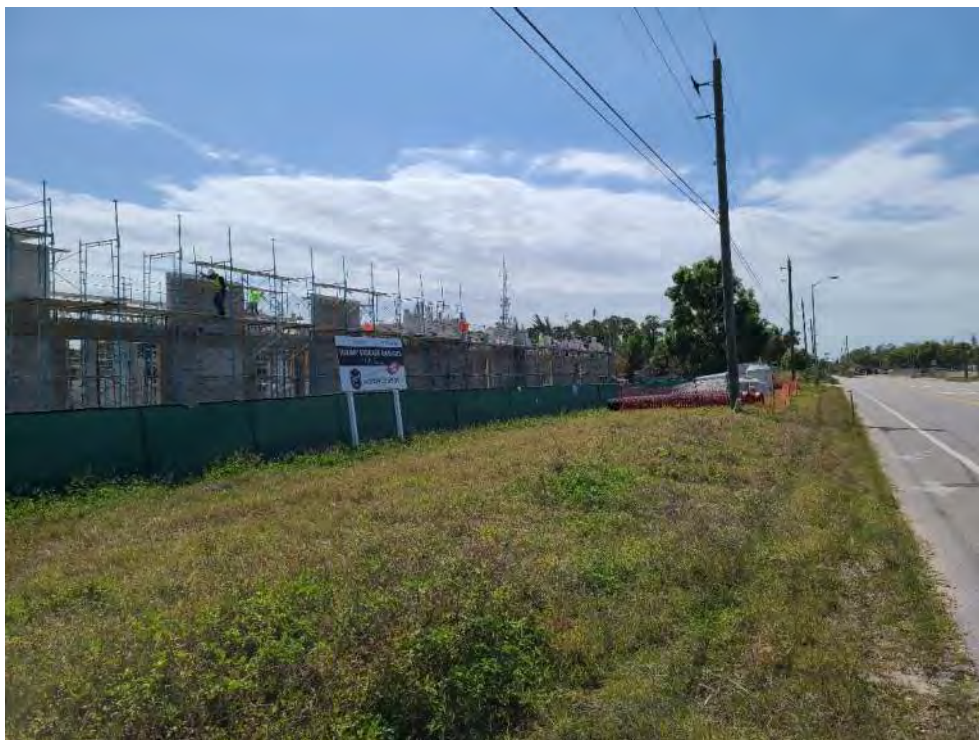
Site 29 – Race Track Road Construction Site Race Track Road looking southeast
