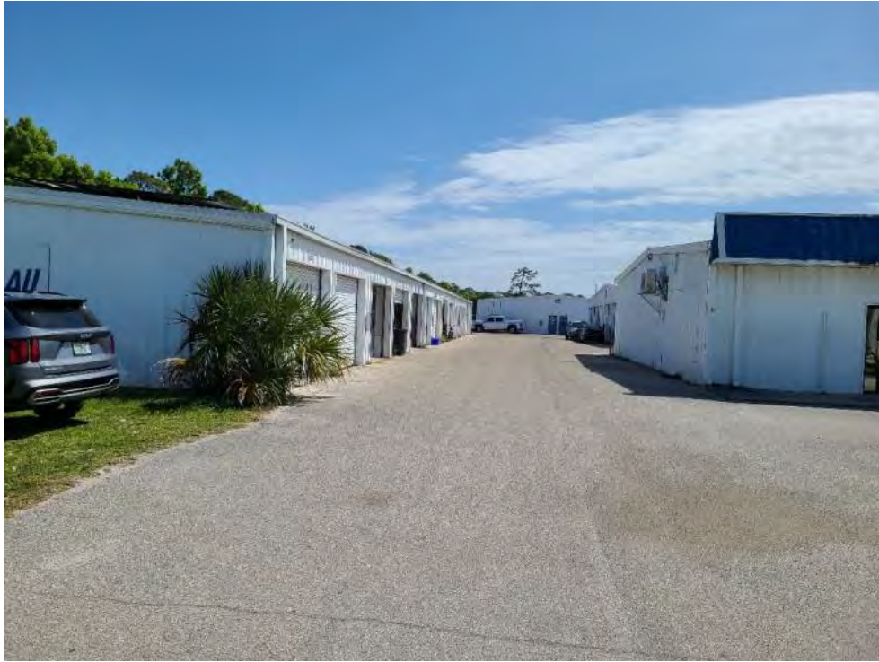
Site 28 – Component Technology, Inc. Race Track Road looking east
