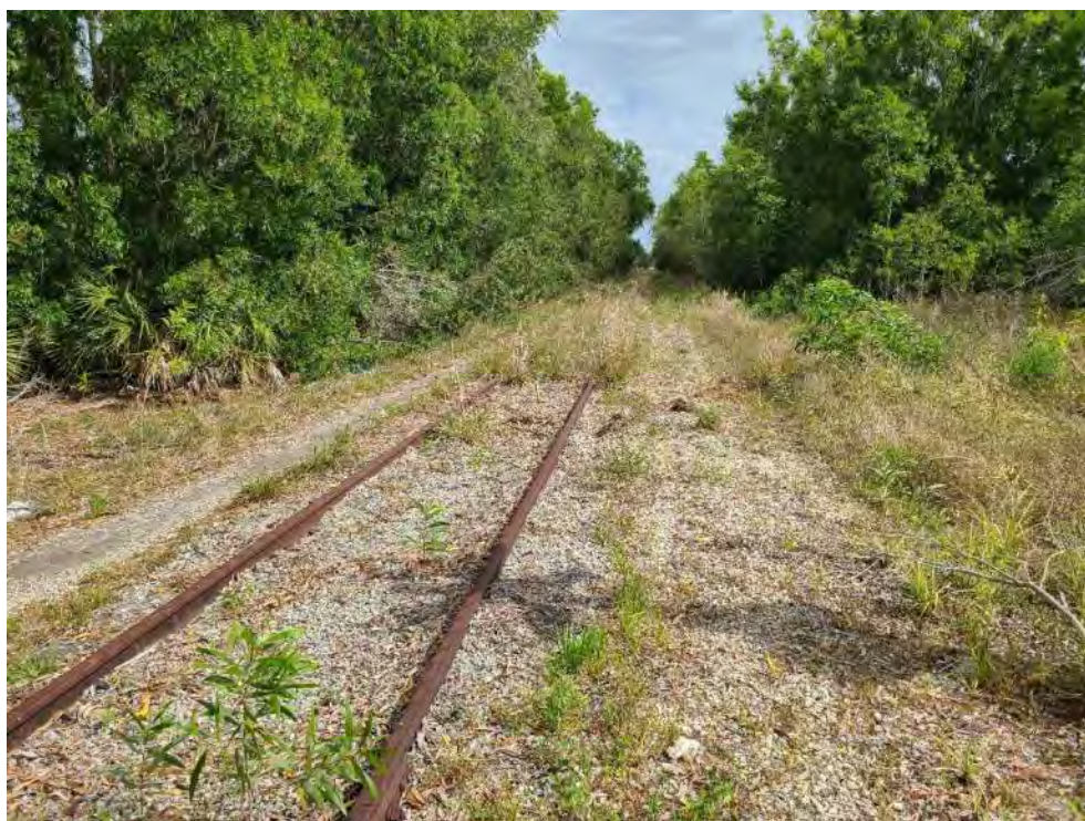
Site 17 – Railroad Near Channel 30 Drive looking northeast
