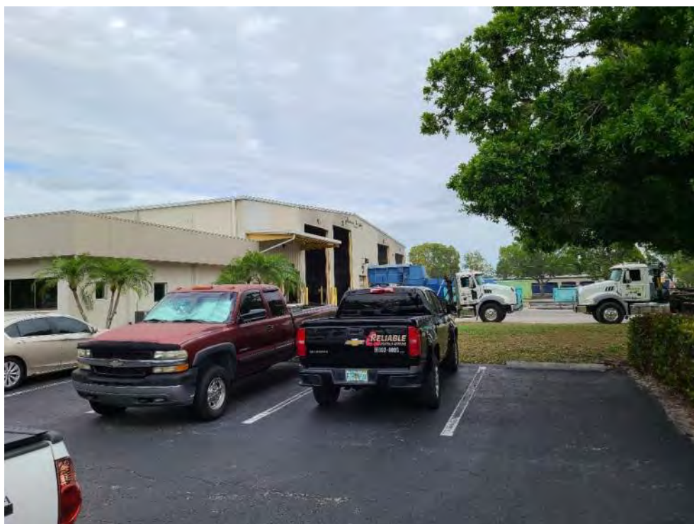
FPC 3 Near the southeastern corner looking north
