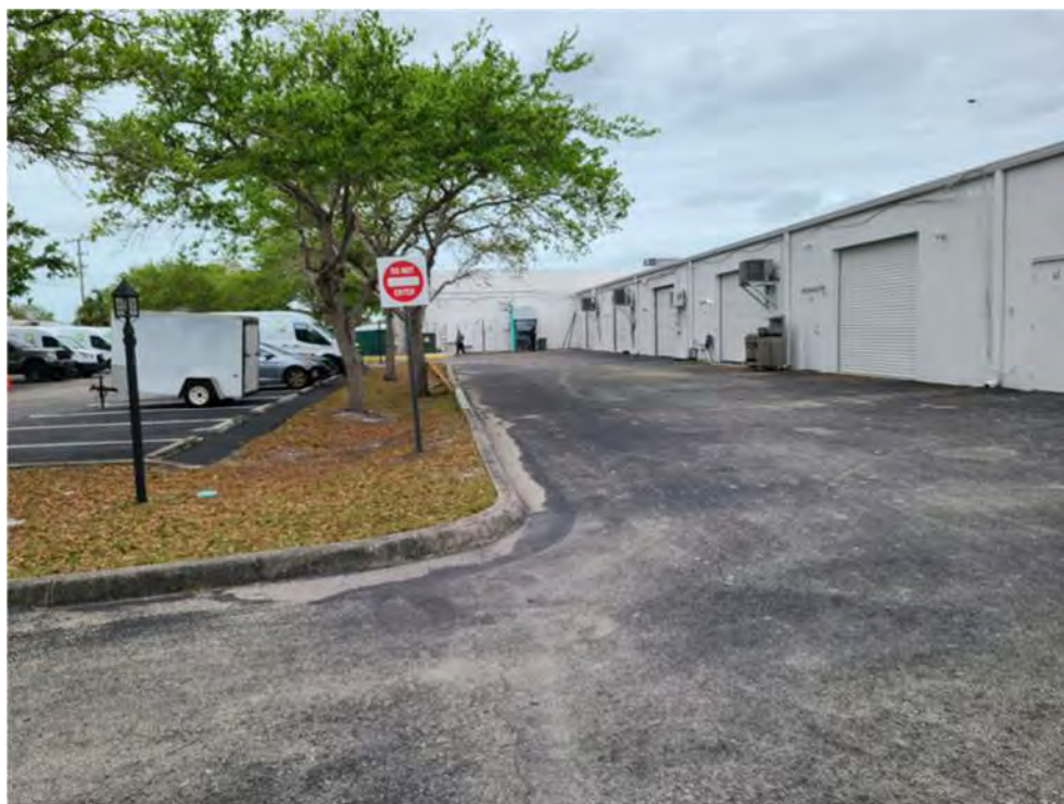
FPC 2 Near the eastern boundary looking west
