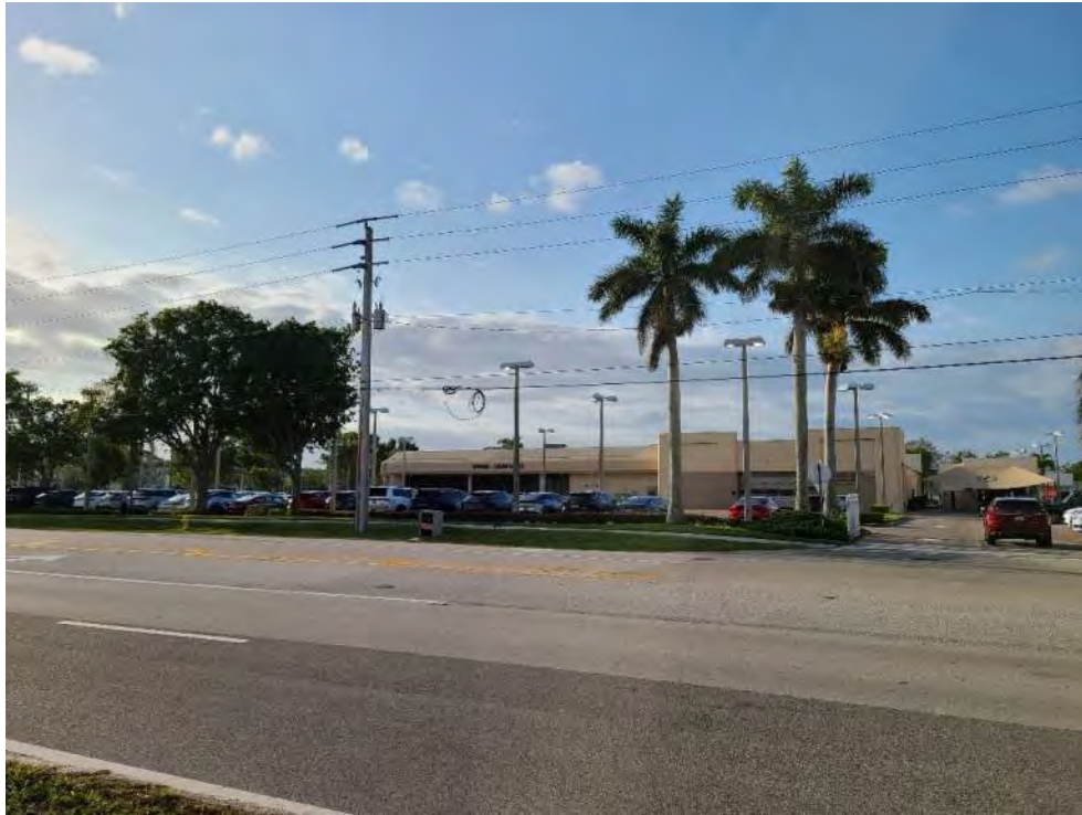
Site 1 – Germain Lexus (Former Germain Lincoln Mercury) Wiggins Pass Road looking southeast
