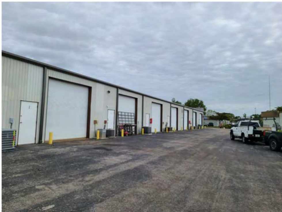
FPC 2 Near the western boundary looking north
