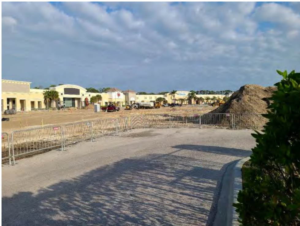
Site 2 – Construction Site Gateway Shoppes Plaza looking northwest
