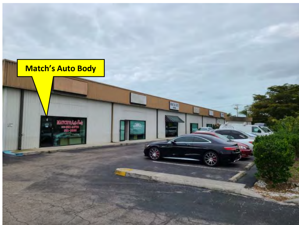
Site 8 – Match's Autobody Near Rail Head Boulevard looking southwest
