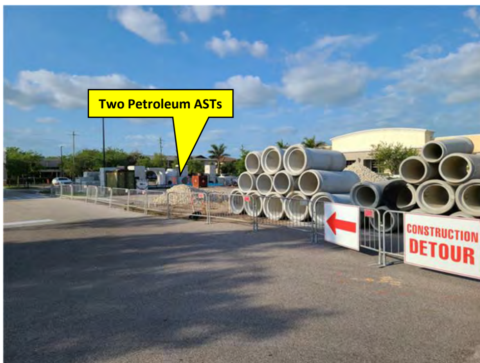
Site 2 – Construction Site Gateway Shoppes Plaza looking southwest
