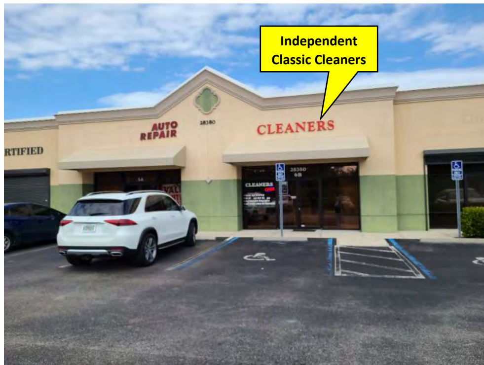
Site 21 – Independent Classic Cleaners (Formerly Gold Coast Custom Drycleaners) Near Old US 41 Road looking west
