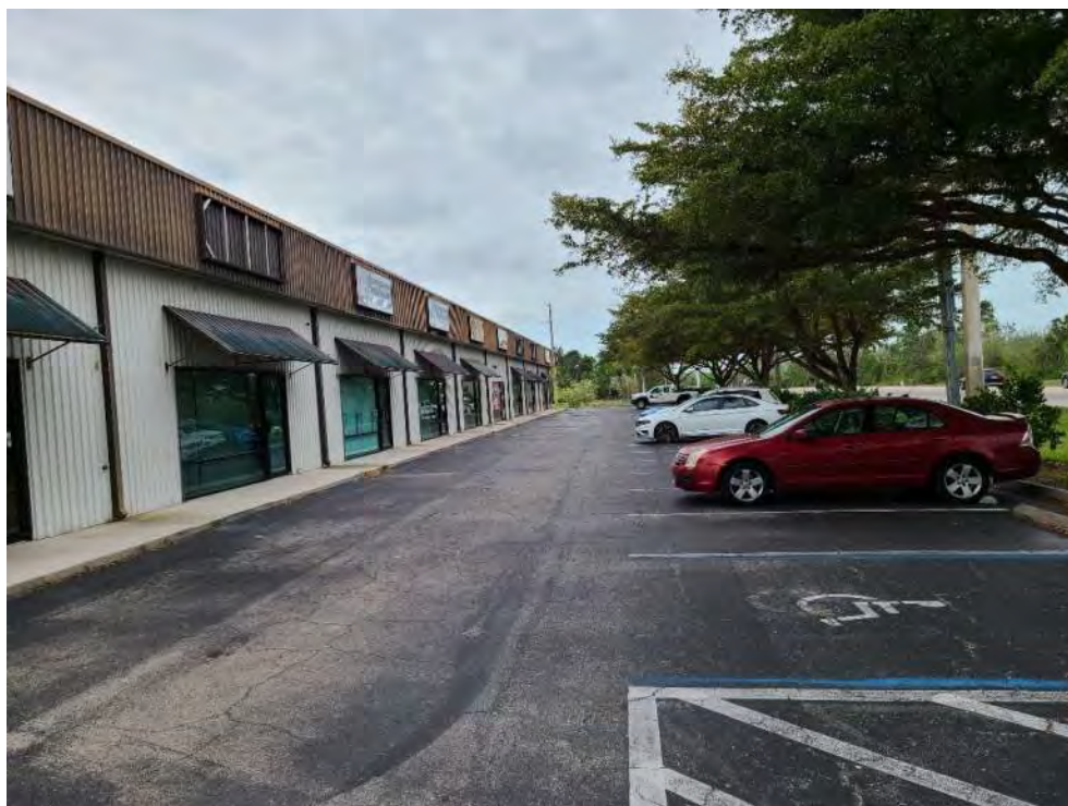
FPC 2 Near the northwestern corner looking southwest
