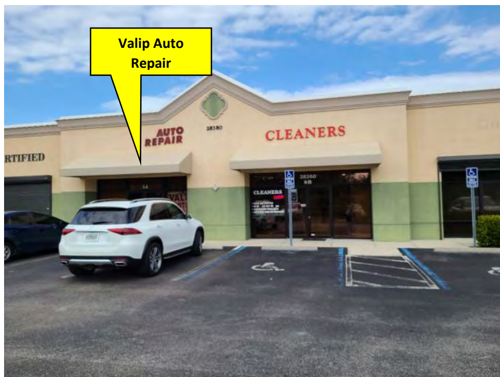
Site 20 – Valip Auto Repair Near Old US 41 Road looking west
