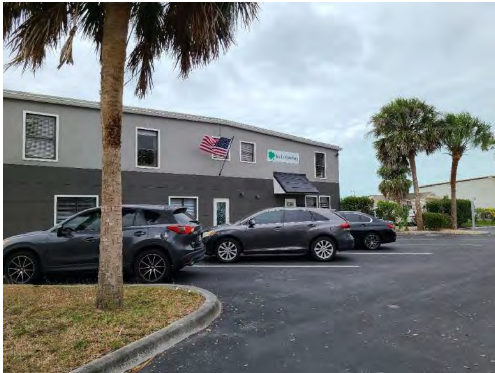
Site 9 – Kelly Roofing (Former American Equipment) Rail Head Boulevard looking southwest
