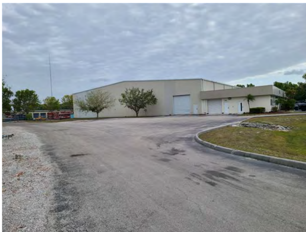
FPC 3 Near the southwestern corner looking northeast
