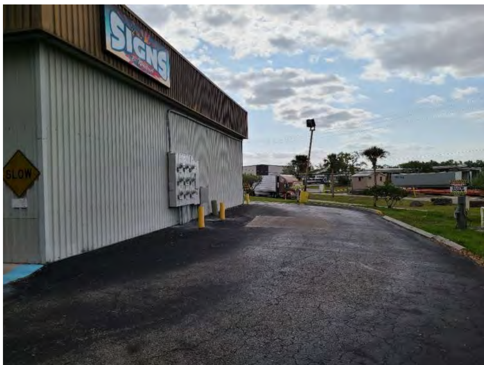
FPC 2 Near southwestern corner looking southeast
