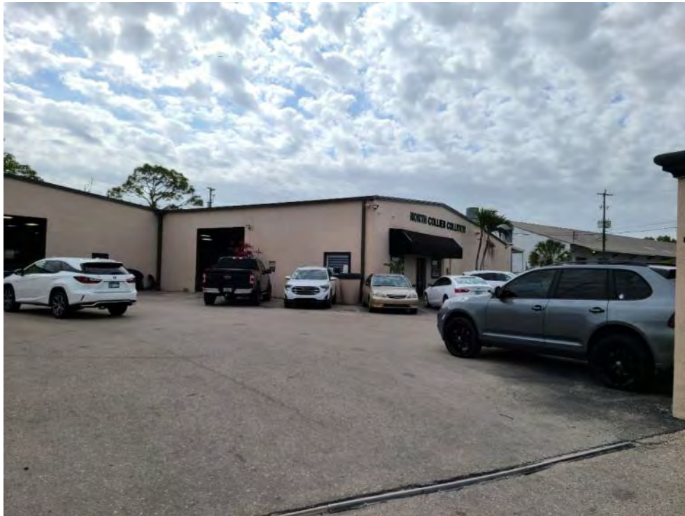
Site 14 – North Collier Collision Old US 41 Road looking southeast
