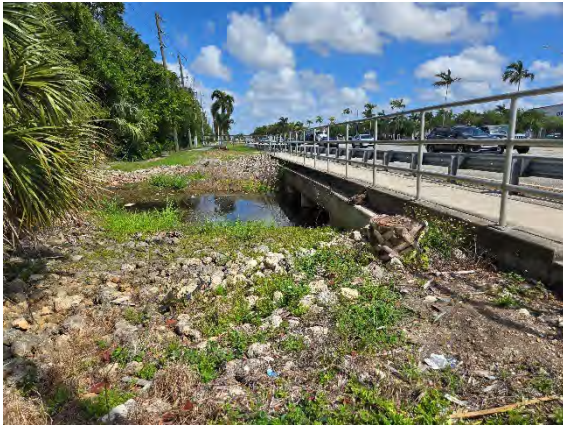
Photo 2.5. View of canal and bridge along west side of Tamiami Trail, facing north.
