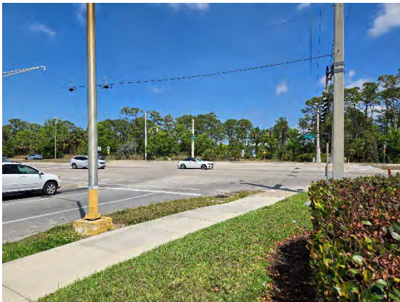
Photo 2.19. Intersection from southeast corner of Race Track Road and Bonita Beach Road in the northeast end of the project, facing northwest.
