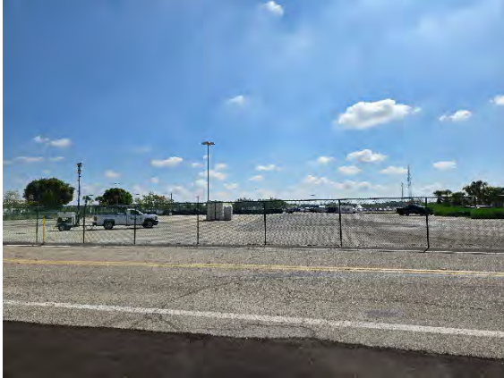
Photo 2.15. General view of parking lot in northeast end of the project, facing northeast.
