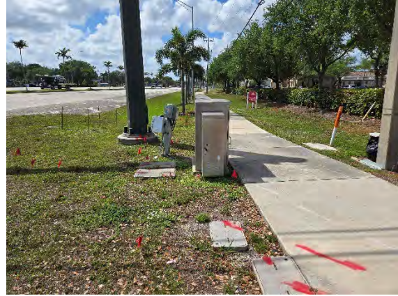
Photo 2.4. Example of utilities along the west side of Tamiami Trail, facing south.
