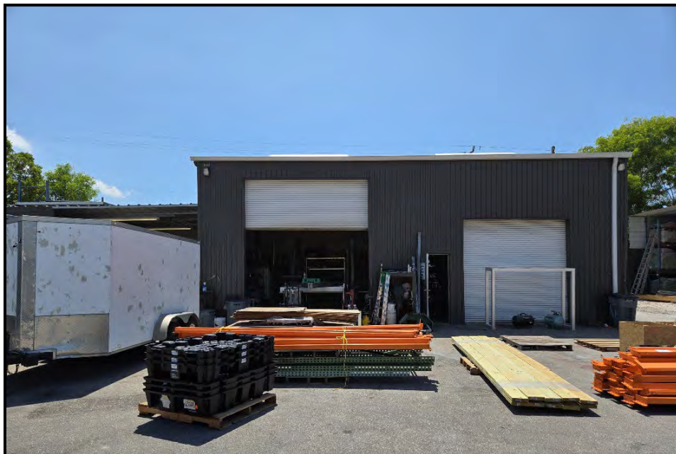
Photo 5.3. 1360 Rail Head Boulevard (Building 1) (8CR01664), looking south.
