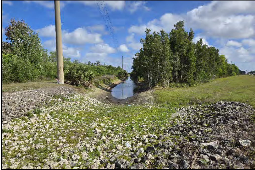
Photo 5.8. Transmission Corridor Canal (8CR01669), looking north.
