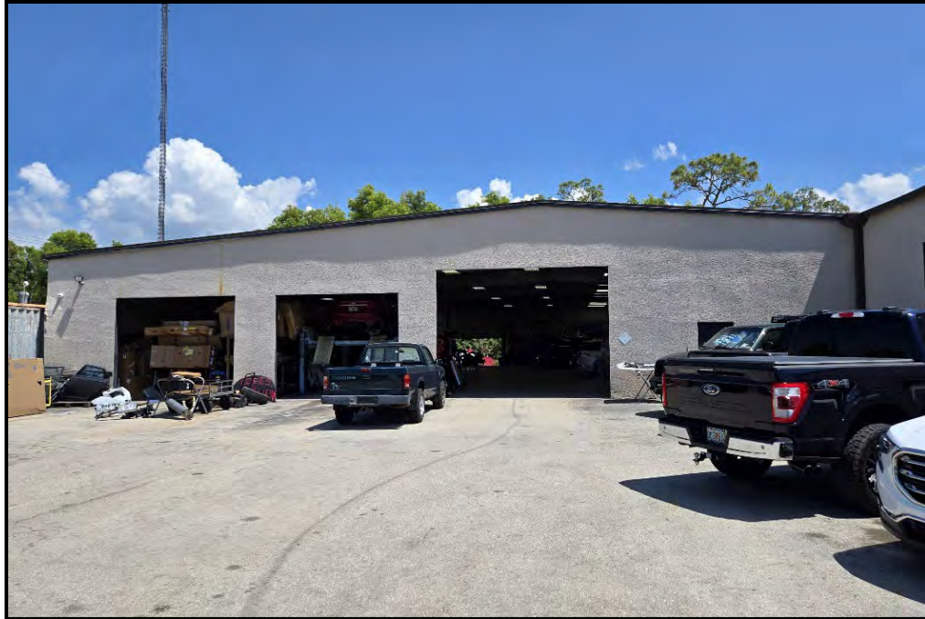
Photo 5.7. 16210 Old 41 Road (Building 2) (8CR01668), looking east.
