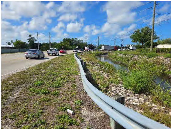
Photo 2.7. View of drainage canal along west side of CR 887 (Old US 41) separated by guard rail, facing southwest.
