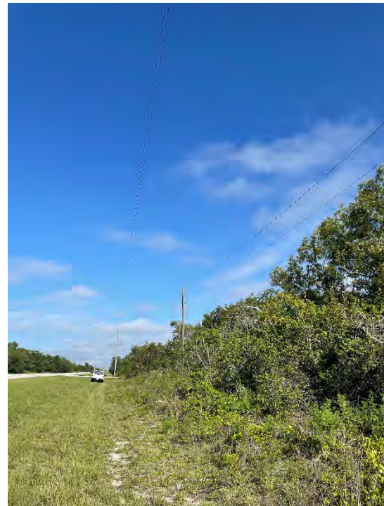
Survey Station No. 42 – Facing West
