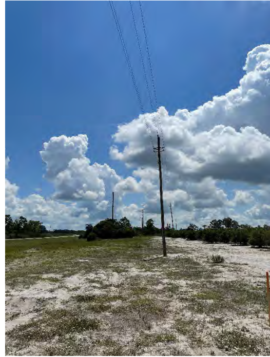
Survey Station No. 2 – Facing East
