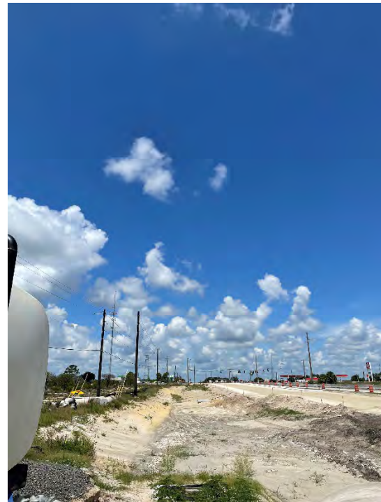
Survey Station No. 11 – Facing West
