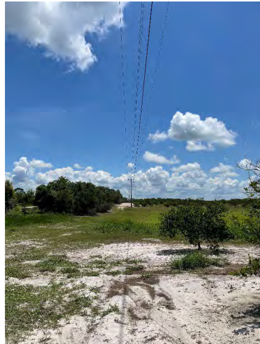
Survey Station No. 17 – Facing East
