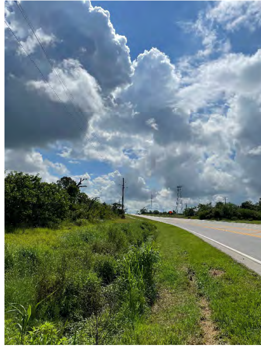
Survey Station No. 57 – Facing East
