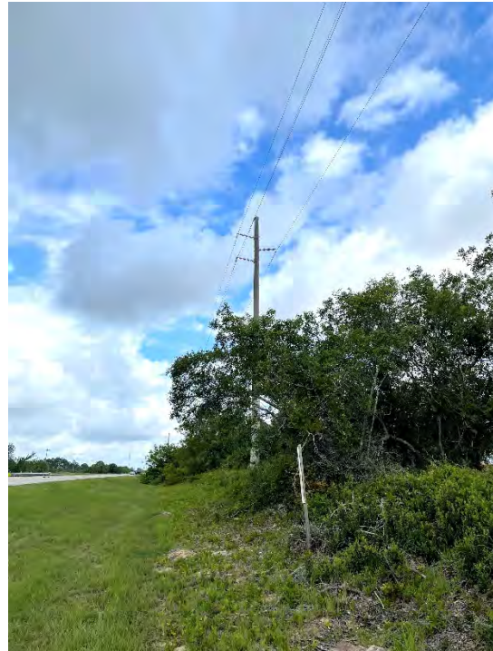
Survey Station No. 50 – Facing West
