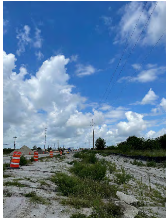
Survey Station No. 53 – Facing West
