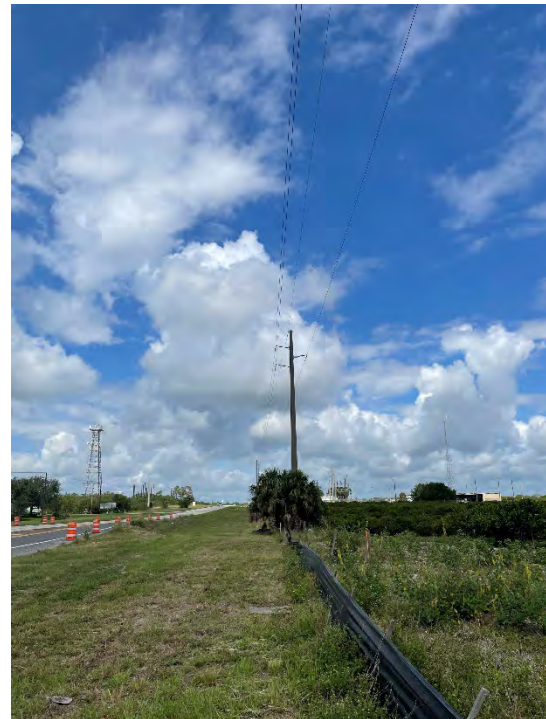
Survey Station No. 54 – Facing West
