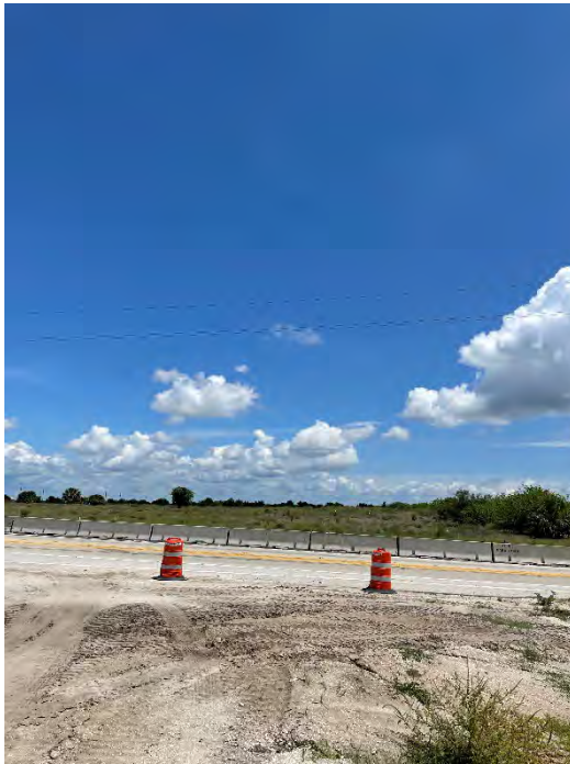
Survey Station No. 11 – Facing North
