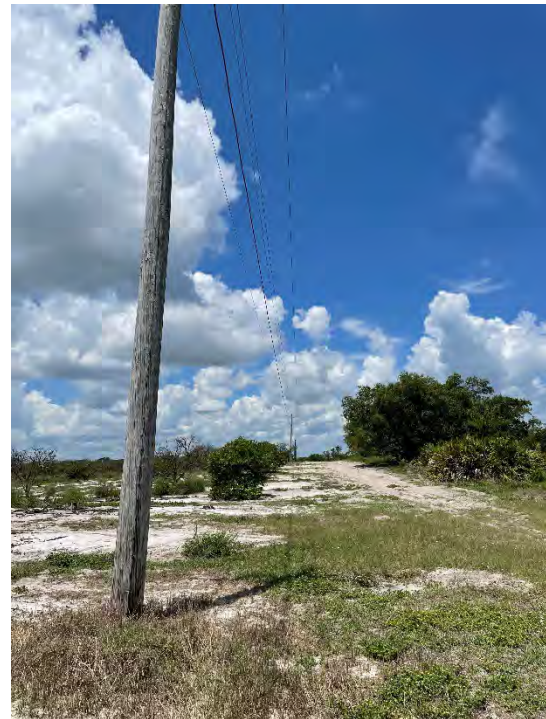
Survey Station No. 17 – Facing West
