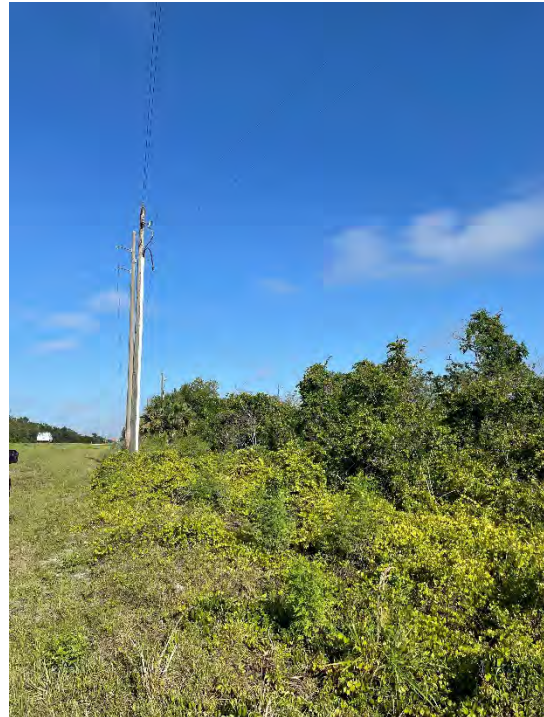
Survey Station No. 41 – Facing West
