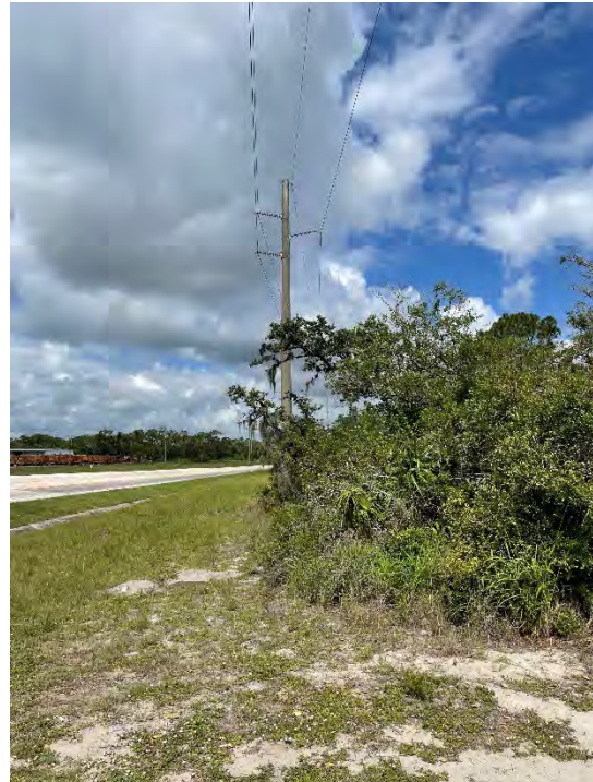
Survey Station No. 56 – Facing West
