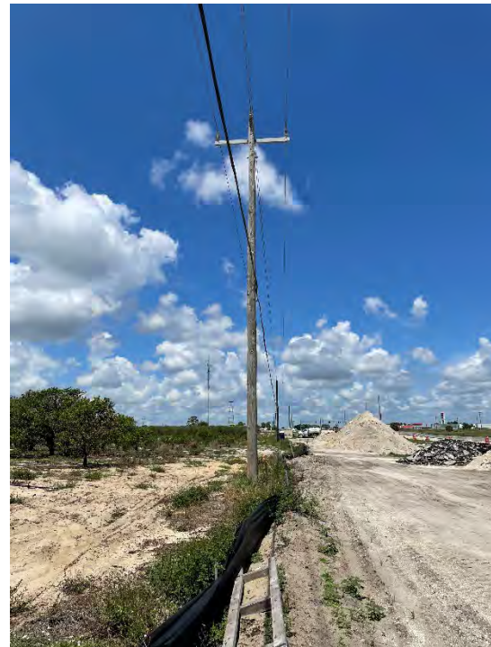
Survey Station No. 12 – Facing West
