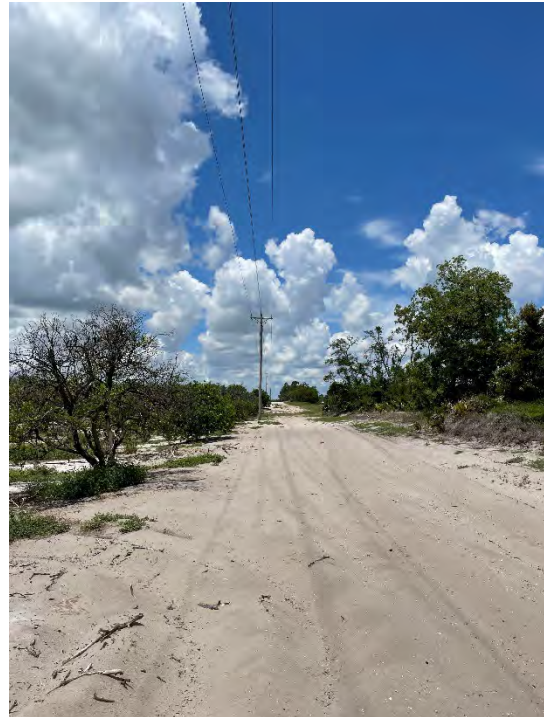
Survey Station No. 19 – Facing West
