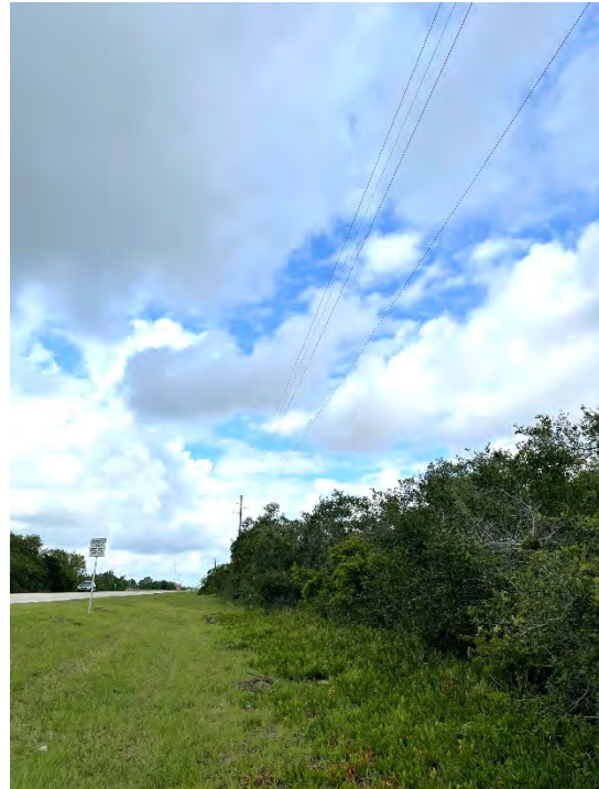
Survey Station No. 49 – Facing West
