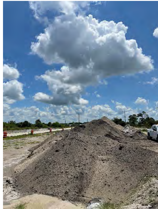
Survey Station No. 11 – Facing East
