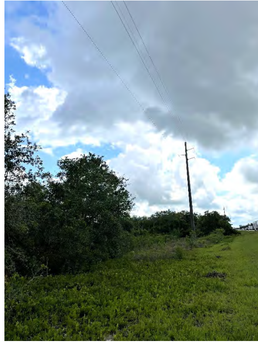
Survey Station No. 49 – Facing East
