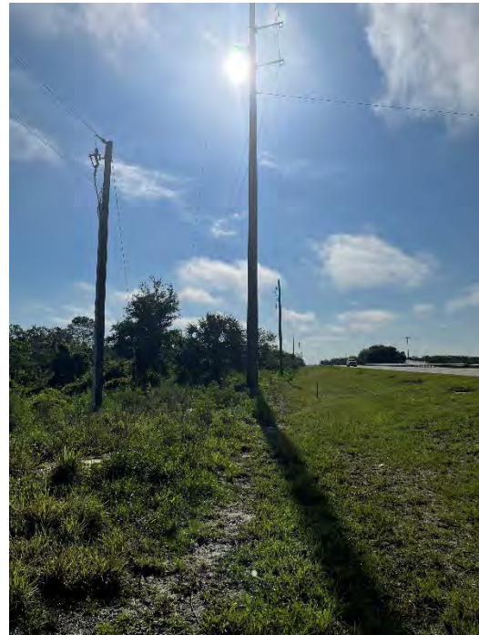
Survey Station No. 42 – Facing East
