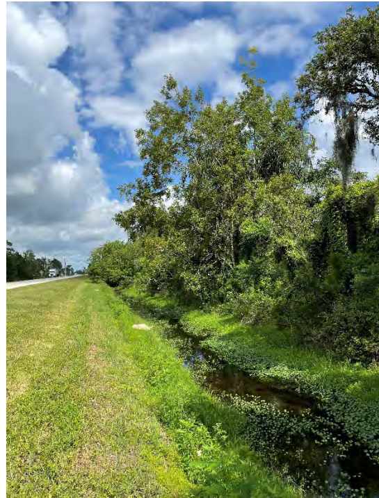
Survey Station No. 59 – Facing West
