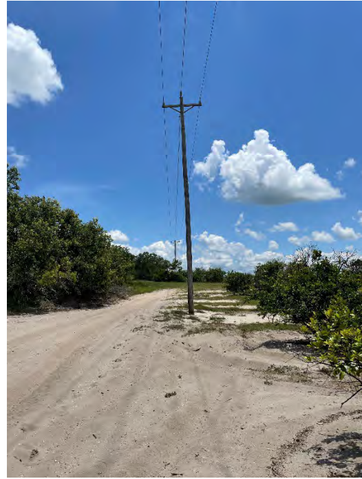
Survey Station No. 19 – Facing East
