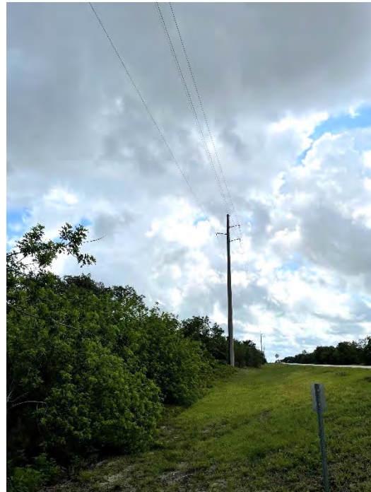
Survey Station No. 47 – Facing East
