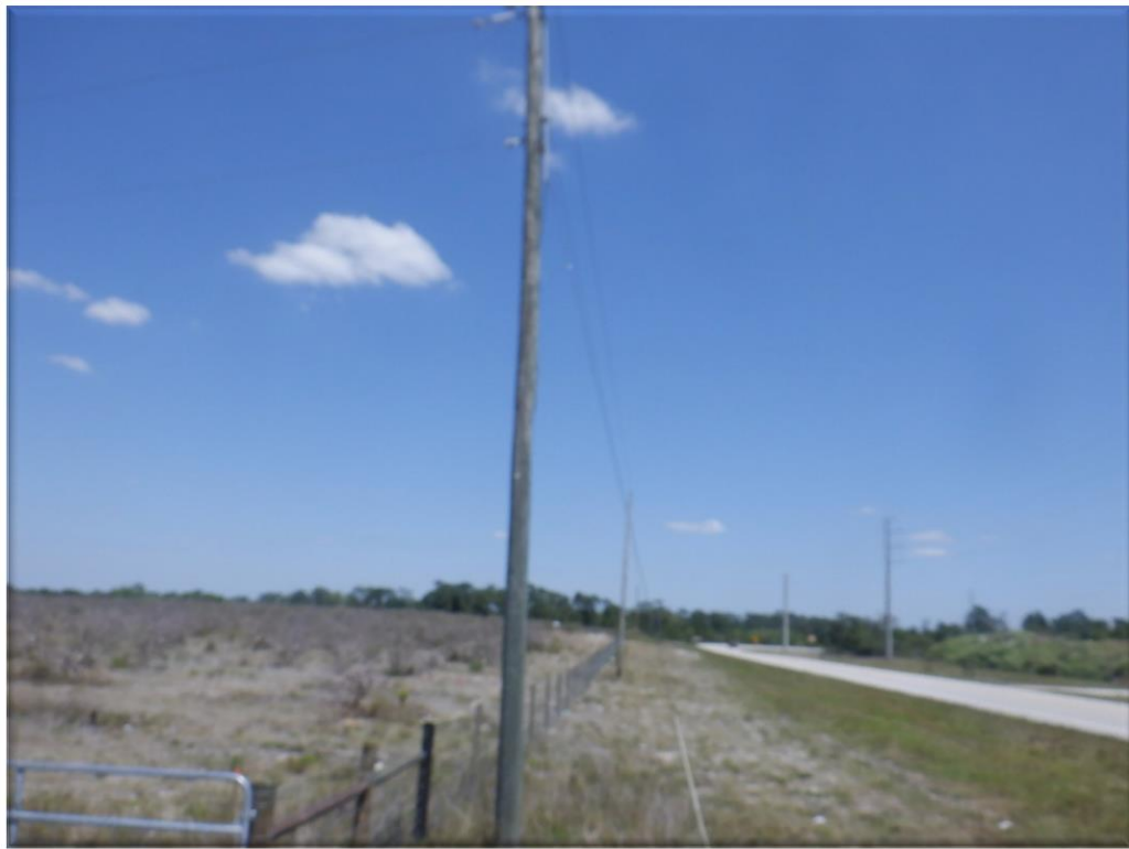
Photo 16: Survey Station 4, facing east
