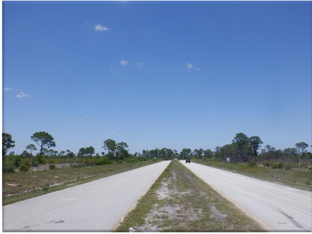
Photo 1: Survey Station 1, facing north
