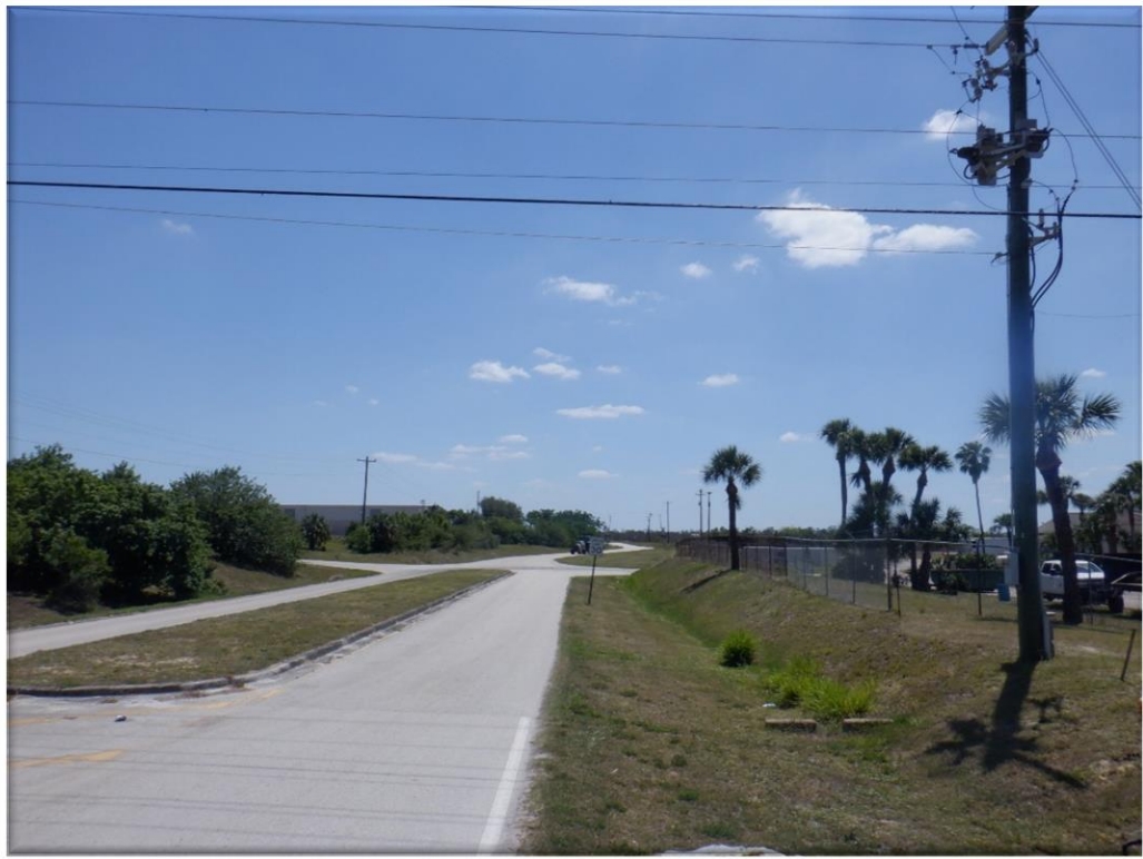
Photo 18: Survey Station 5, facing south
