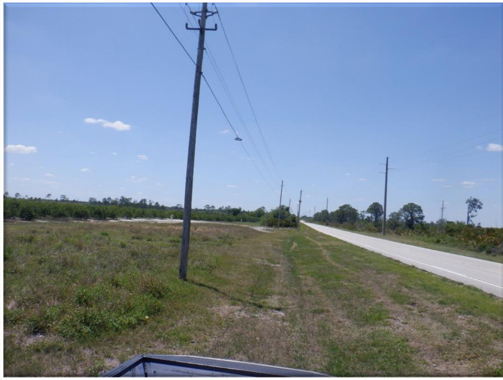
Photo 11: Survey Station 3, facing west
