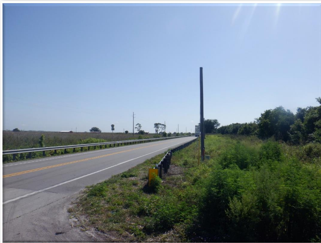
Photo 32: Survey Station 8, facing east
