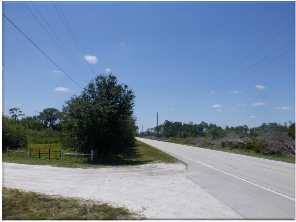
Photo 7: Survey Station 2, facing west
