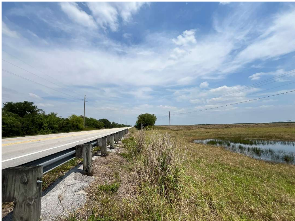
Survey Station No. 16 – Facing East
