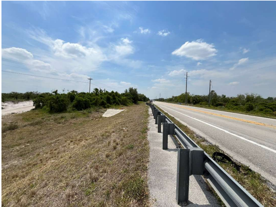
Survey Station No. 17 – Facing West
