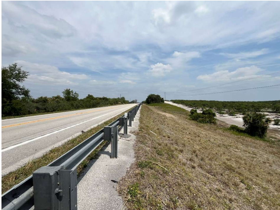
Survey Station No. 17 – Facing East
