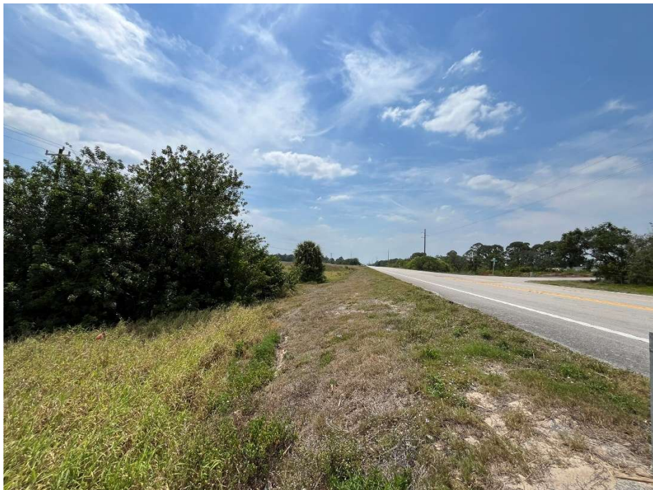
Survey Station No. 16 – Facing West
