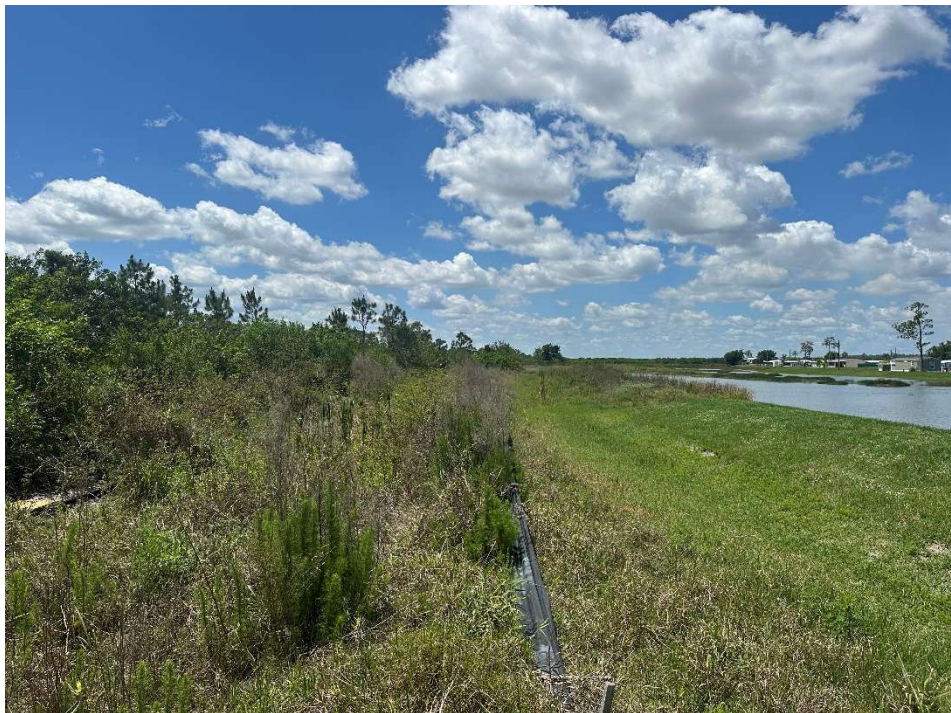
Survey Station No. 15 – Facing South
