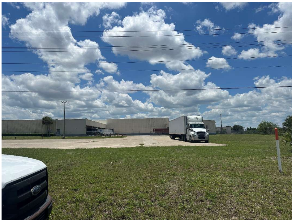
Survey Station No. 13 – Facing South
