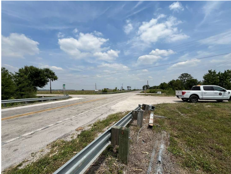
Survey Station No. 19 – Facing East
