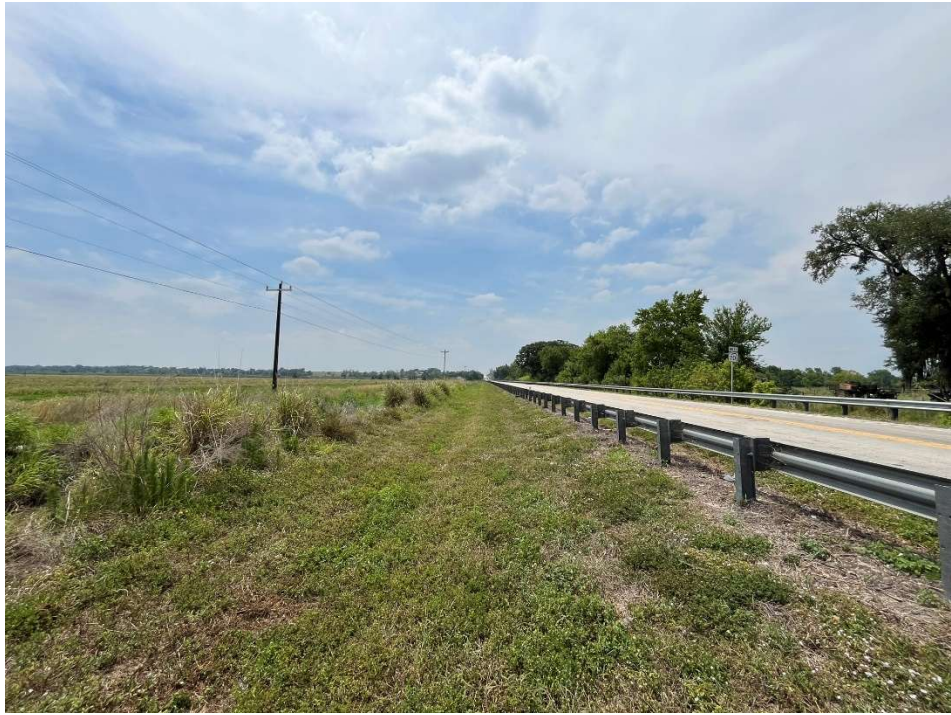
Survey Station No. 19 – Facing West
