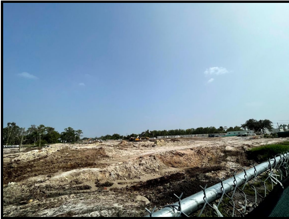
Photo 5: Area under construction adjacent to project limits
