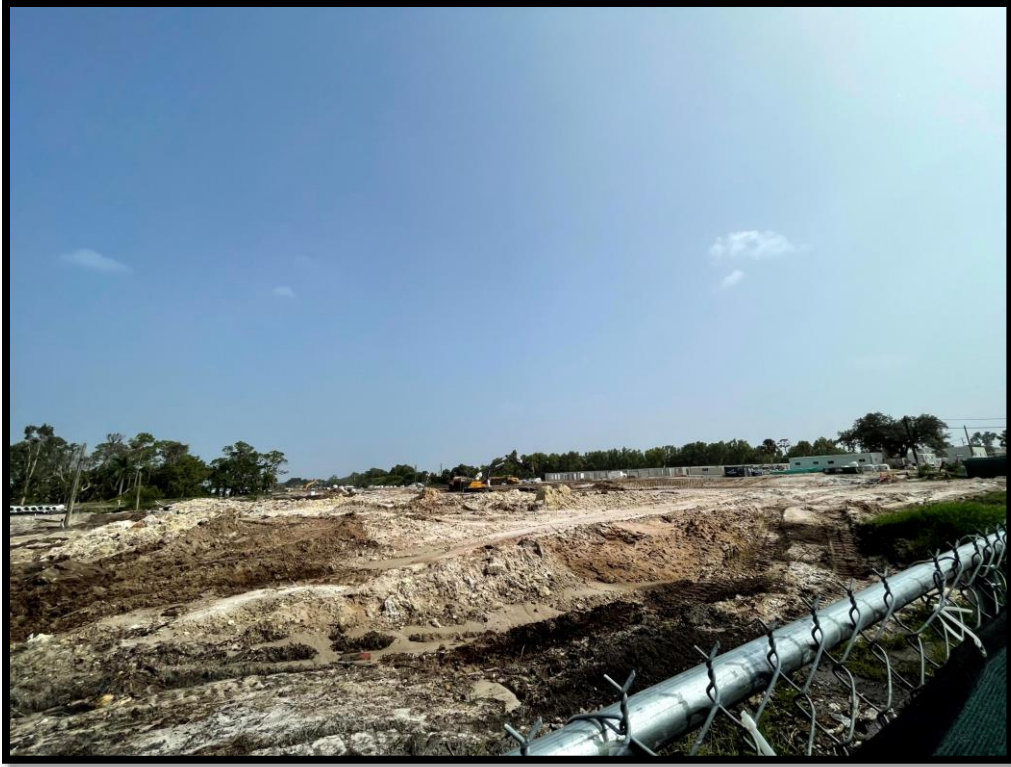
Photos: Area Under Construction
