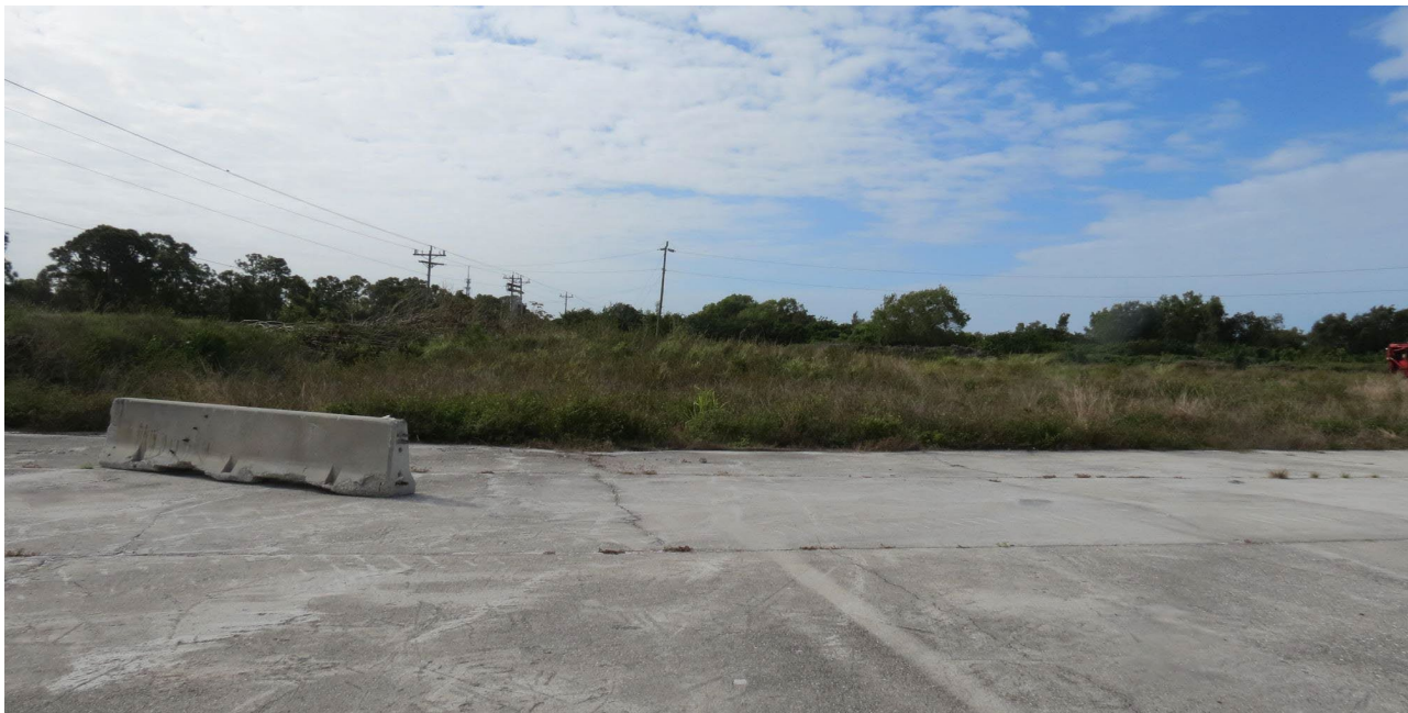
Photo 20. Contamination Site #3: Facing south from mid-way into concrete loading area. Some remaining vegetative matter to be used for soil remains. Typically, the access fence is kept locked to prevent dumping.
