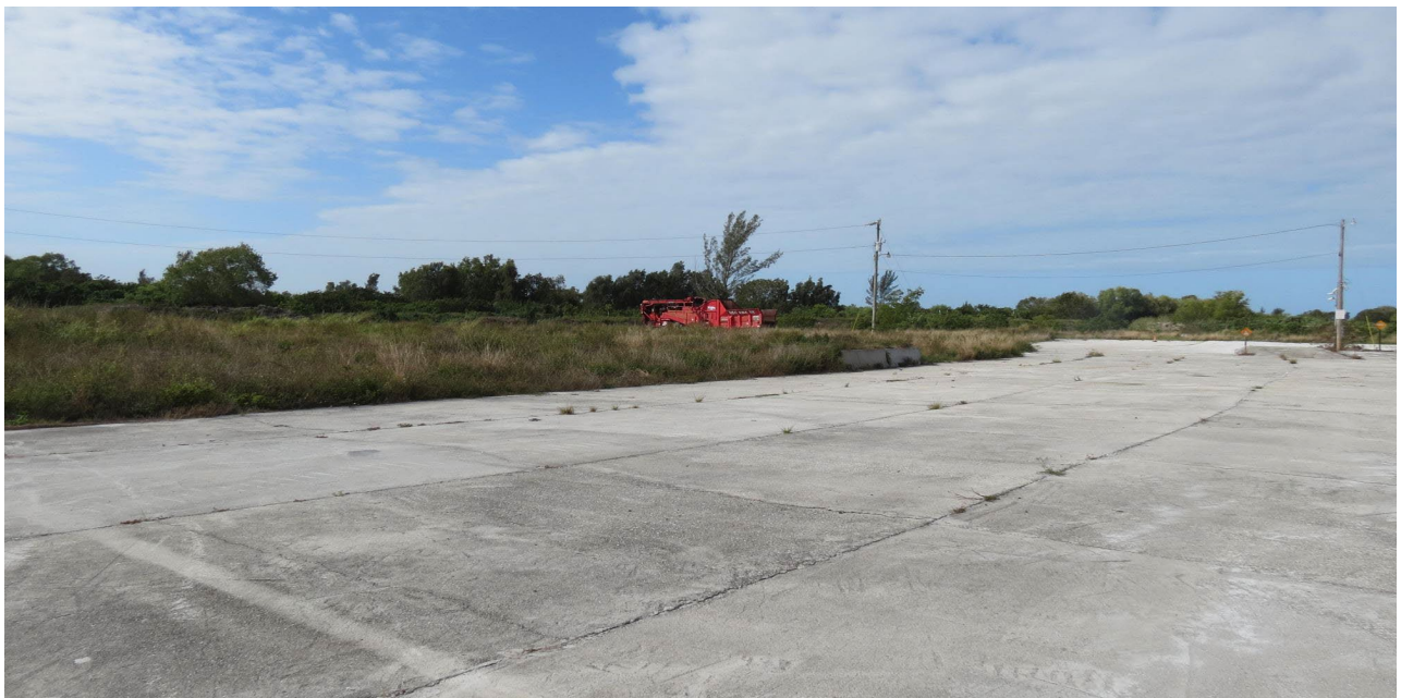
Photo 18. Contamination Site #3: Facing southeast at last remaining heavy equipment on former Cape Recycling facility. This was picked up the same day.
