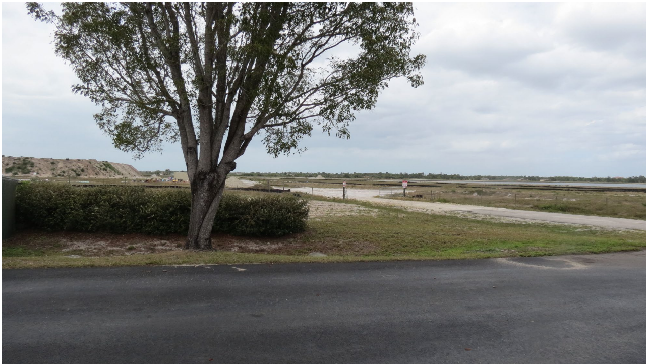
Photo 24. Facing west. New luxury motorcoach development using NW 40 th Lane along north side of fire station.
