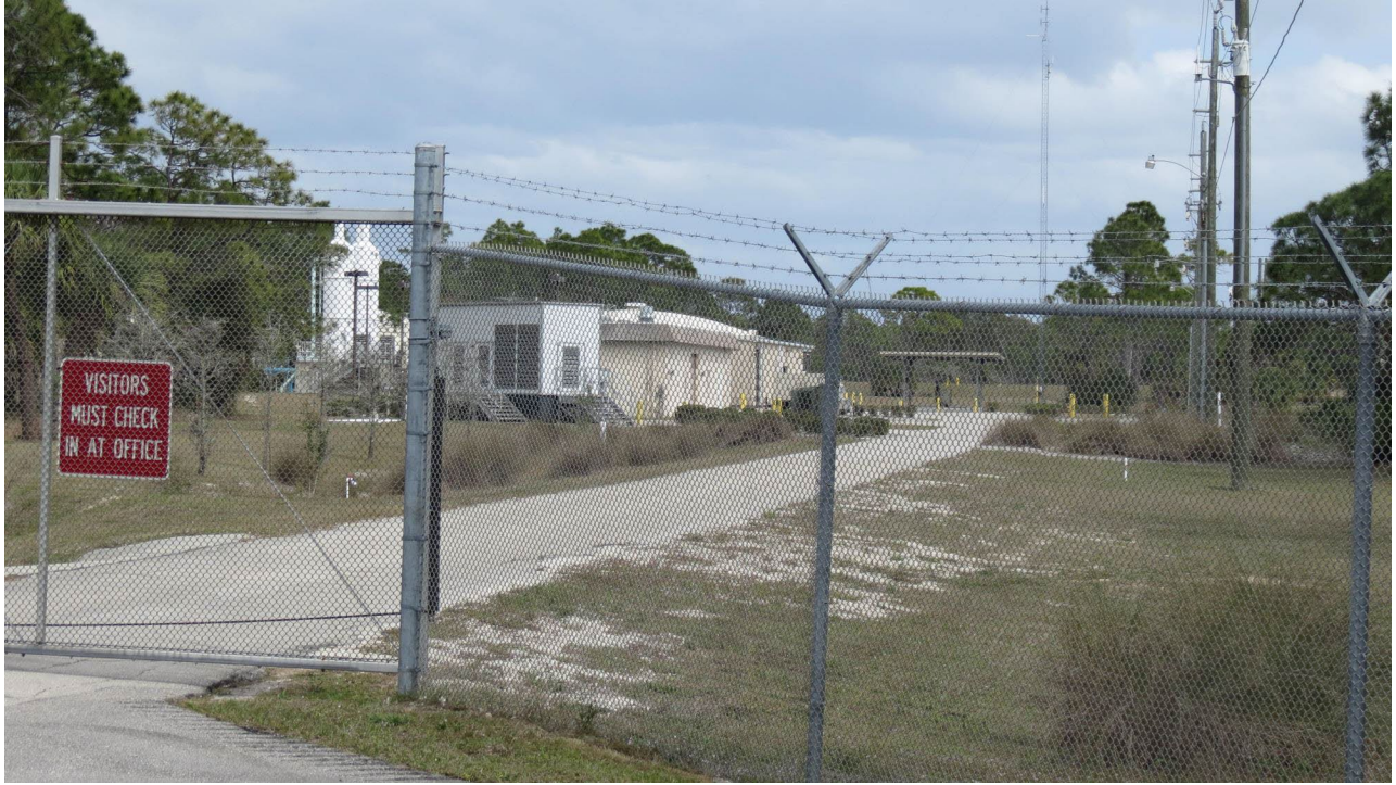
Photo 31. Contamination Site #6: Facing east at Water Reclamation facility. Emergency generator with below generator fuel tank. Site closed for the day.
