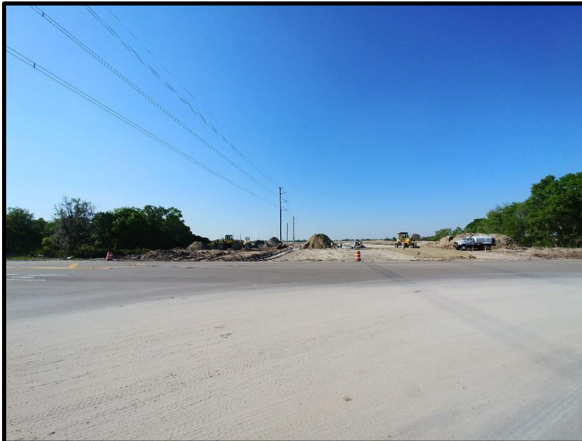
Photo 2.9. Looking south, southeast towards proposed roundabout at Bourneside Boulevard.
