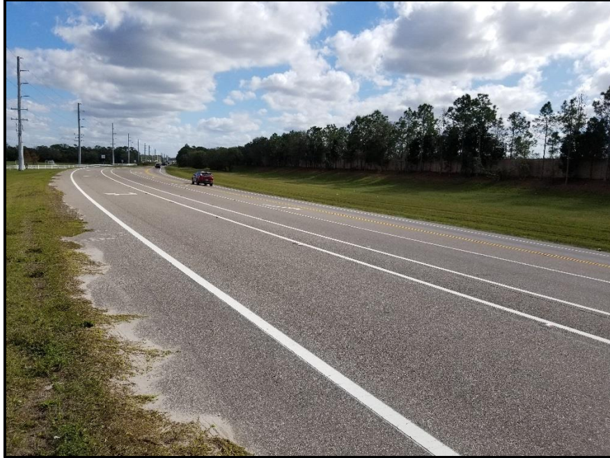
Photo 5.2. Looking at SR 70 from Post Boulevard.
