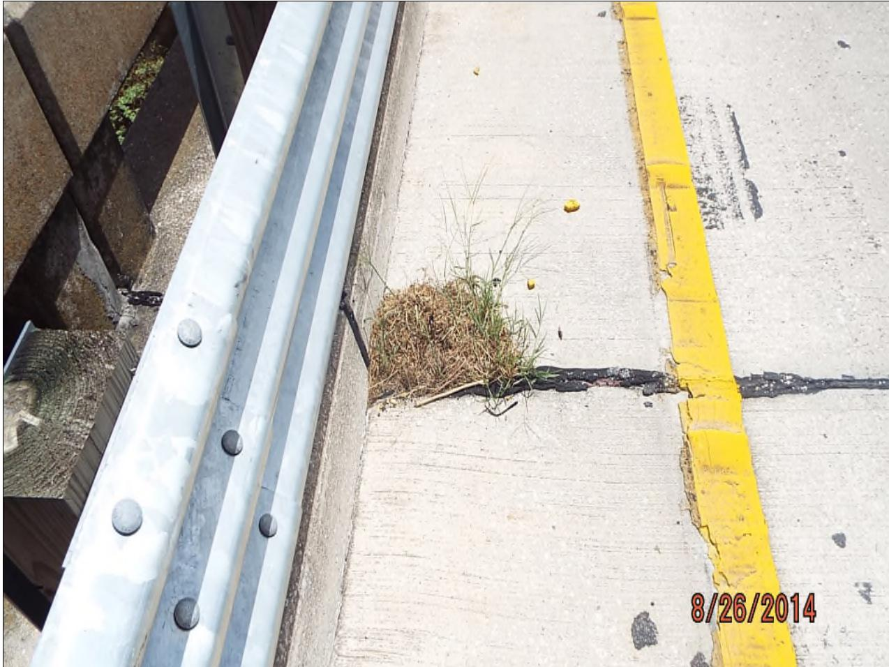
**Photo 1 - Element 301/3 Pourable Joint Seal**
