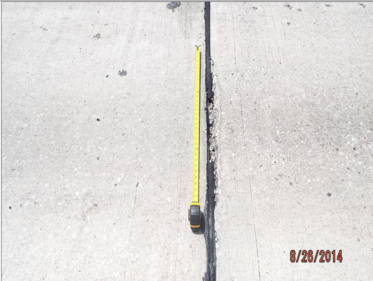
**Photo 2 - Element 301/3 Pourable Joint Seal**
