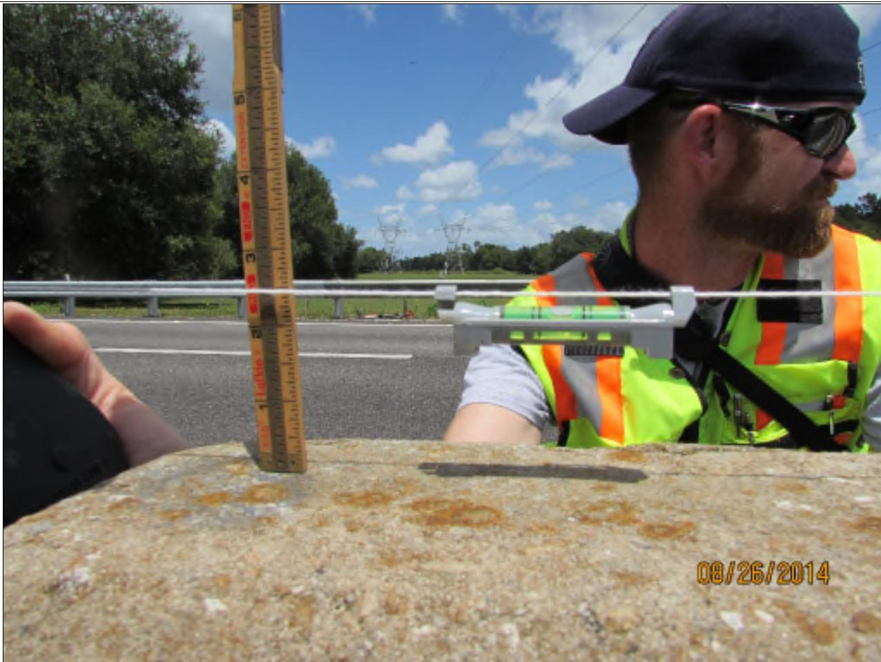
**Photo 2 - Element 331/3 Conc Bridge Railing**
