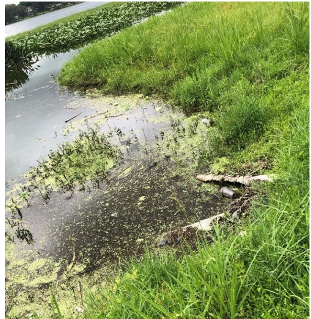
Figure 13: Eroded MES with Outfall to Lake Hunter (August 2020)
