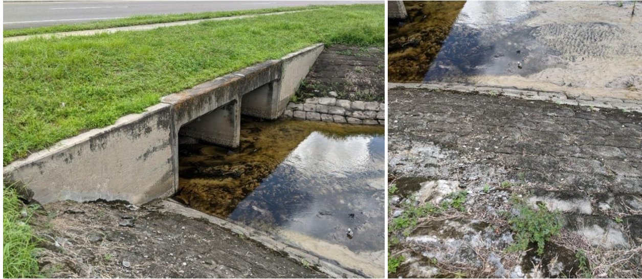
Left image: east end and wingwalls of the concrete box culvert north of the Sikes Blvd. and Ariana St. intersection. Right image: sand-cement rip rap protecting slopes adjacent to the east end of the concrete box culvert.
