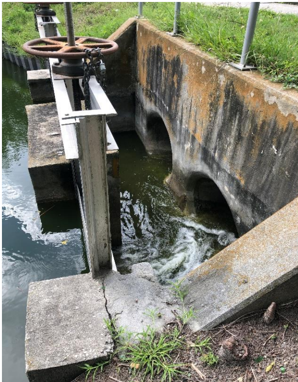
Figure 14. Weir Control Structure for Overflow into Regulatory Floodway
