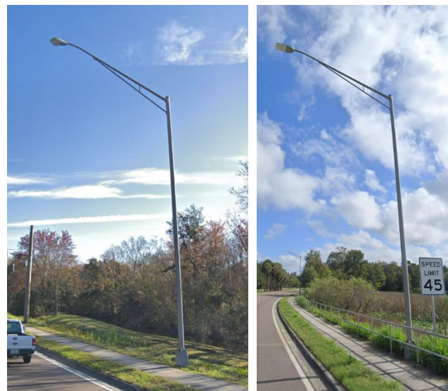
Figure 25: Typical Aluminum Street Lighting Along East Side of Corridor
