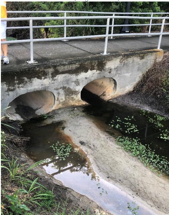
Figure 11. Elliptical Side Drain Permit No. 13139.000 (August 2020)
