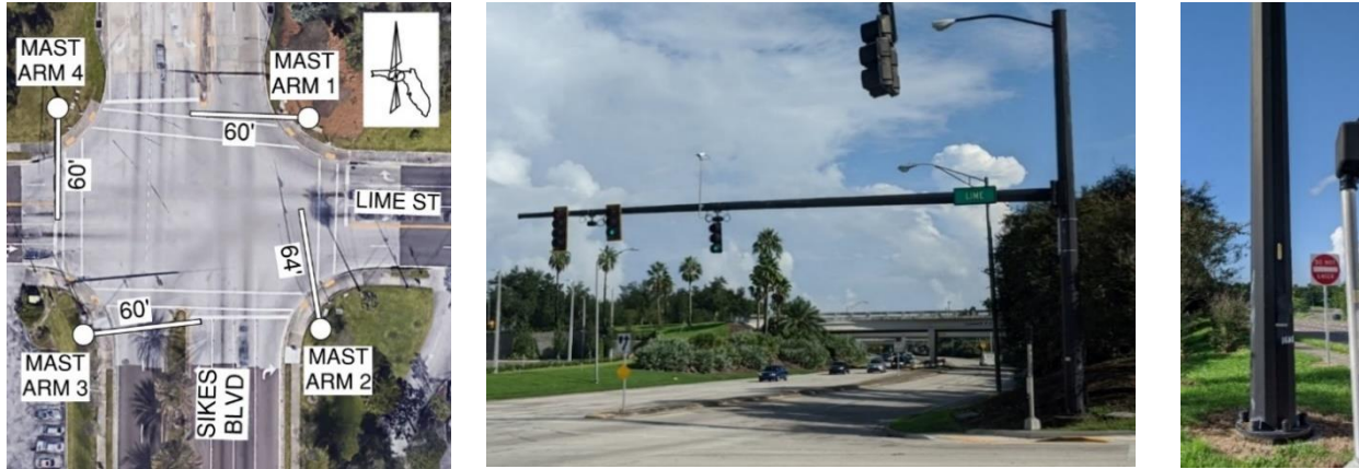
Left image: aerial showing mast arm locations and lengths at the intersection of Sikes Blvd. and Lime St. Middle image: Mast Arm 1. Right image: the upright of Mast Arm 2.
