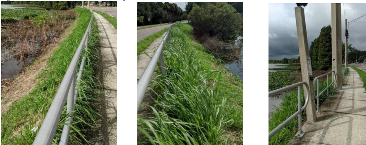
Left image: view from 100' north of the Hartsell intersection, looking south along the Lake Hunter bank. Middle image: view from 100' north of the Hartsell intersection, looking north along the Lake Hunter bank. Right image: pedestrian signal pole listing toward Lake Hunter.
