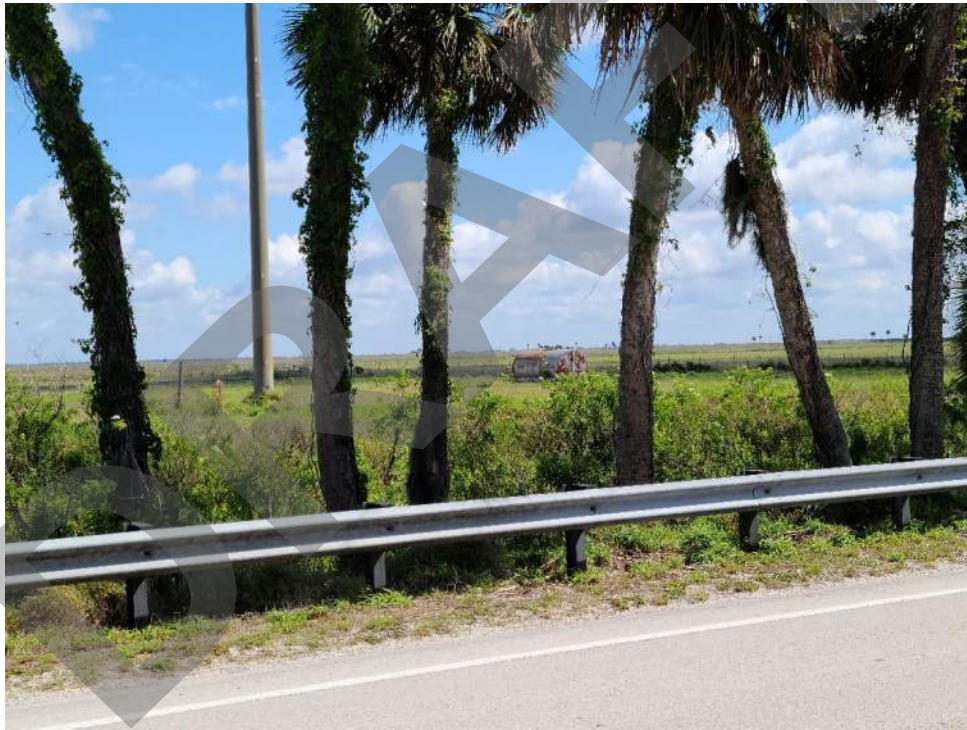
Site 11 – AST SR 70 looking northeast
