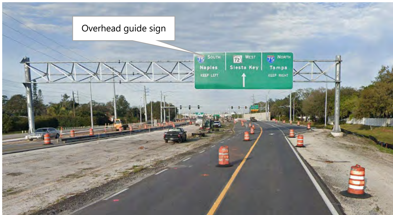
Figure 24: Overhead Guide Sign on SR 72 (looking west) (Source: Google Earth)
