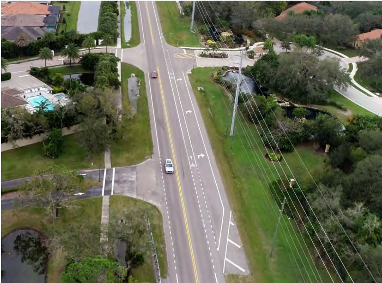
Figure 10: Keyhole Bike Lane on SR 72 (looking east)
