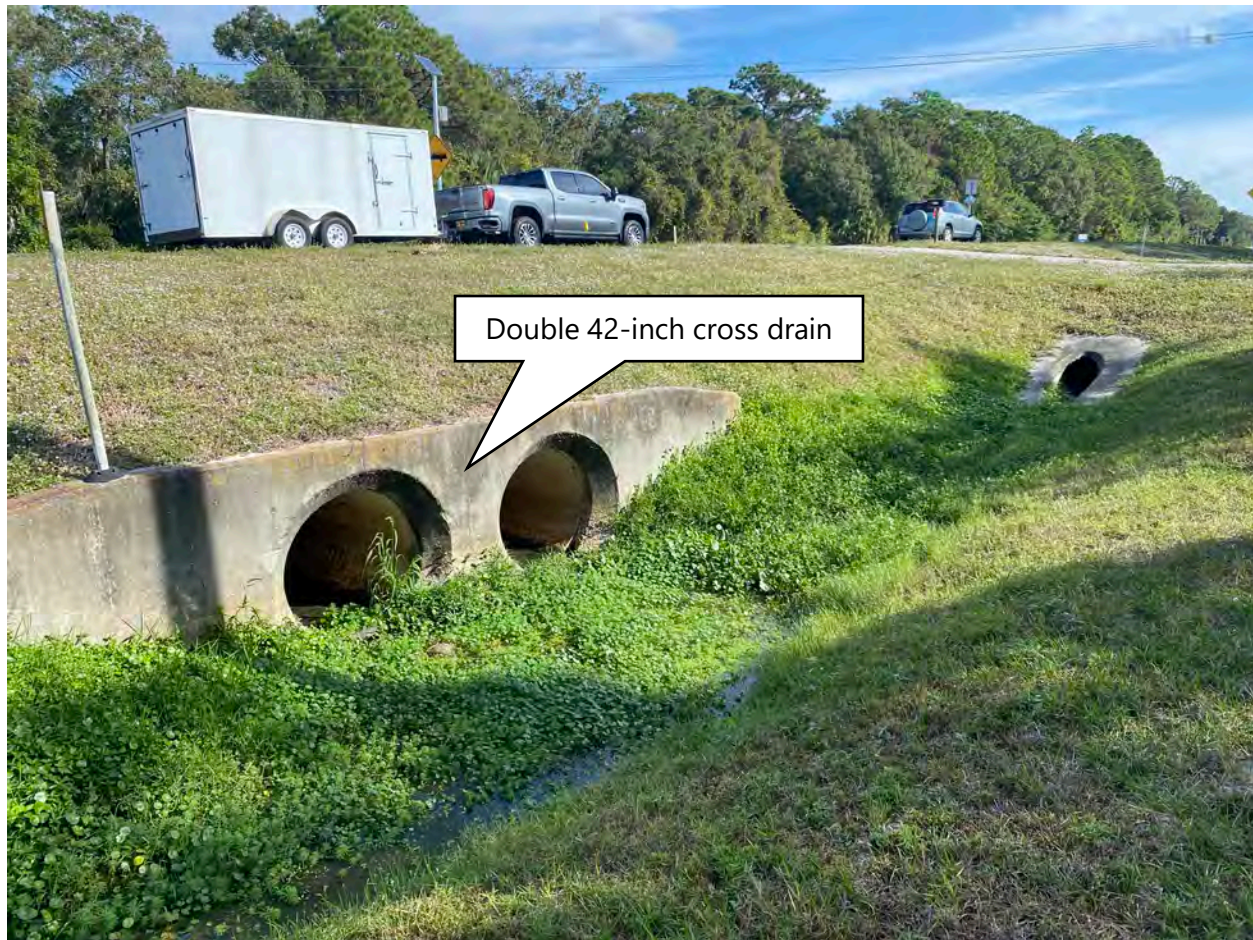
Figure 16: Cross Drain at MP 5.205 SR 72 (looking northeast)
