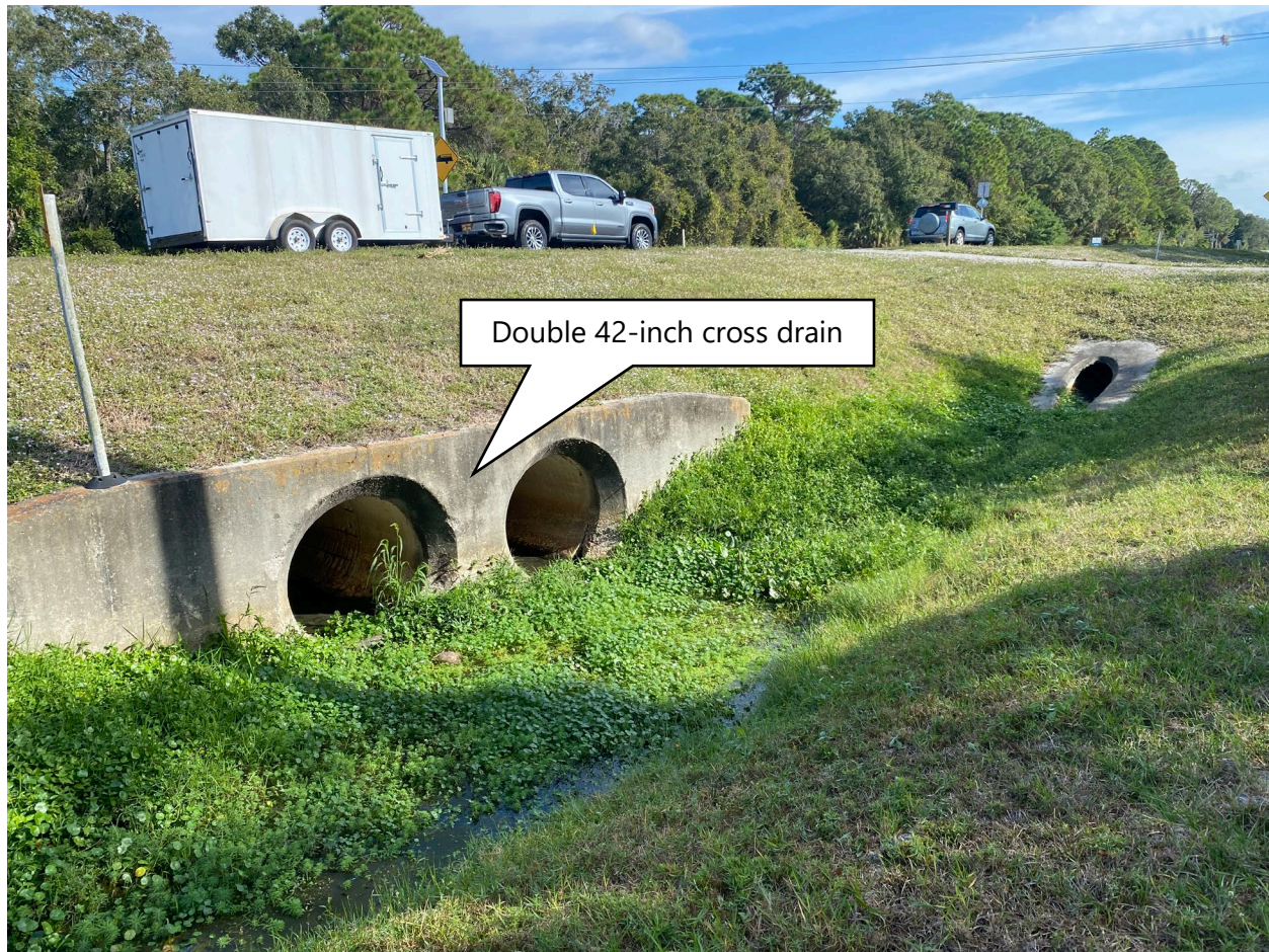
Figure 16: Cross Drain at MP 5.205 SR 72 (looking northeast)
