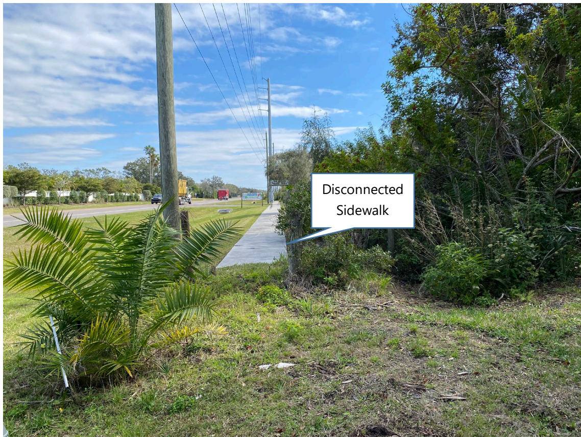
Figure 8: Disconnected Sidewalk along SR 72 (looking east)
