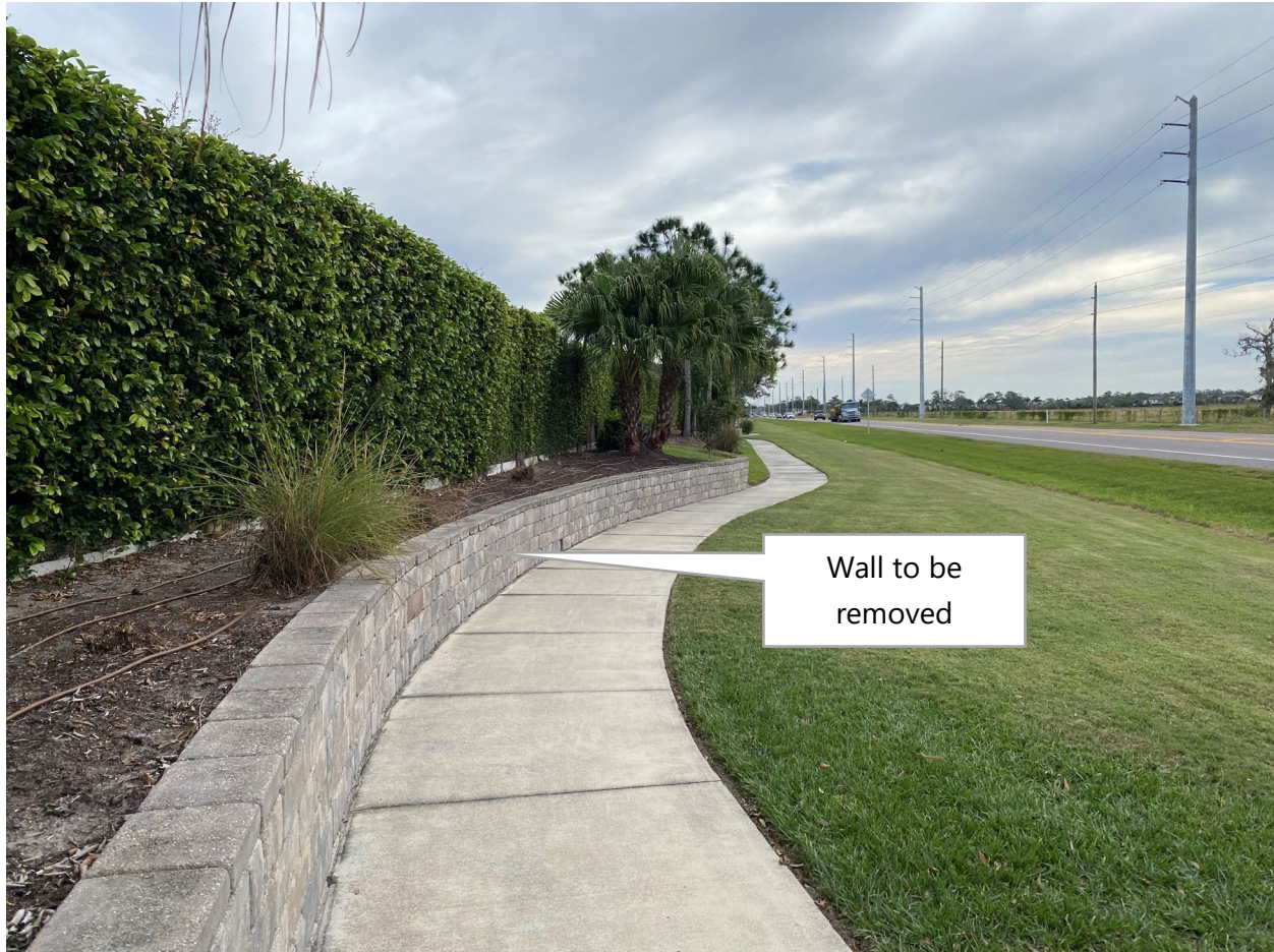
Figure 40: Wildgrass Subdivision Retaining Wall (looking east)
