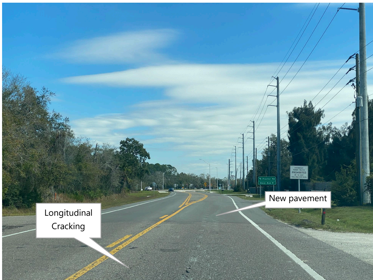
Figure 6: Photo of Pavement Distress on SR 72 (looking east)
