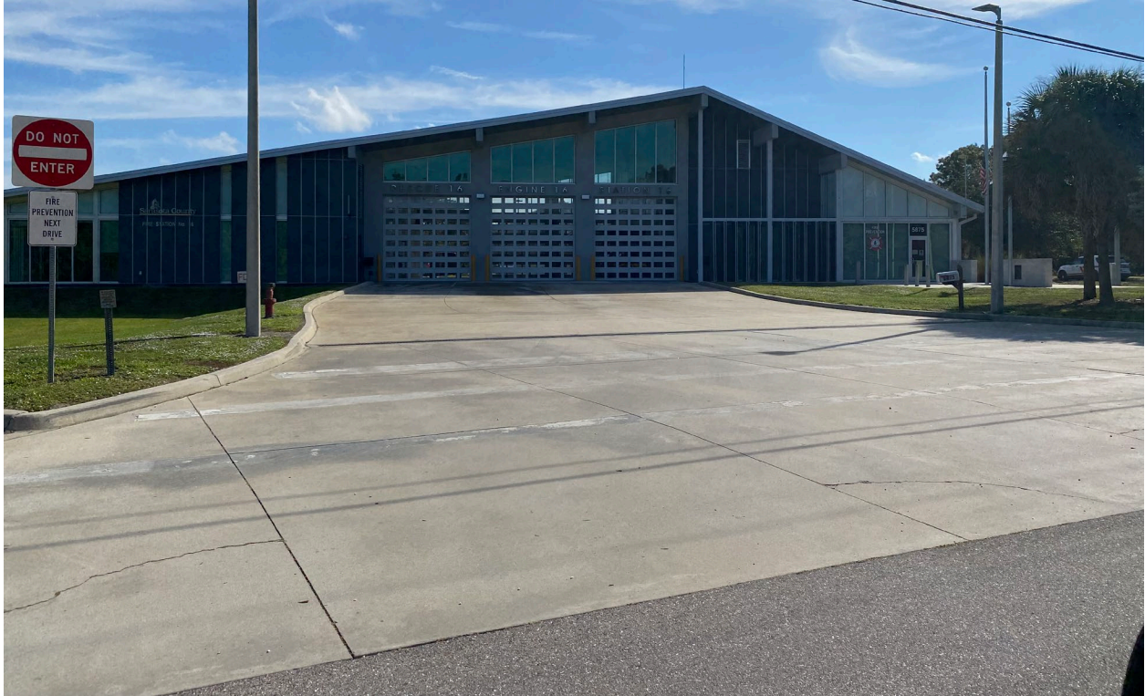
Figure 37: Fire Station 16 (looking east)
