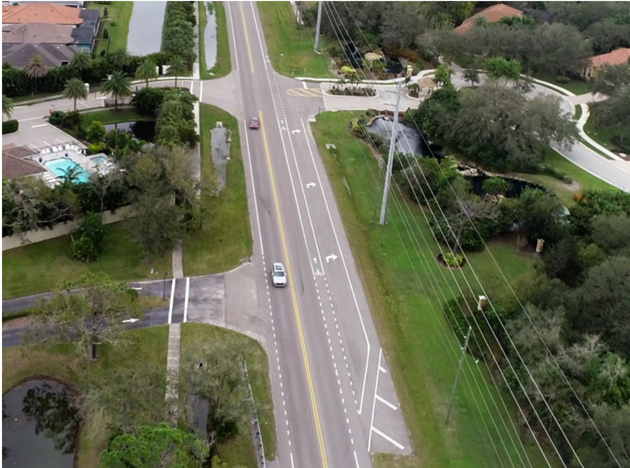
Figure 10: Keyhole Bike Lane on SR 72 (looking east)
