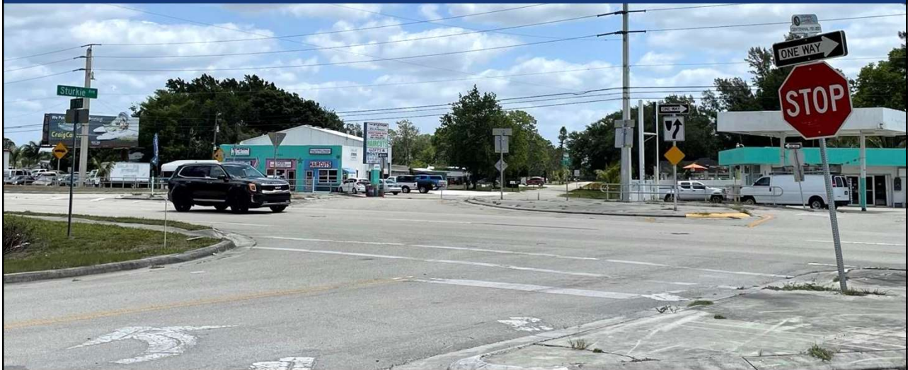
Intersection of SR 776 and Sturkie Avenue | Facing east from Sturkie Avenue
