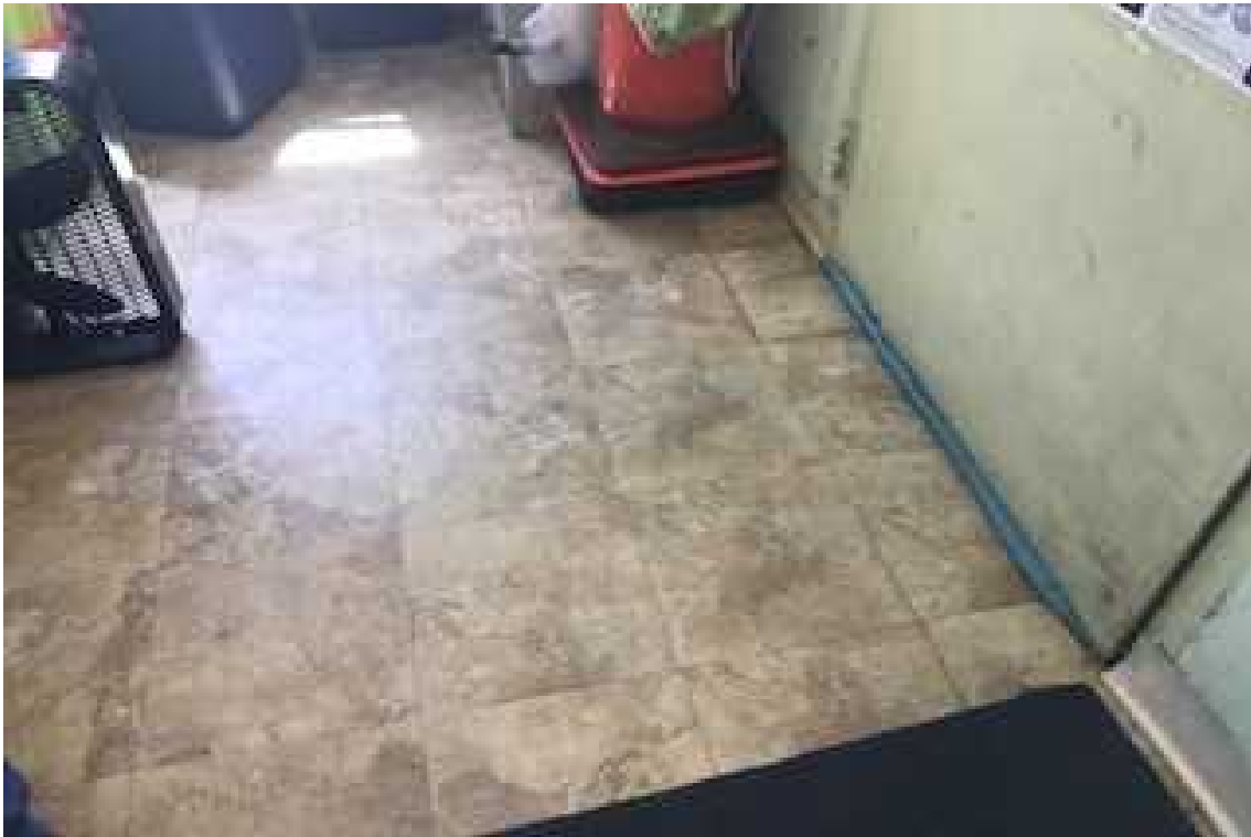
Photo No. 9: Non Asbestos-Containing Floor-Tile
