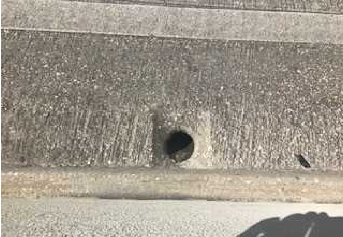
Photo No. 15: Non Asbestos-Containing Metal Scuppers
