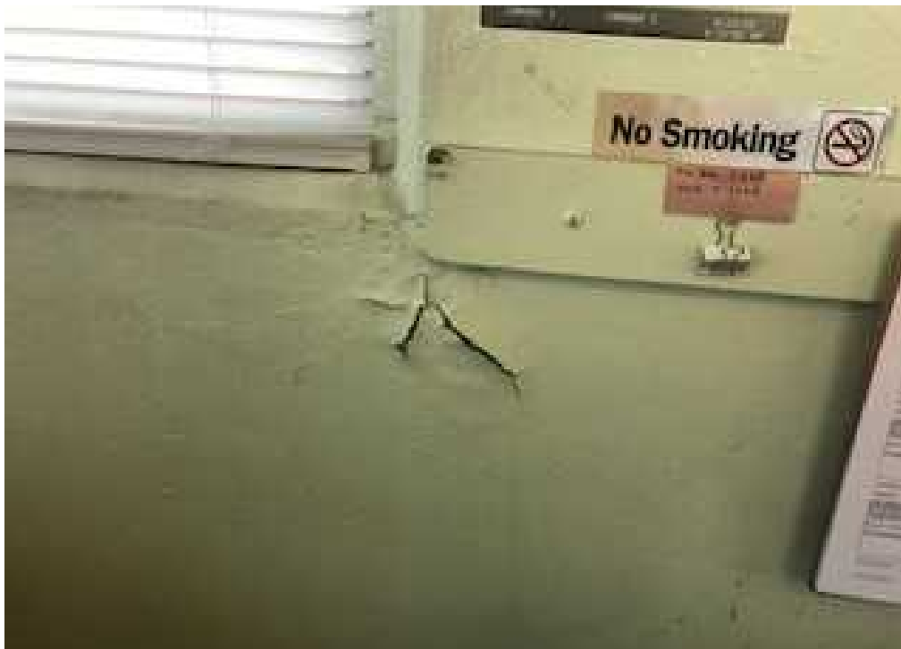
Photo No. 8: Non Asbestos-Containing Interior Wall Paint in Tender House
