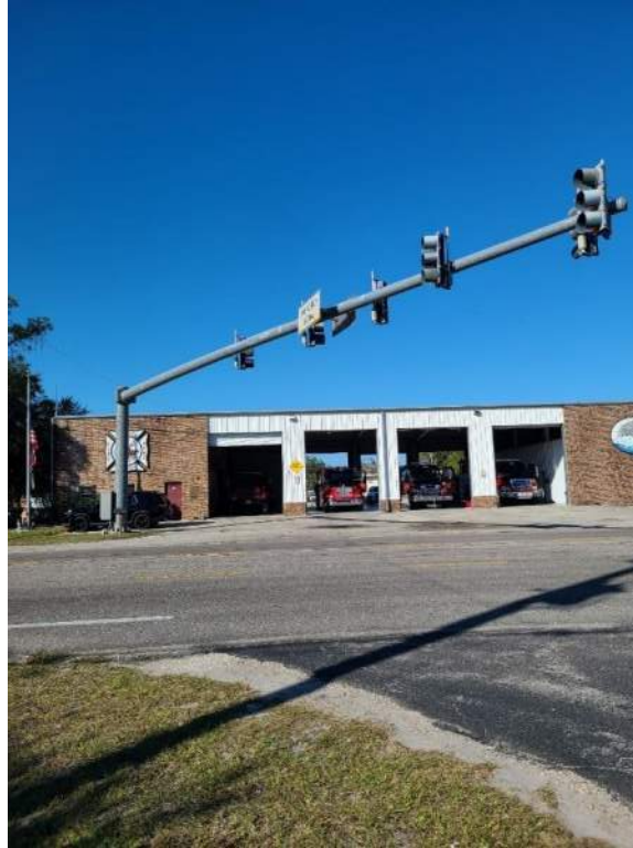
Site 40 – LaBelle City Fire Department Main Street looking west
