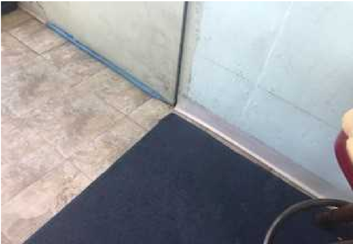
Photo No. 10: Non Asbestos-Containing Baseboard Adhesive
