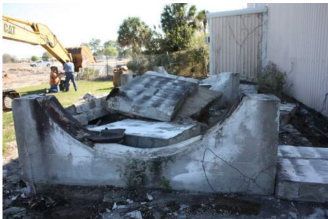
01. TXI- Tank removal1-2/15/2011
