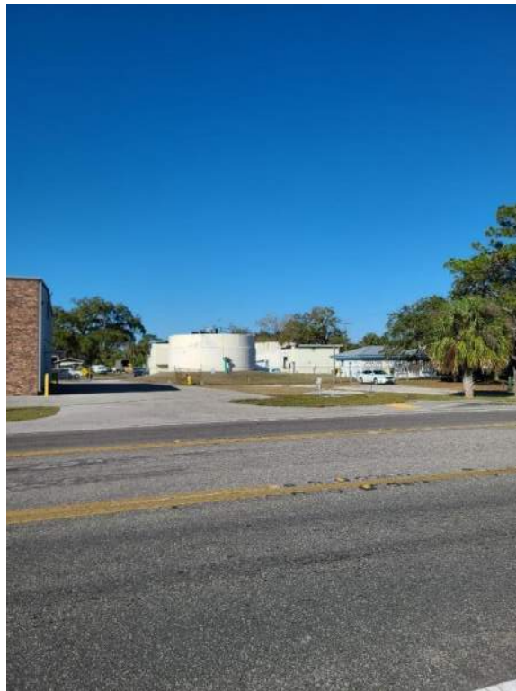
Site 41 – LaBelle Water Treatment Plant #1 / LaBelle City Water Works Main Street looking northwest
