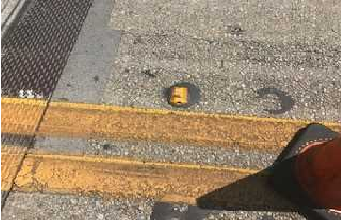
Photo No. 5: Non Asbestos-Containing Reflector Mastic and Yellow Lane Paint
