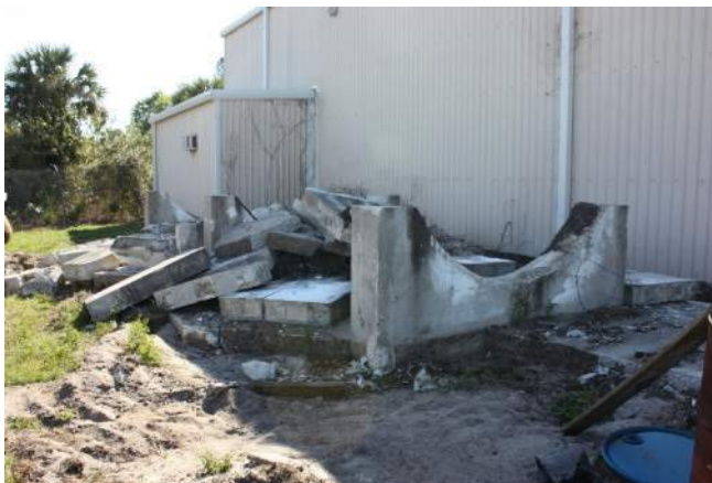
02. TXI- Tank removal2- 7/15/2011
