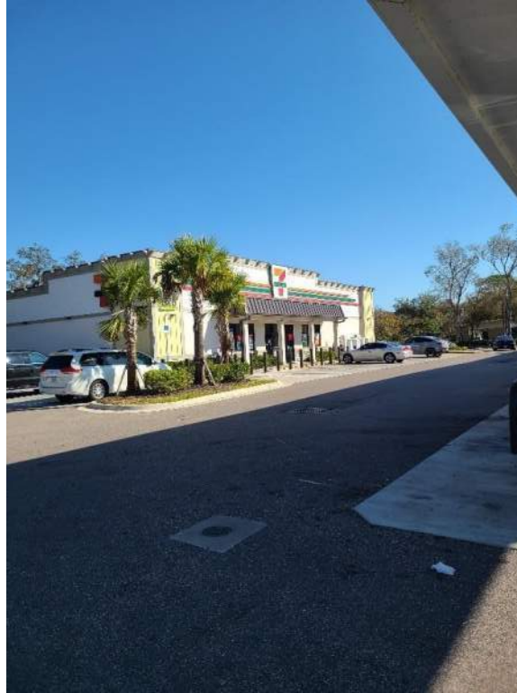
Site N11 – 7-Eleven #41335 Near SR 80 and North Lee Street looking northeast
