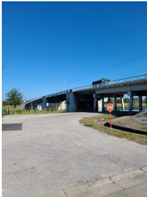
Site N14 – LaBelle Draw Bridge over Caloosahatchee River Near Desoto Avenue looking northeast
