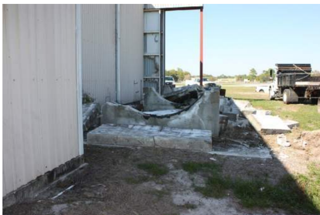
03. TXI- Tank removal3- 2/15/2011
