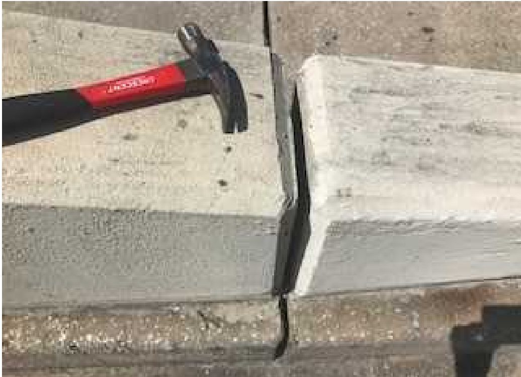
Photo No. 3: Non Asbestos-Containing Concrete Barrier
