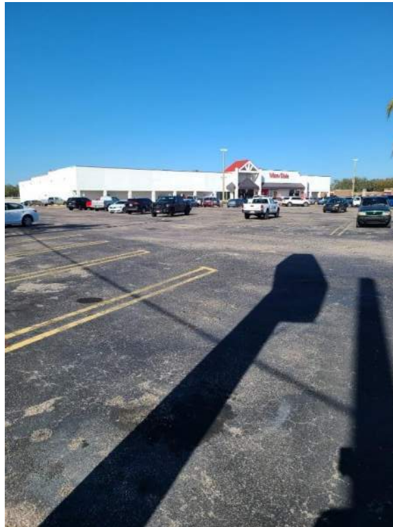
Site 10/11 – Former Alico-Maddox Property and Winn Dixie #721 Near the intersection of Main Street and Cowboy Way looking northwest
