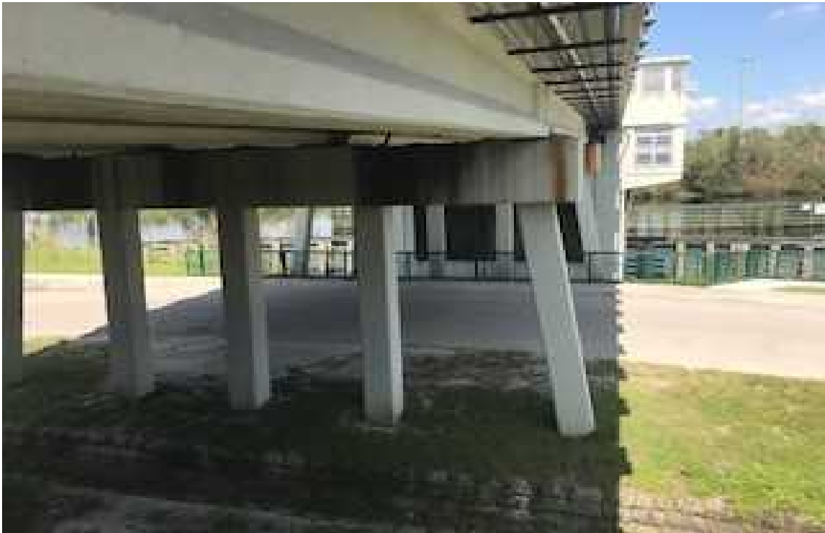
Photo No. 11: Non Asbestos-Containing View of Bridge Structure (Facing North)
