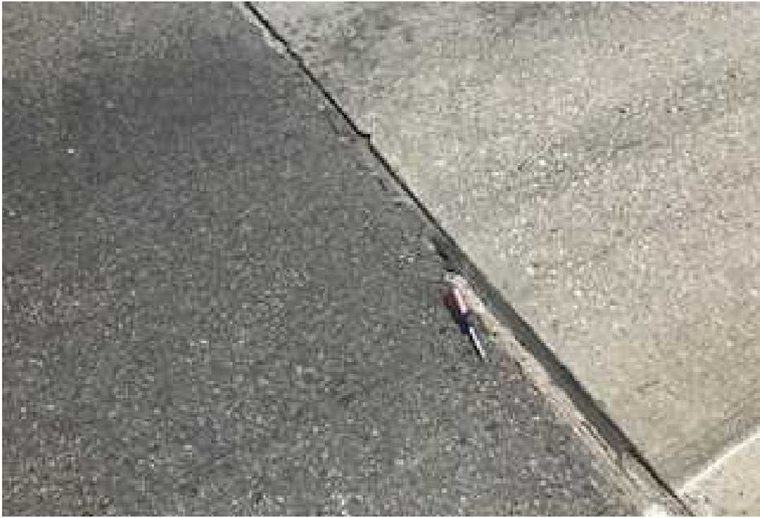
Photo No. 1: Non Asbestos-Containing Asphalt Bridge Approach
