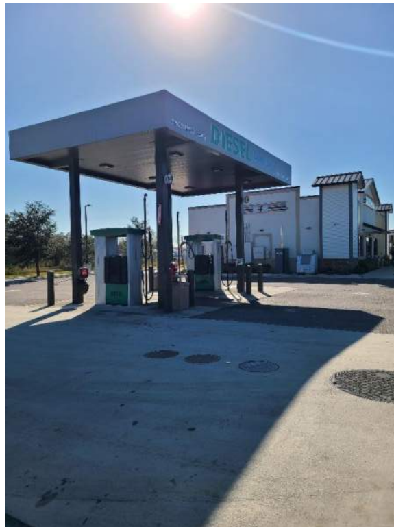
Site N4 – 7-Eleven #41127 Near Main Street looking southeast
