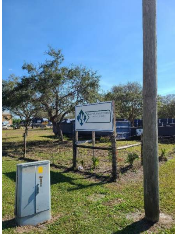
Site 38 – Waste Connections LaBelle / Historic Row Crops SR 29 looking southeast
