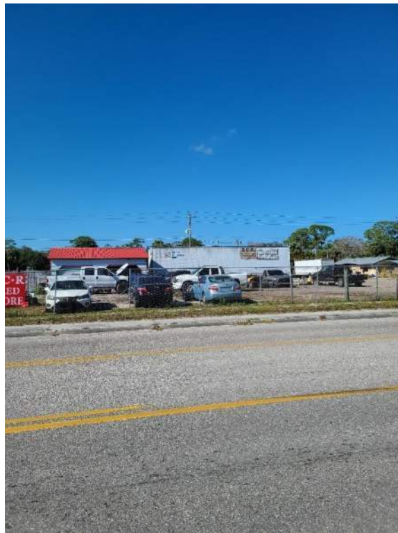
Site 16 – SCR Feedstore / The Shop / J&M Auto Repair Bridge Street looking west
