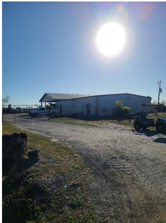
Site N2 – Crews Septic Industrial Loop looking southeast.
