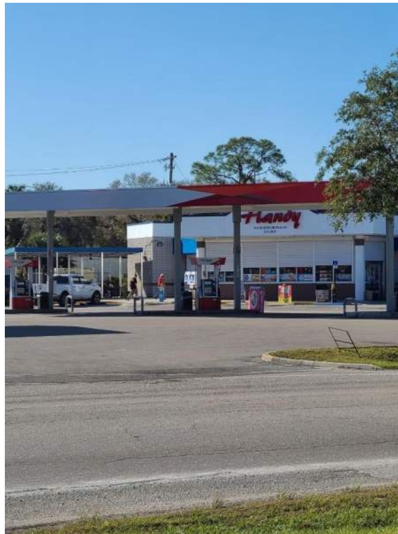
Site 3 – Handy Food Store #58 Near intersection of Cowboy Way and Main Street looking southwest
