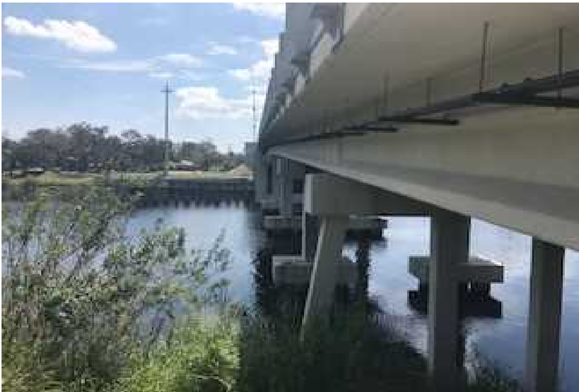
Photo No. 14: Non Asbestos-Containing View of Bridge Structure (Facing South)
