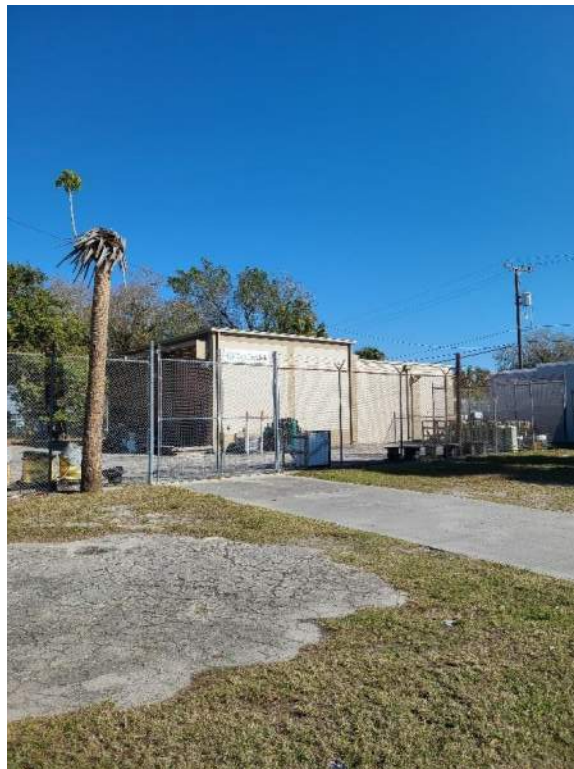
Site N12 – LaBelle Central Cutoff Fort Thompson Avenue looking northeast
