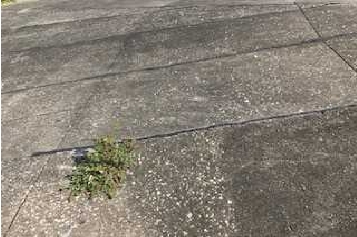
Photo No. 13: Non Asbestos-Containing Embankment Expansion Joints
