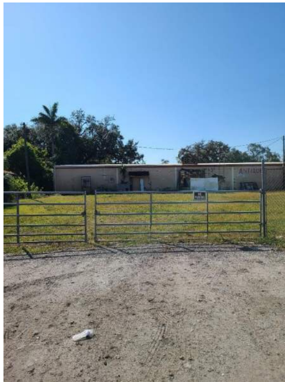
Site 33 – LaBelle Development Co, Inc. Near southeast quadrant of Fort Thompson Avenue and Bridge Street looking south
