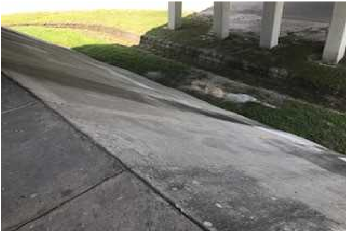
Photo No. 12: Non Asbestos-Containing Embankment Concrete
