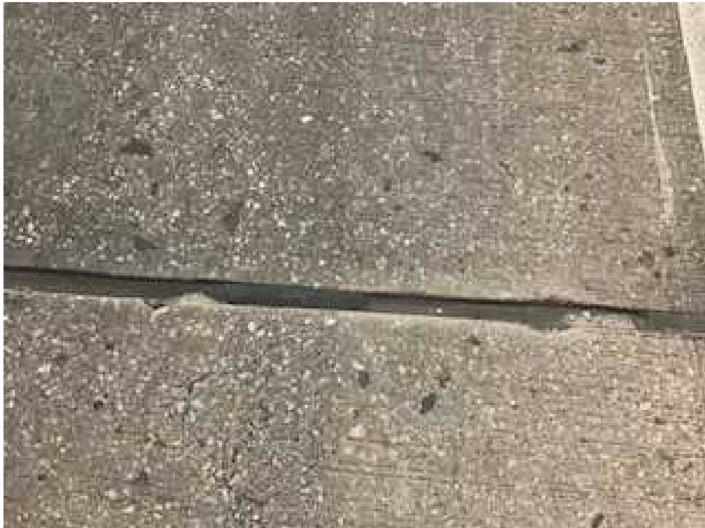
Photo No. 4: Non Asbestos-Containing Expansion Joint
