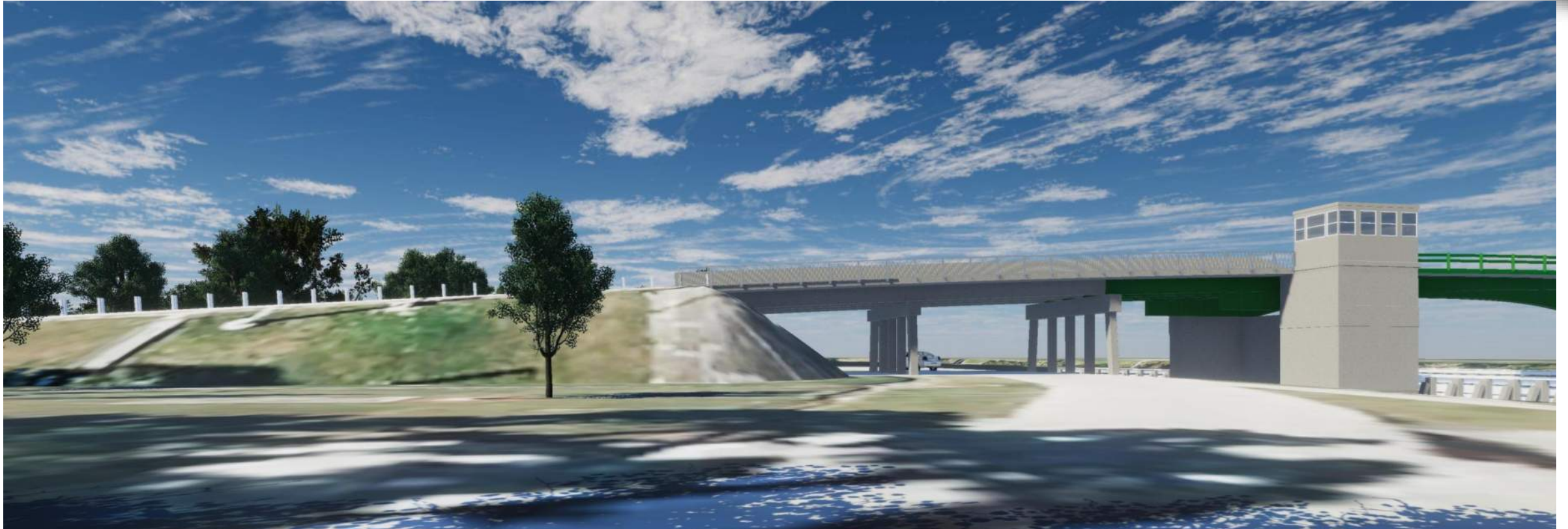
EXISTING BRIDGE LOOKING WEST FROM DESOTO AVE (AT BARRON PARK ENTRANCE)
