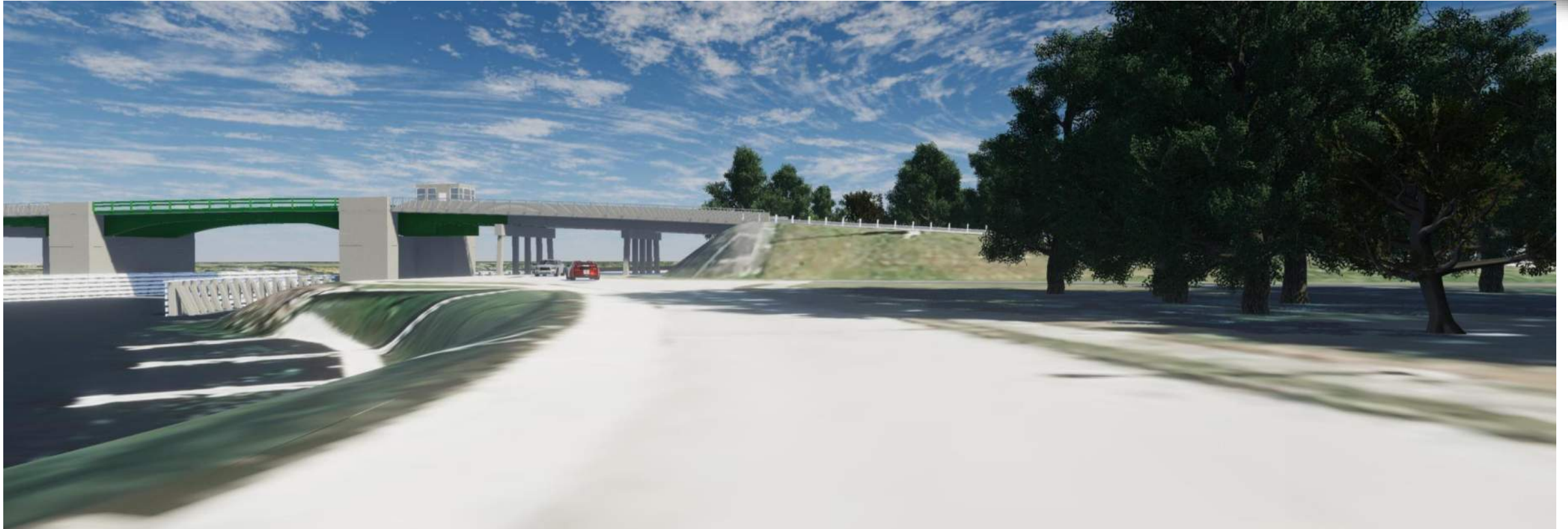
EXISTING BRIDGE LOOKING EAST FROM DESOTO AVE (IN FRONT OF BARRON LIBRARY)
