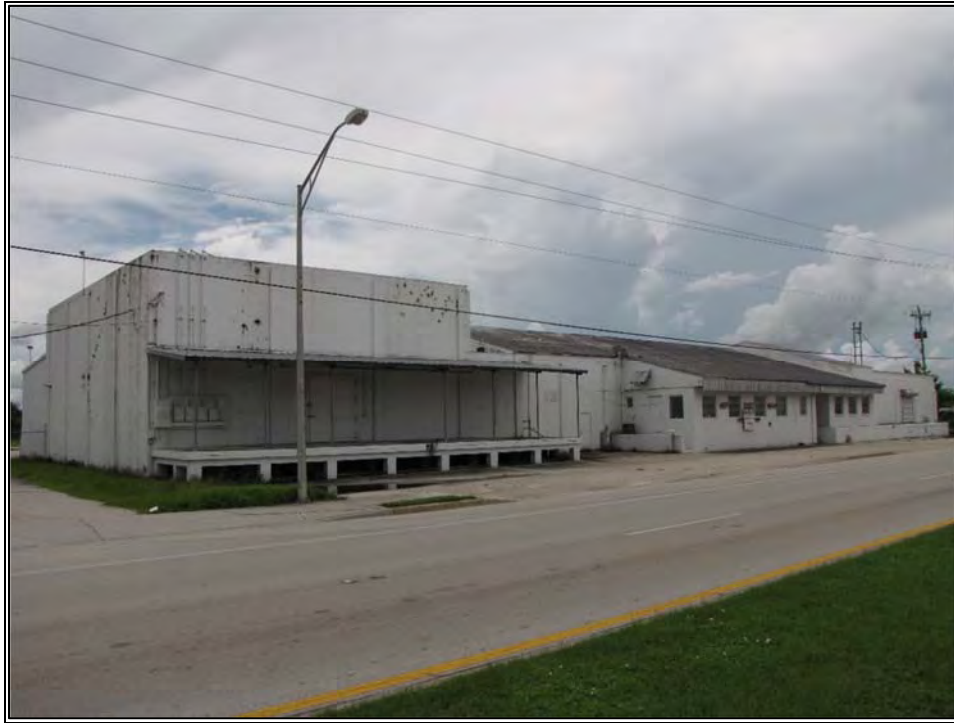
FIGURE 9-21 IMMOKALEE ICE PLANT / 403 E. MAIN STREET (8CR642), FACING SOUTHWEST
