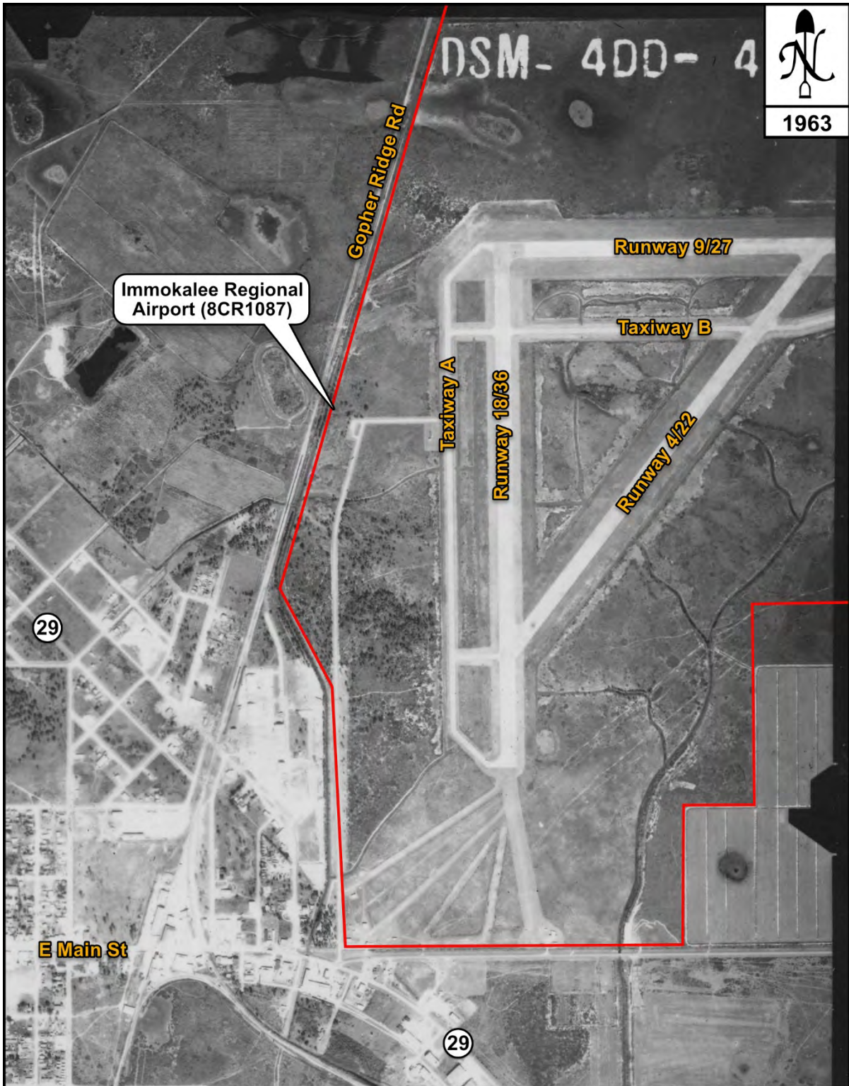
Figure 3: A 1963 Aerial Photograph of the Immokalee Army Air Field/Immokalee Regional Airport (8CR1087)
