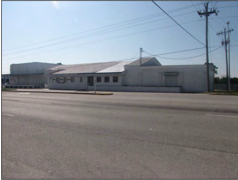
FIGURE 9-22 IMMOKALEE ICE PLANT / 403 E. MAIN STREET (8CR642), FACING SOUTHEAST
