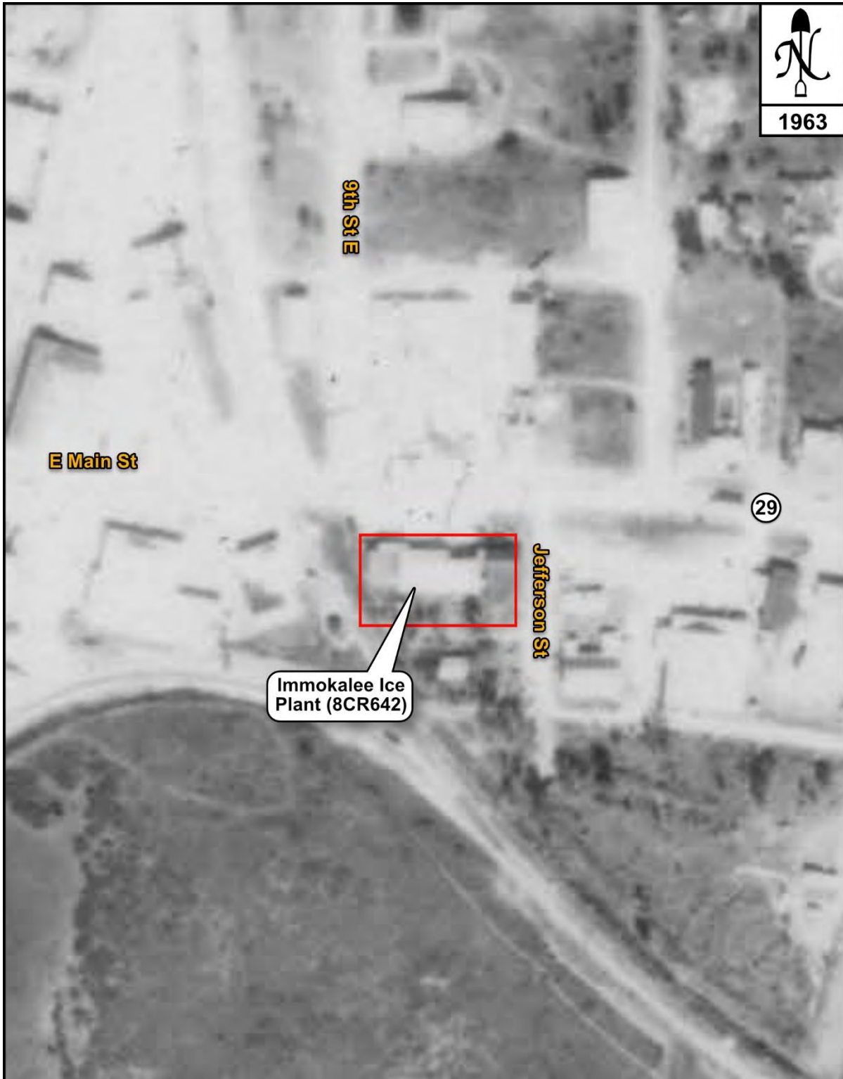
FIGURE 9-24 A HISTORIC 1963 AERIAL PHOTOGRAPH, SHOWING THE WESTERNMOST GABLE-ROOFED ADDITION HAVING BEEN ADDED BETWEEN 1953 AND 1963
