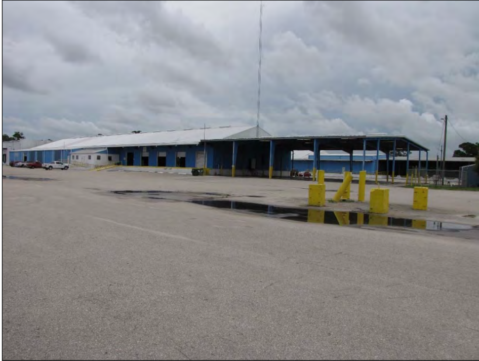
FIGURE 9-34 IMMOKALEE STATE FARMERS MARKET (8CR1500), BUILDING 10, C. 1966, FACING NORTHEAST
