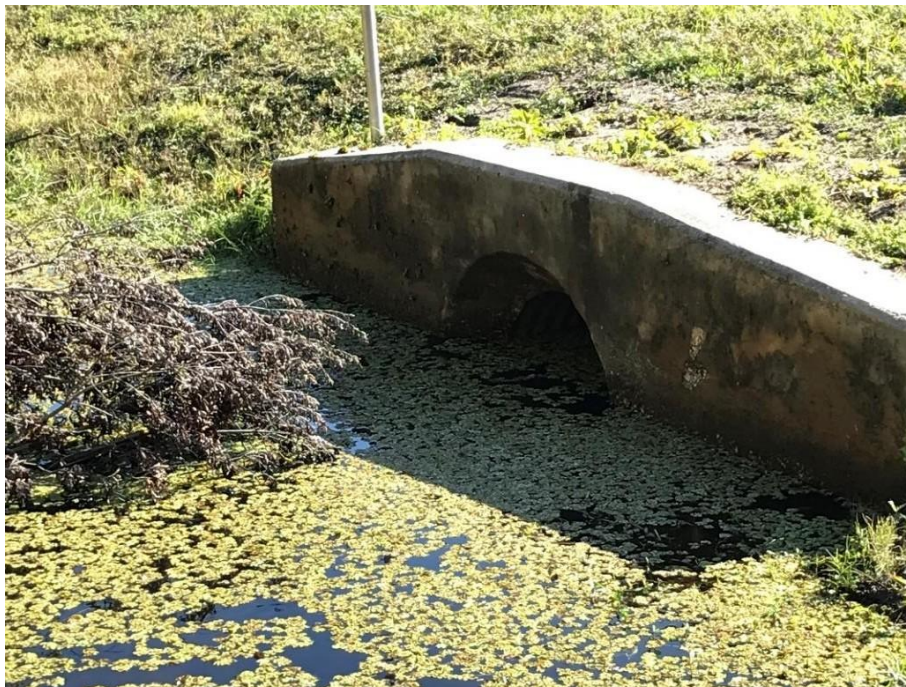
Figure 6 - EX-2 (Existing 30-inch RCP)(12/18/2017)
