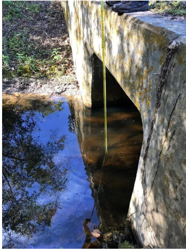
Figure 5 - EX-1 (Existing 4' x 5' CBC) (1/9/2018)
