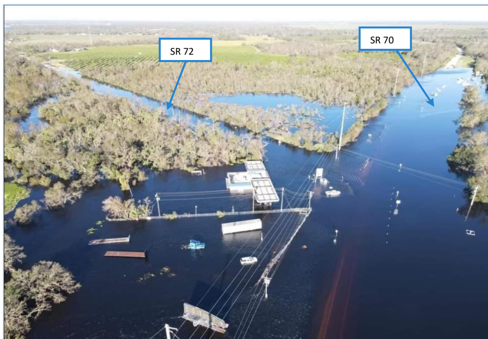
Figure 9 - Hurricane Ian Flooding of SR 70 and SR 72
