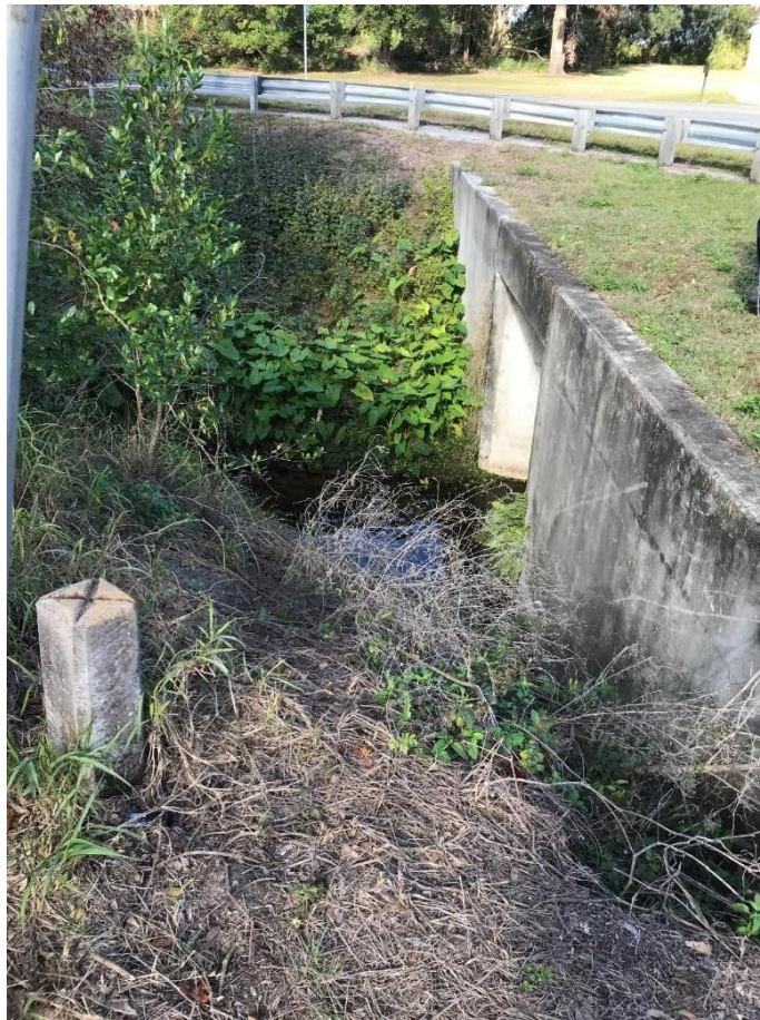
Figure 4- EX-0 (Existing 8'x 8' CBC) (12/18/2017)
