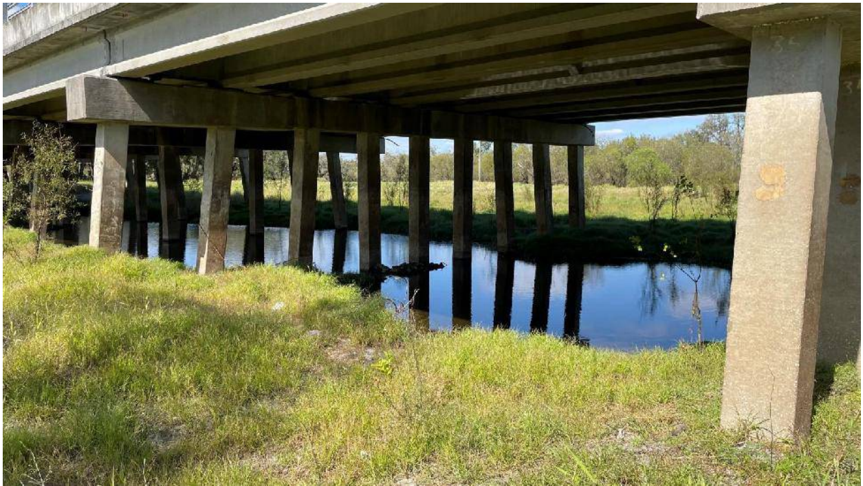
Photo 14 – view northwest from the edge of Wetland 6 under SR 70, the only location where standing water was observed within Wetland 6.
