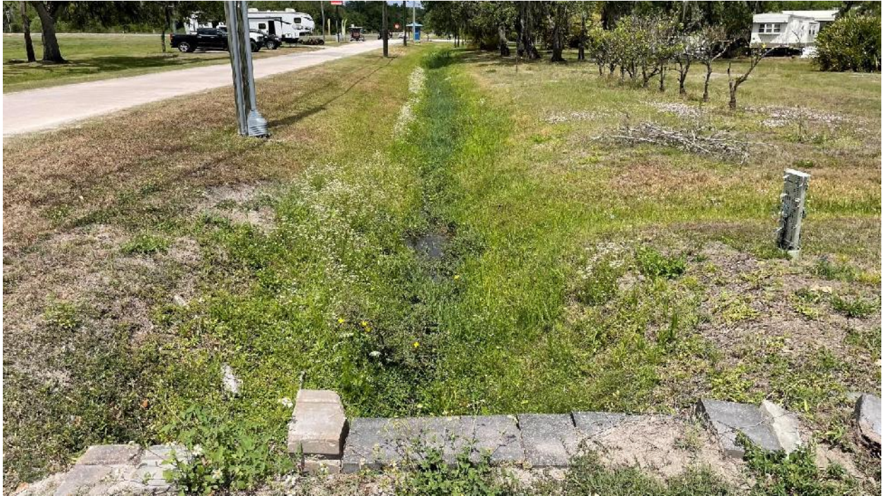
Photo 1 – view west along Surface Water 6 (FLUCCS 5100), an excavated ditch in the northwest portion of the project area. The west portion of the ditch runs through maintained uplands and crosses under roadways via culverts and connects to wetlands west of the project area.
