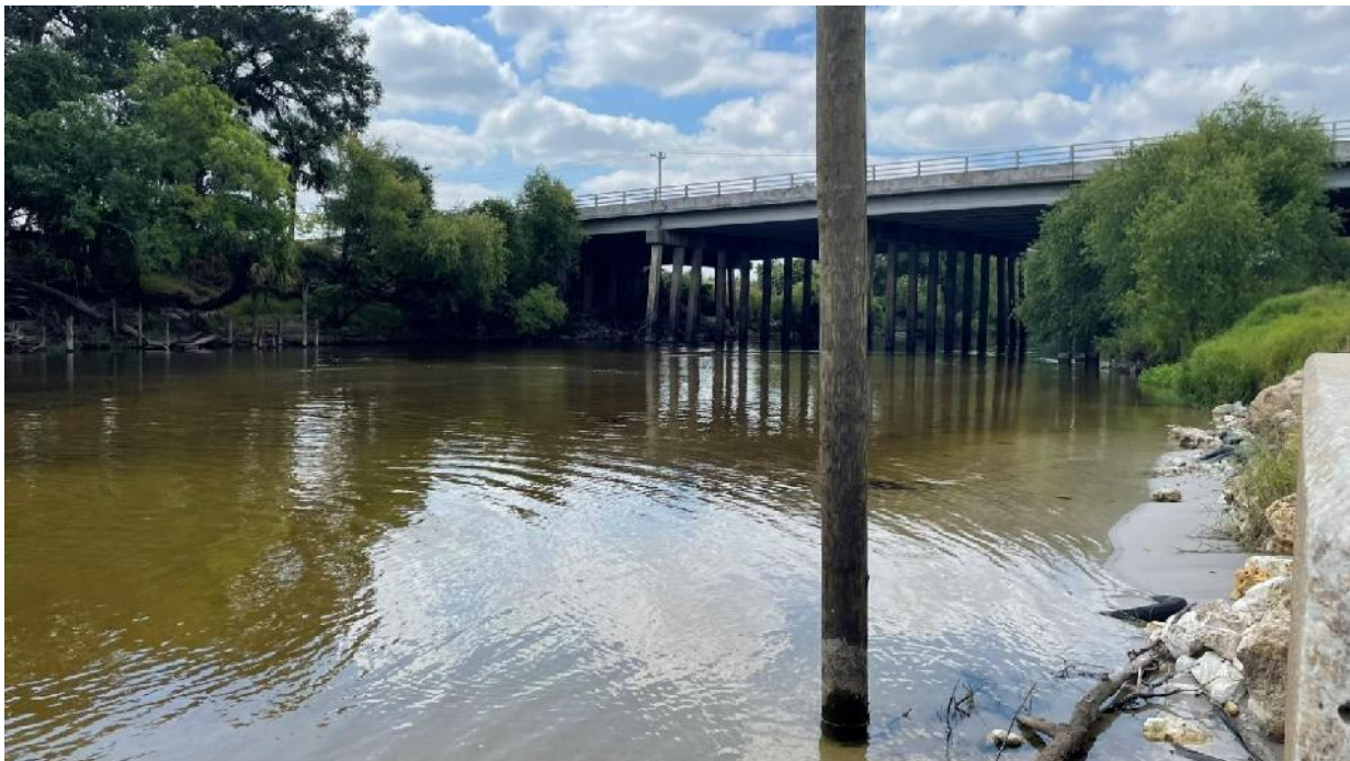
Photo 6 – view south toward the SR 70 bridge crossing the Peace River, Wetland 7 (FLUCCS 5100). The river is shallow and sandy at this location, with banks that are largely altered by previous construction. Portions of the river banks contain trees and shrubs including Brazilian pepper ( Schinus terebinthifolia ), Carolina willow, and buttonbush ( Cephalanthus occidentalis ).
