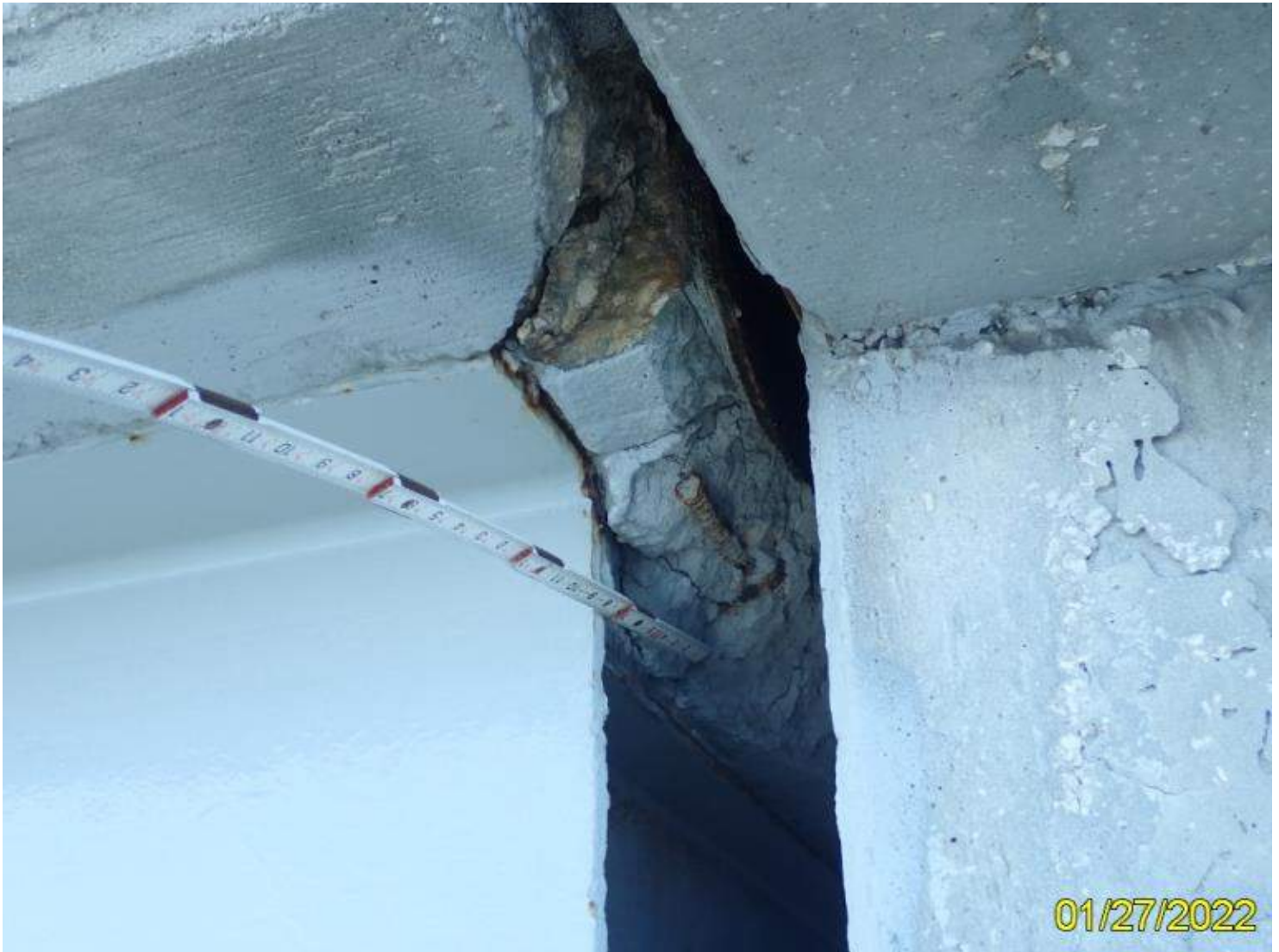
Photo 1 - Element 12 Re Concrete Deck
