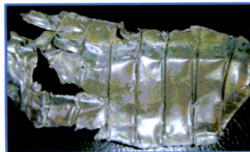
Girder 22-1 Bottom Tendon Duct
