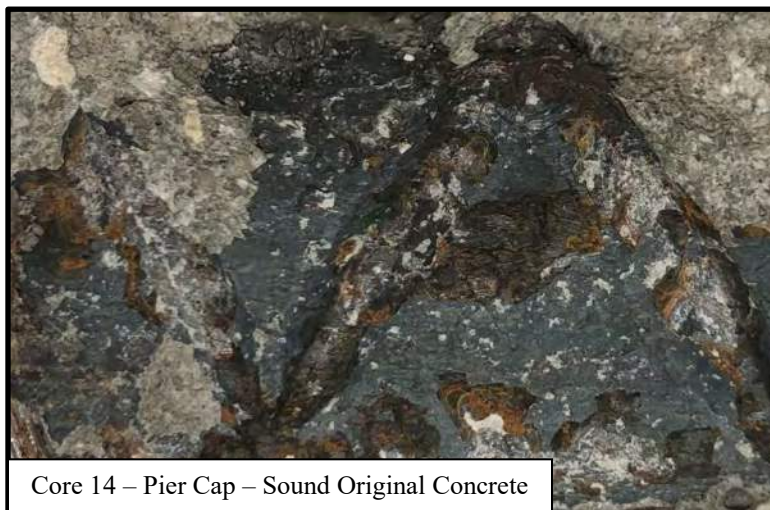
Figure 12. Condition of the reinforcing steel in deck and pier cap.
