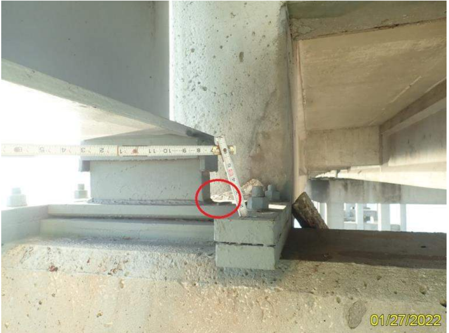
Photo 17 - Element 313 Fixed Bearing (8516 Painted Steel)
