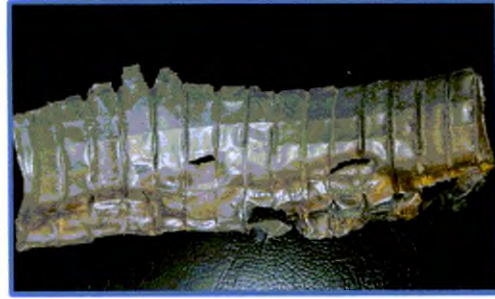
Girder 5-1 Top Tendon Duct
