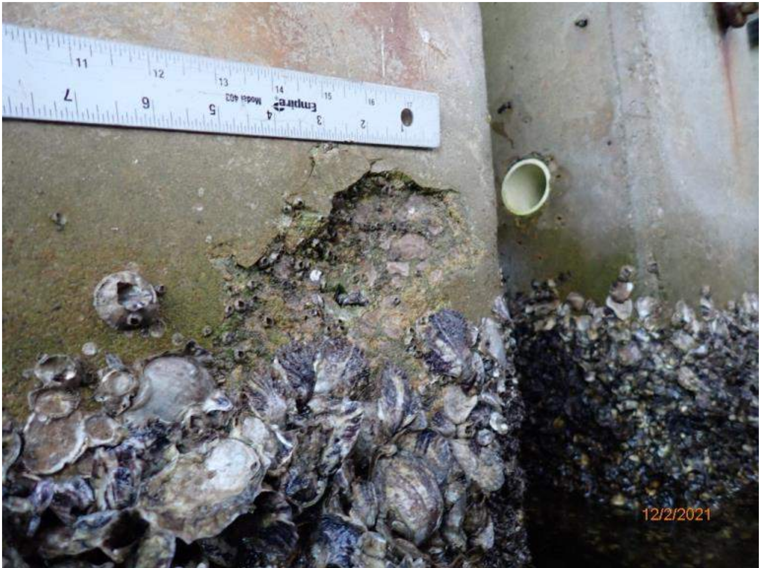
Photo 11 - Element 8387 PS Fender/Dolphin
