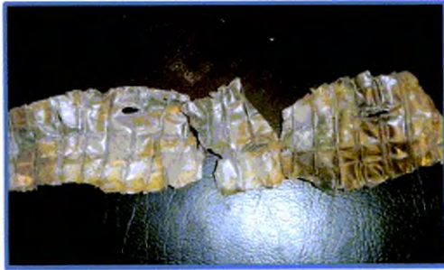
Girder 5-1 Bottom Tendon Duct
