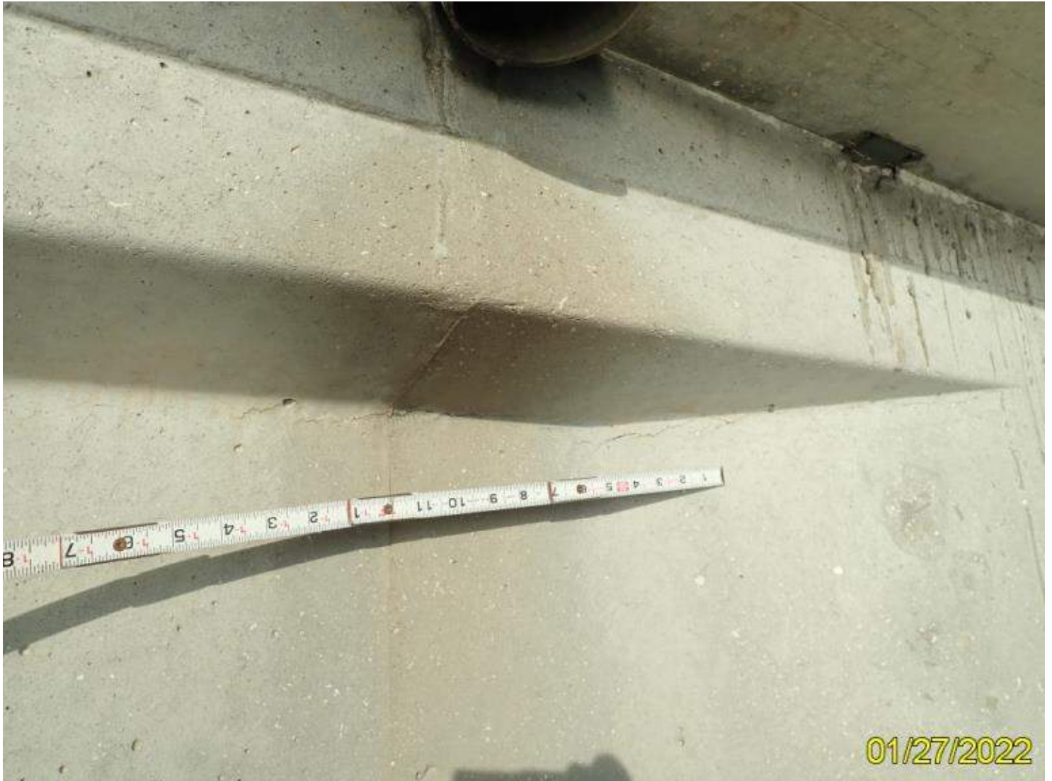
Photo 19 - Element 109 Pre Opn Conc Girder/Beam
