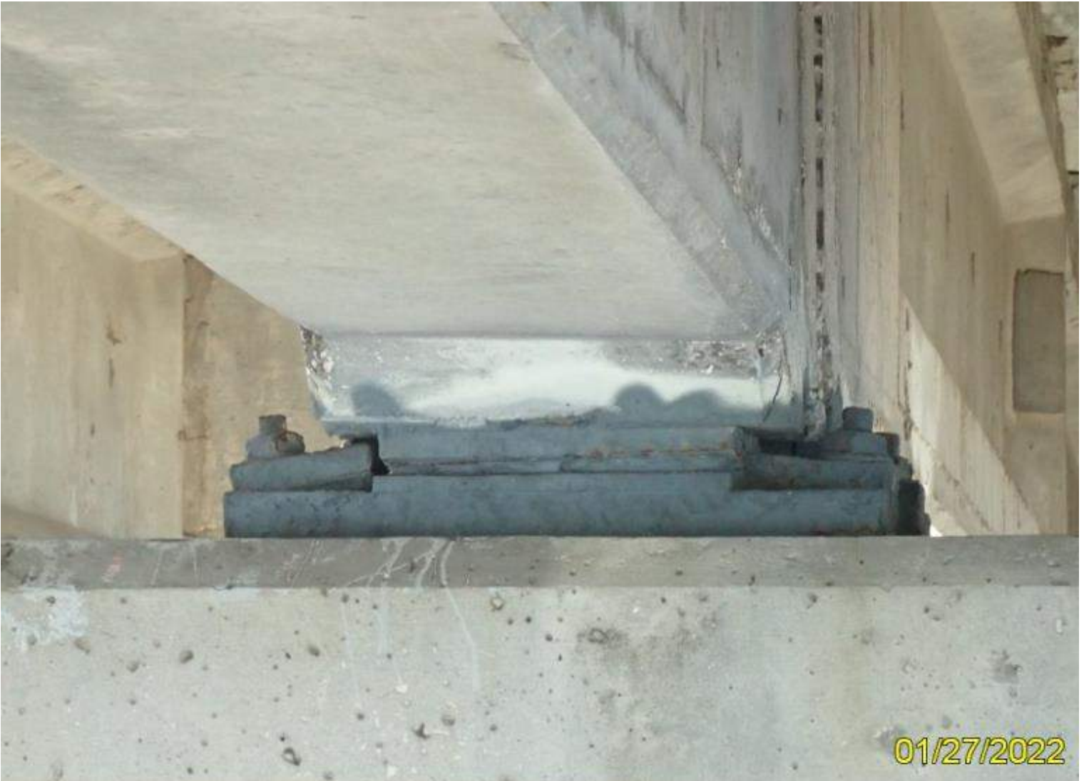
Photo 13 - Element 311 Moveable Bearing (8516 Painted Steel)
