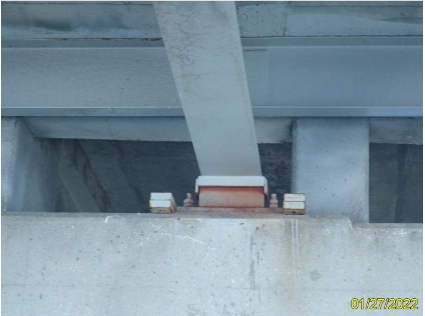
Photo 15 - Element 311 Moveable Bearing (8516 Painted Steel)
