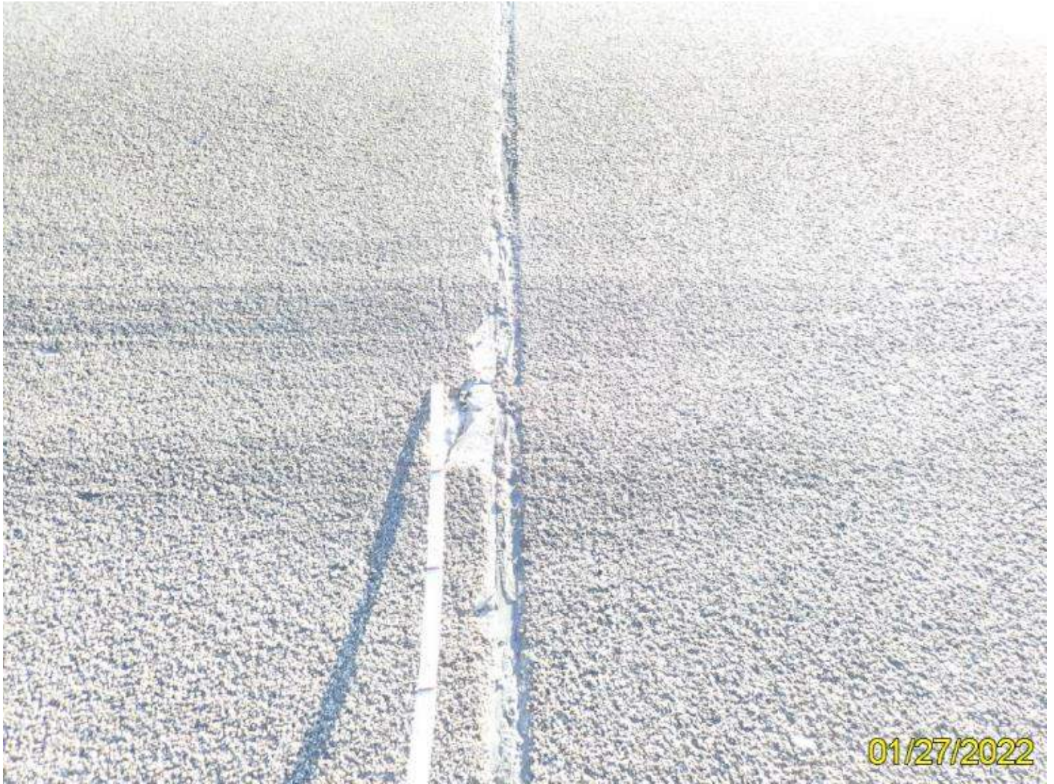
Photo 2 - Element 12 Re Concrete Deck (510 Wearing Surfaces)
