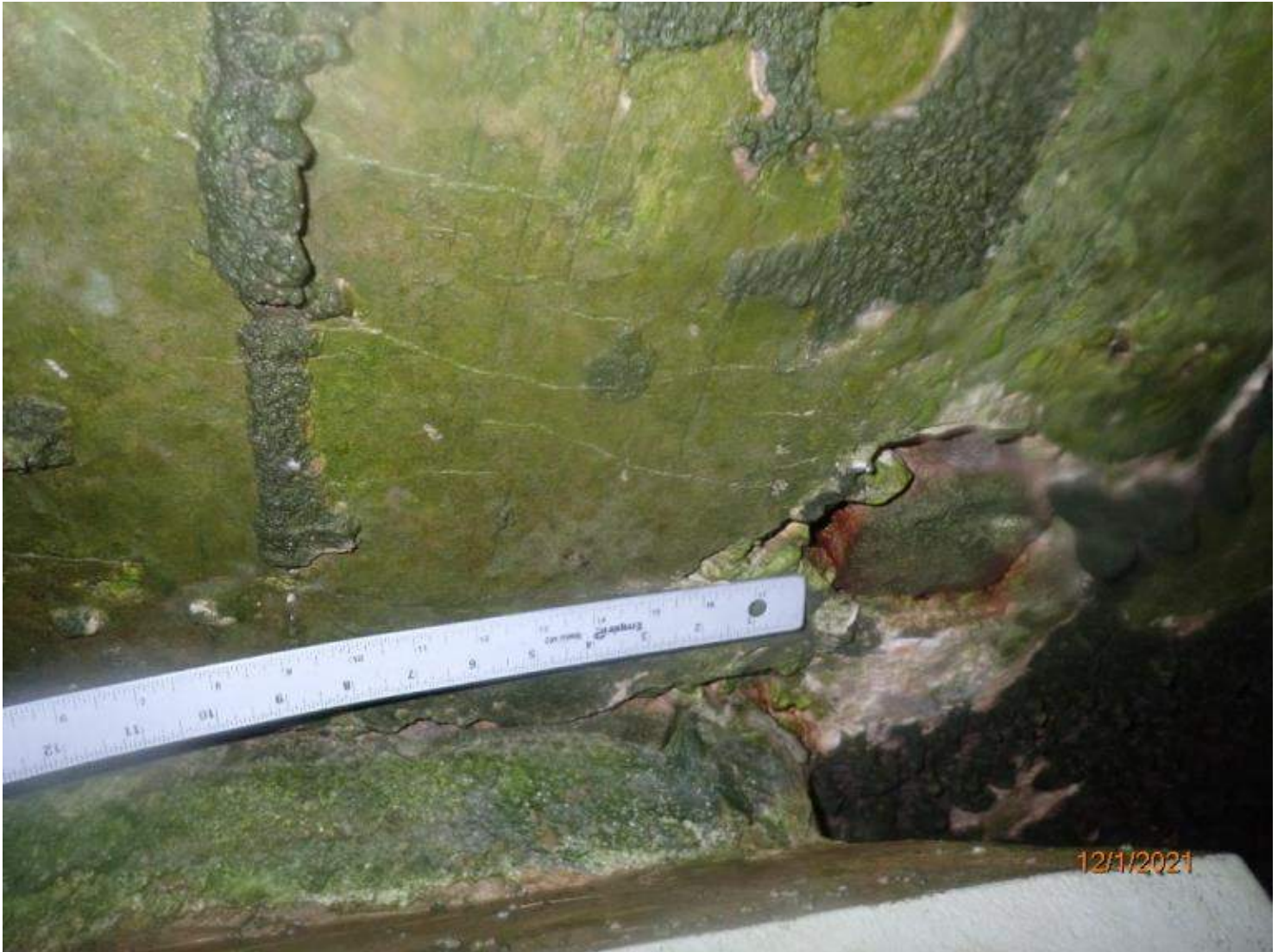
Photo 5 - Element 220 Re Conc Pile Cap/Ftg
