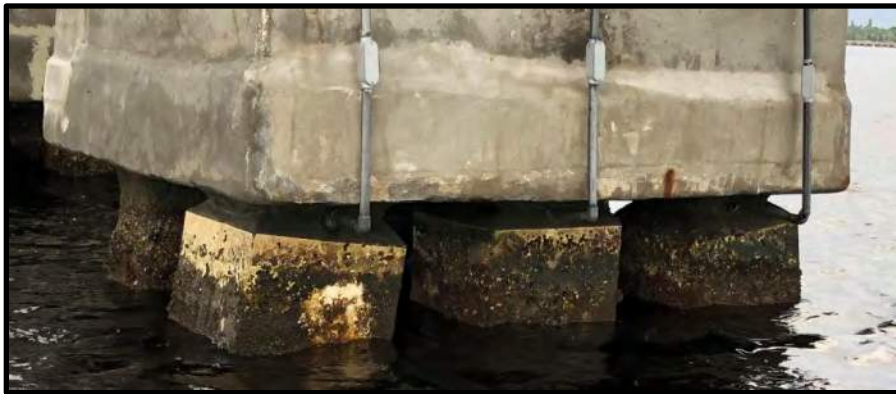
Figure 8. Typical exposed portions of piles at low tide.
