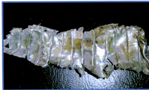
Girder 26-1 Bottom Tendon Duct
