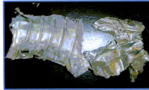
Girder 26-1 Top Tendon Duct
