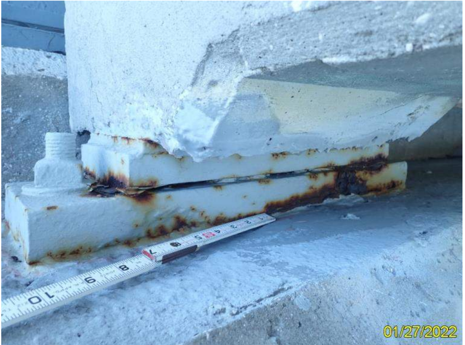
Photo 16 - Element 313 Fixed Bearing (8516 Painted Steel)
