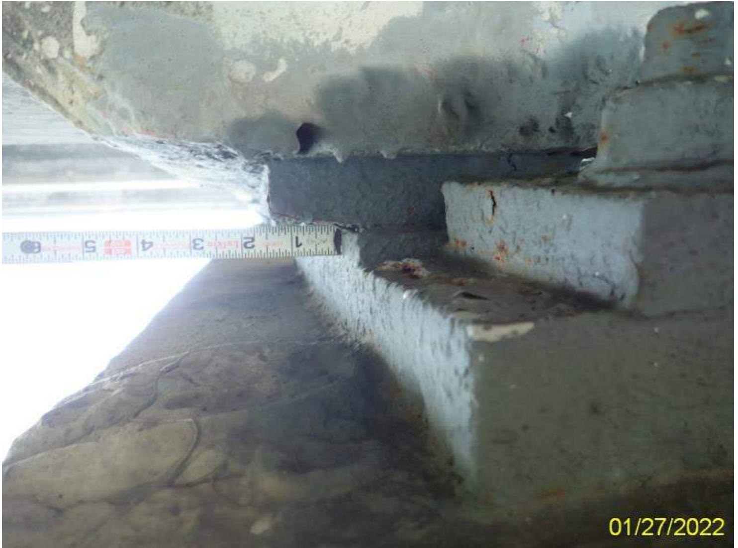
Photo 14 - Element 311 Moveable Bearing
