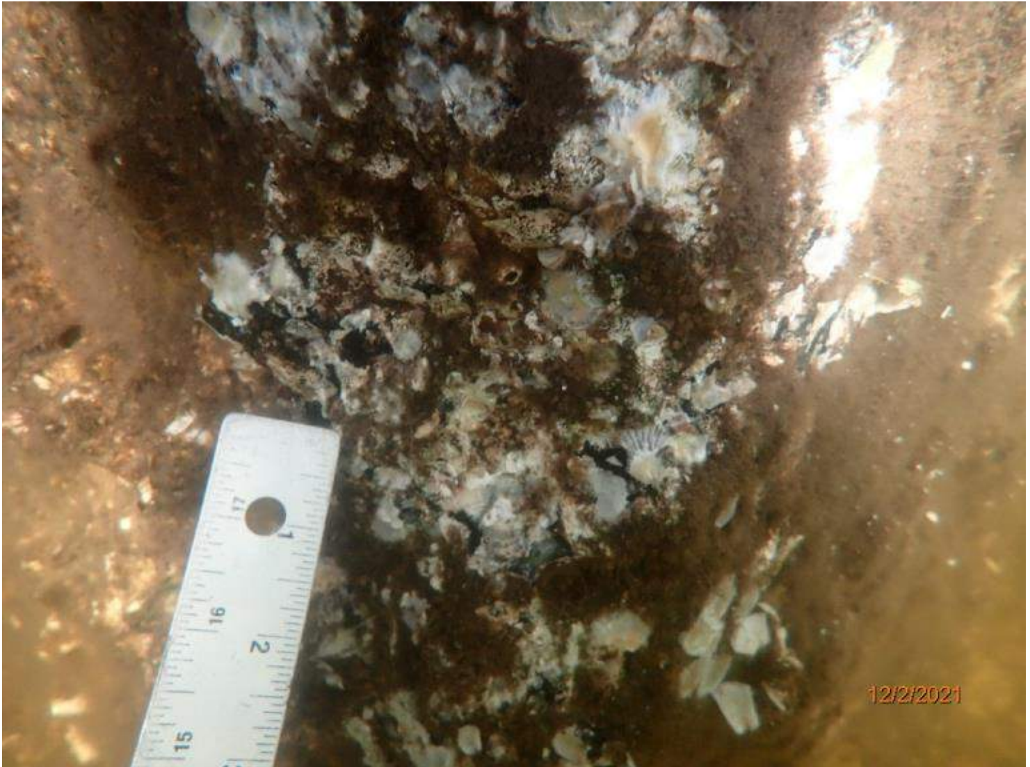
Photo 8 - Element 227 Re Conc Pile
