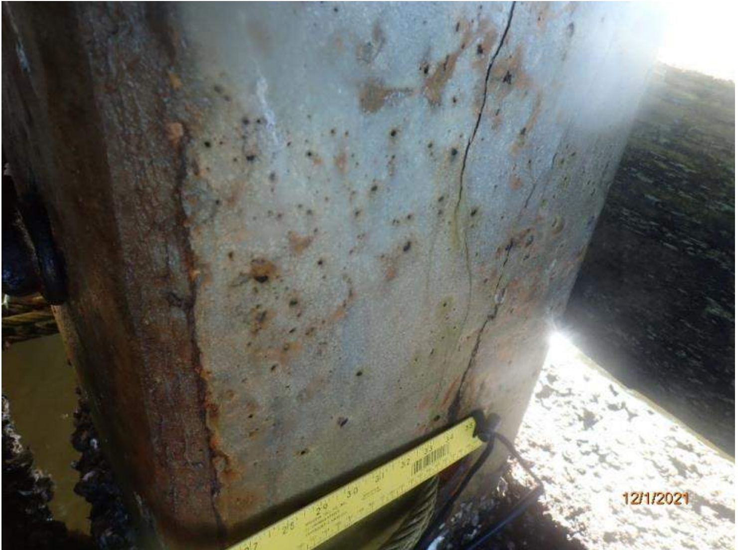
Photo 12 - Element 8387 PS Fender/Dolphin
