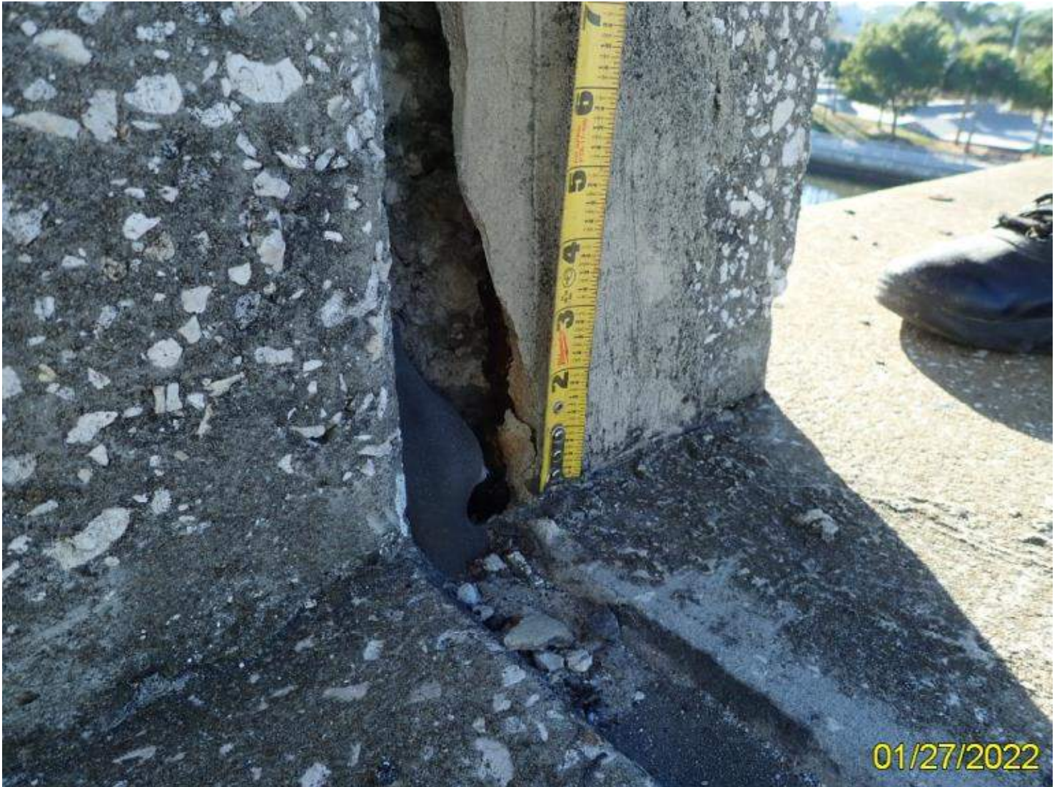
Photo 20 - Element 331 Re Conc Bridge Railing
