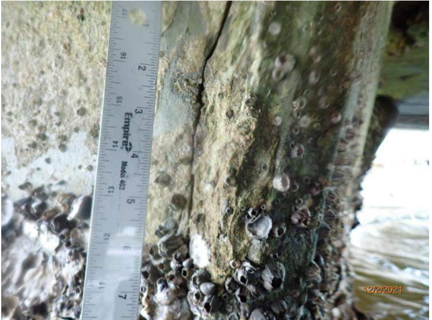
Photo 9 - Element 227 Re Conc Pile
