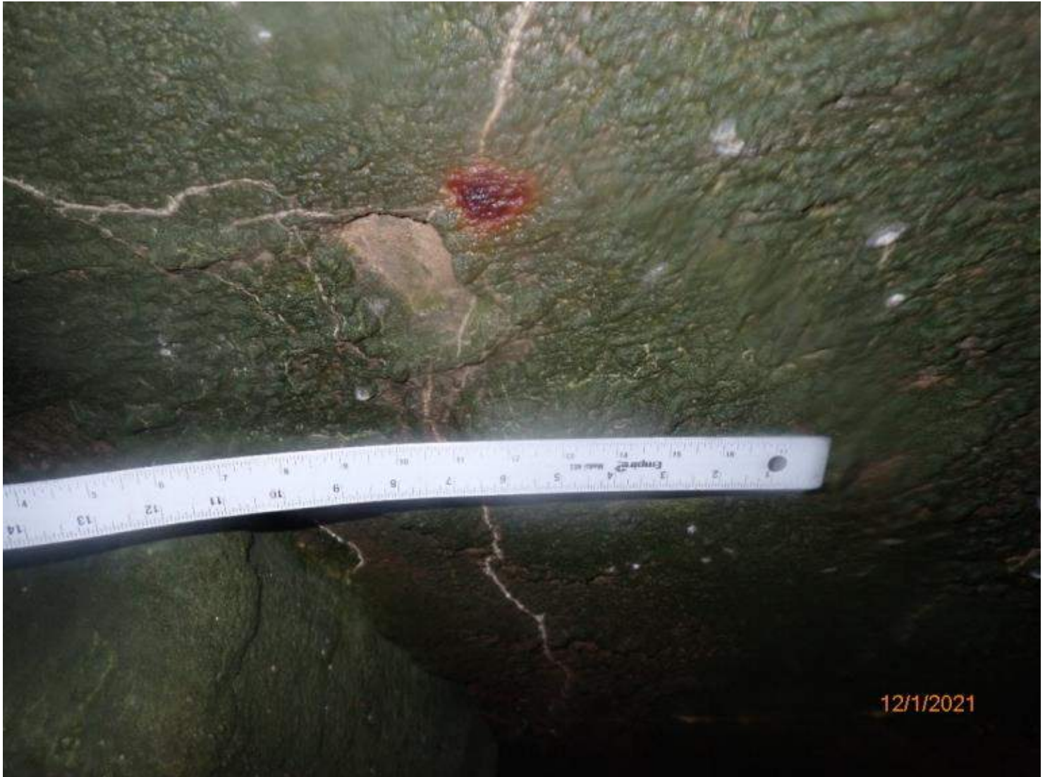
Photo 6 - Element 220 Re Conc Pile Cap/Ftg
