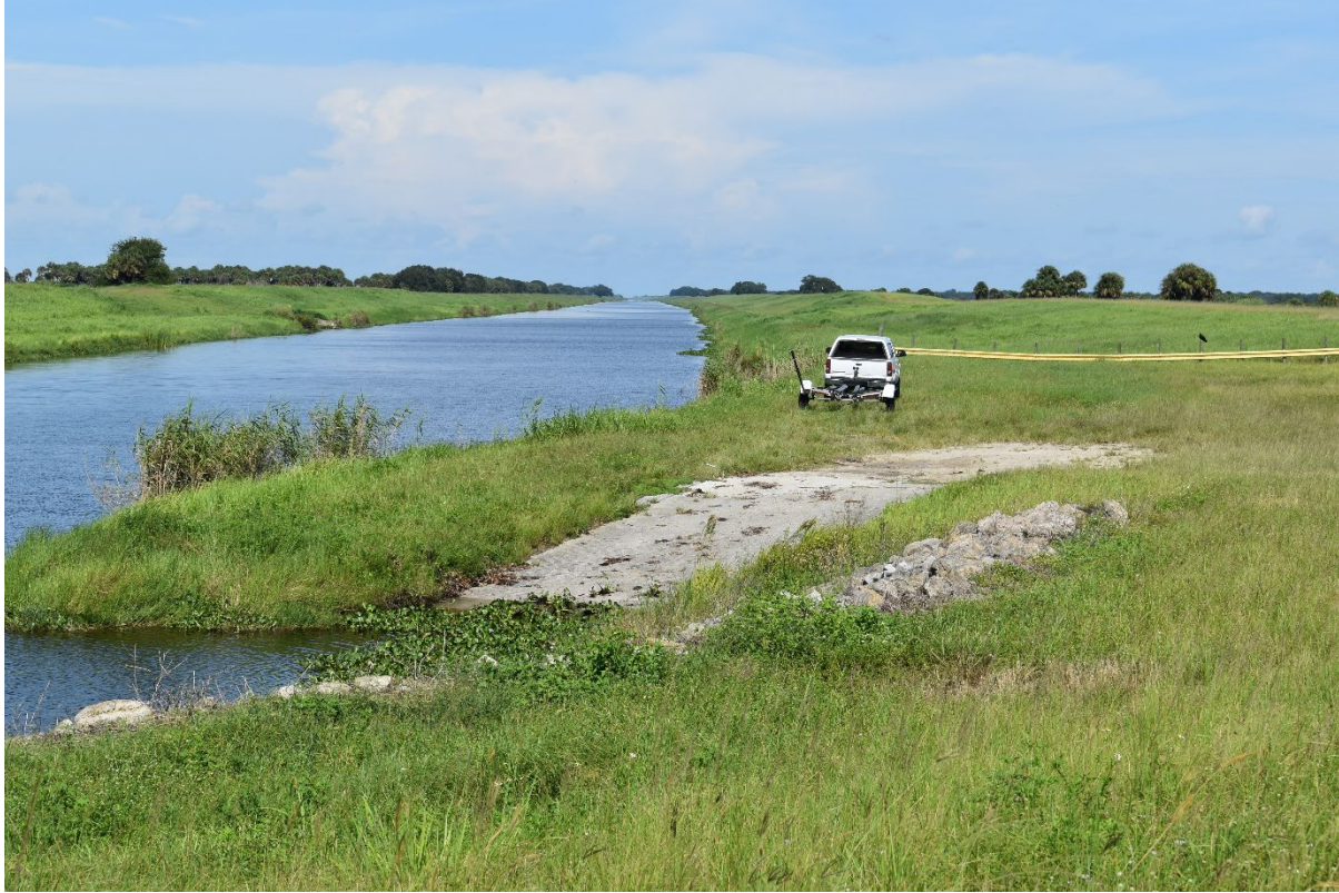
Photo 3: View facing north near boat ramp.
