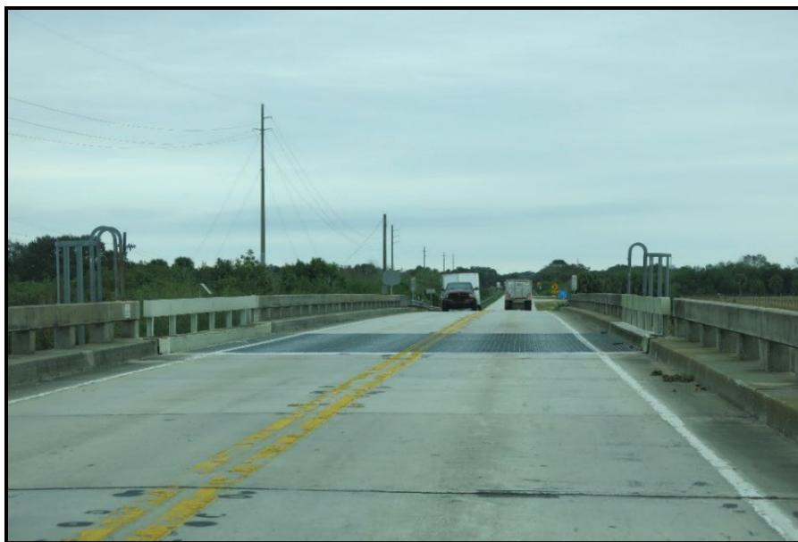
Photo 4-2 SR 70 over Kissimmee River Bridge, Bridge No. 910001 (8HG01236/8OB00336), looking east. Note the removable steel span.
