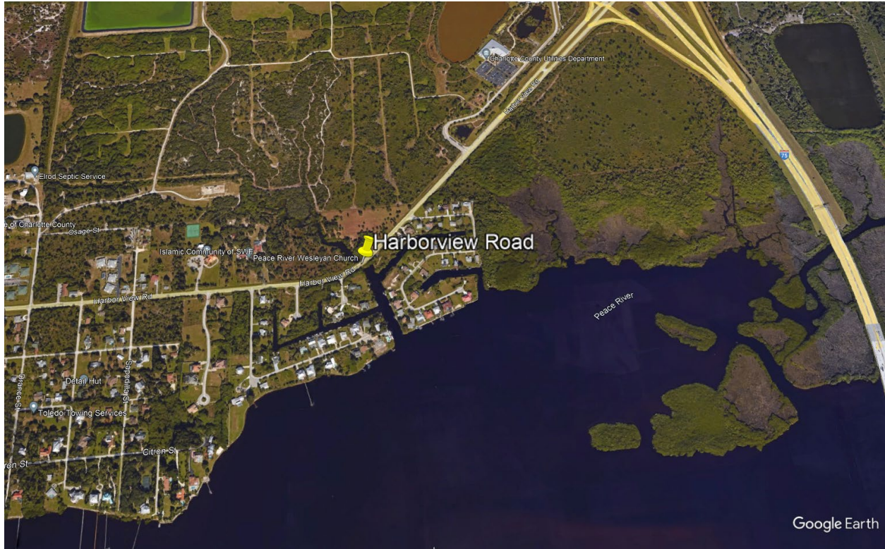
Figure 2. The project site at Harborview Road, showing the location of the box culvert bridge crossing an unnamed salt creek (©2024 Google).
