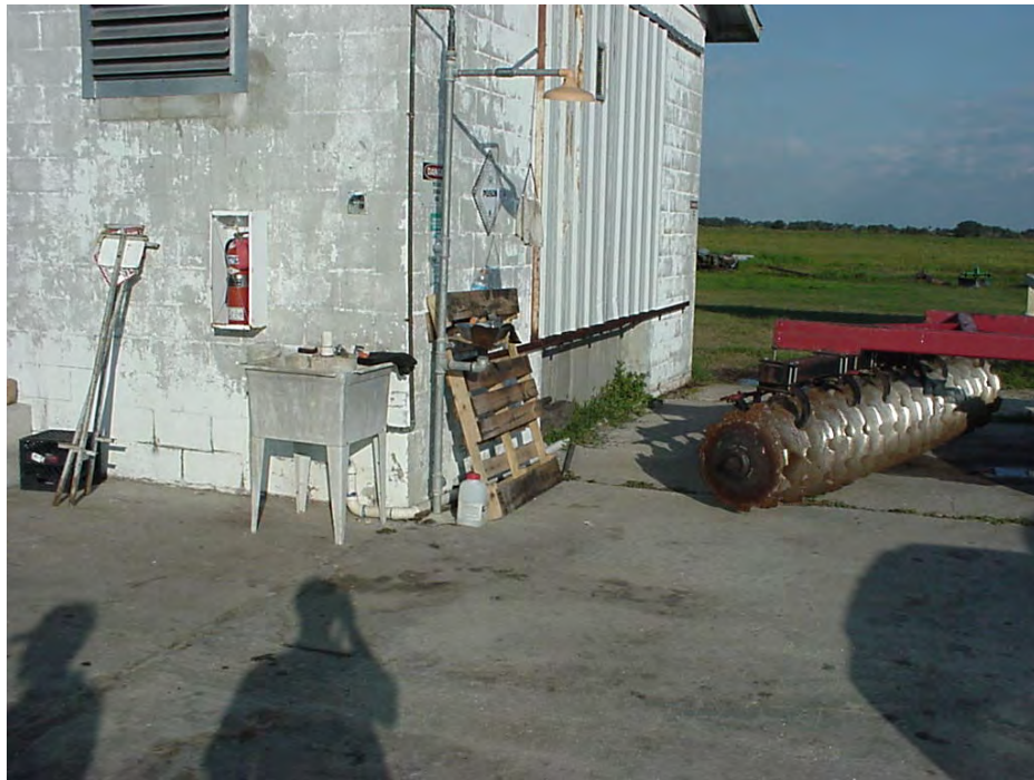
Photo 32. AOI 16: Herbicide-Pesticide Mixing and Storage Area. Note: Sink, drain line, and puddle of liquid at east edge of concrete slab.
