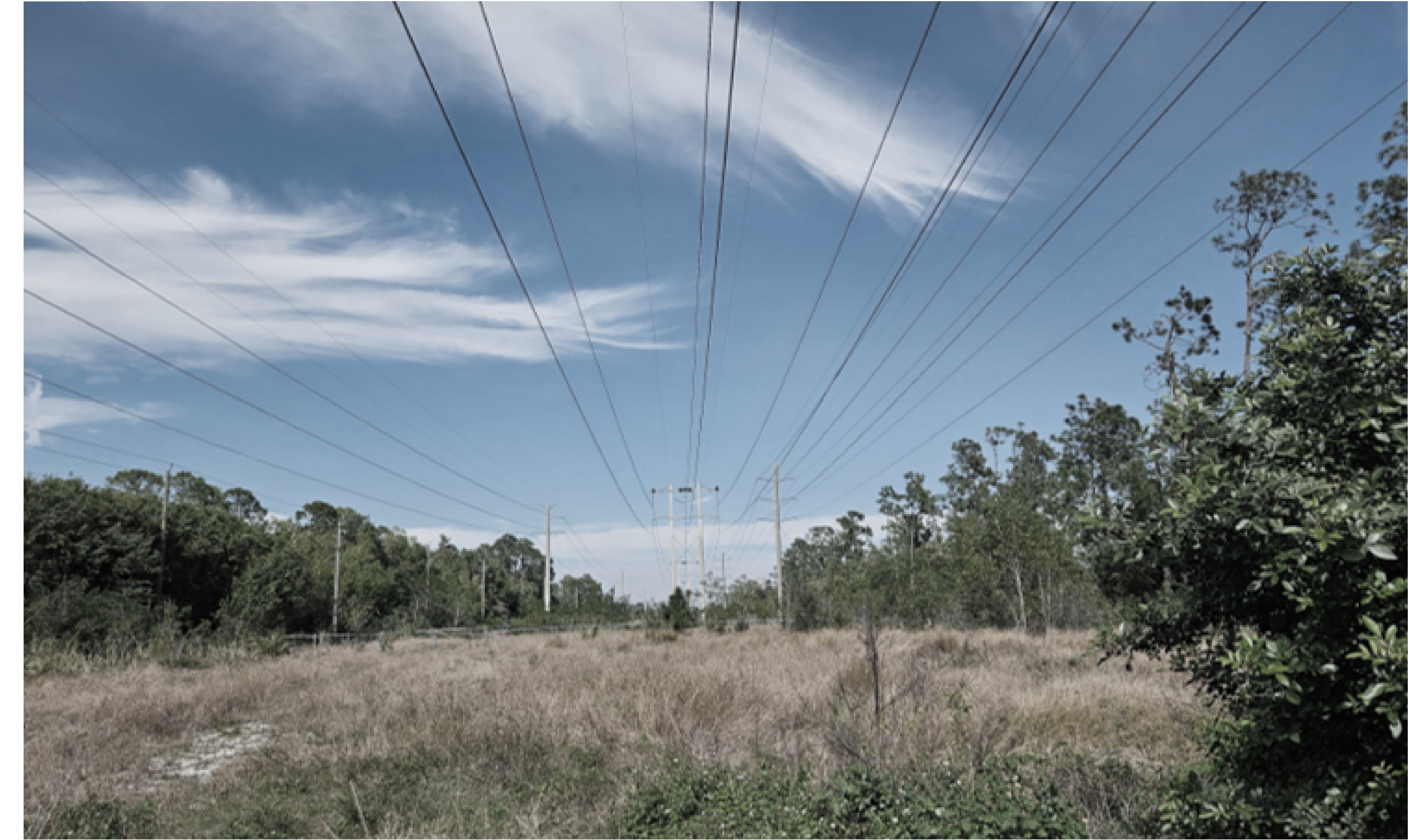
FPL EASEMENT (LOOKING NORTH)
