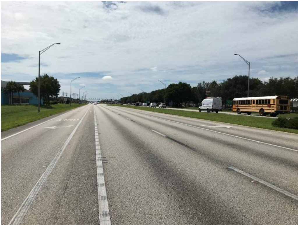
Looking west from the intersection along SR 78
