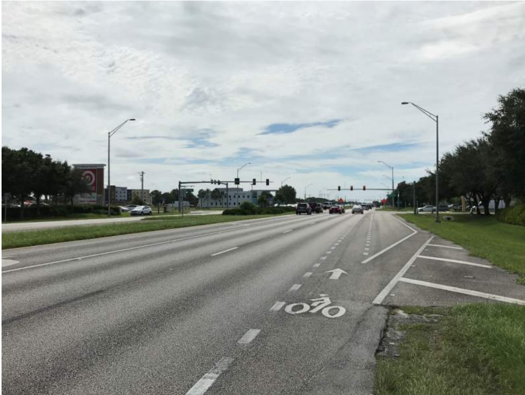
Looking west into the intersection along SR 78
