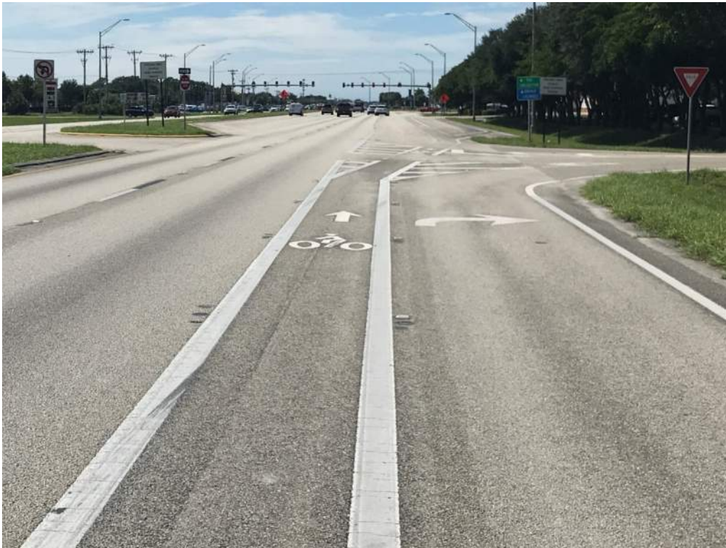
Looking west into the intersection along SR 78
