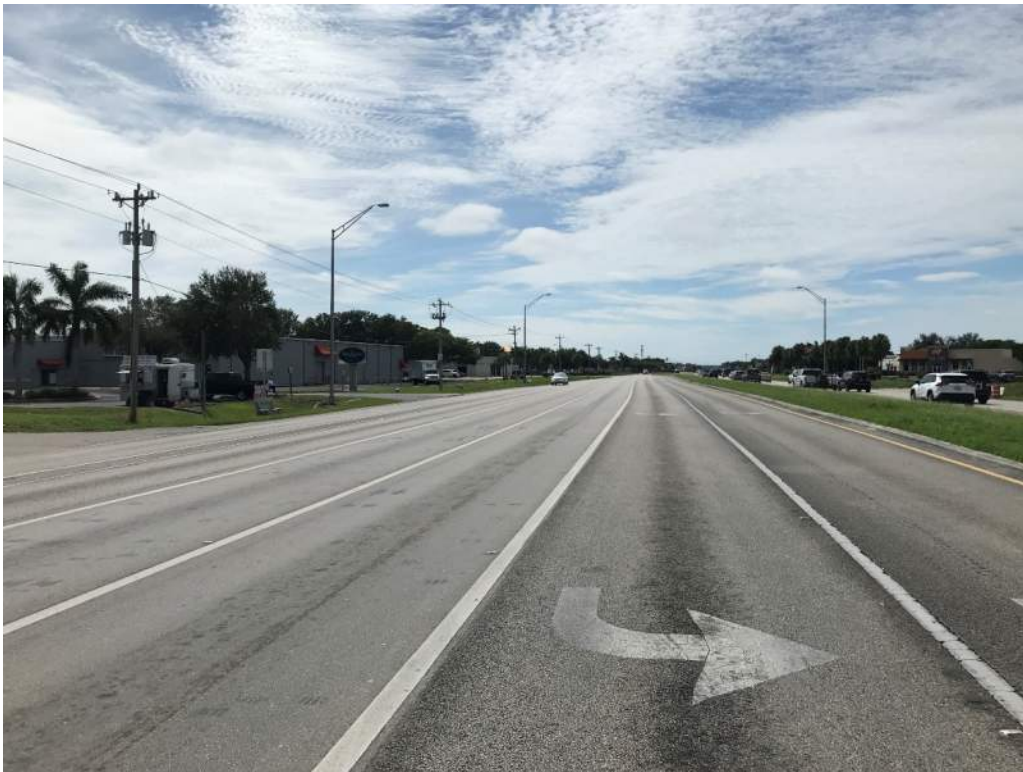
Looking west from the intersection along SR 78
